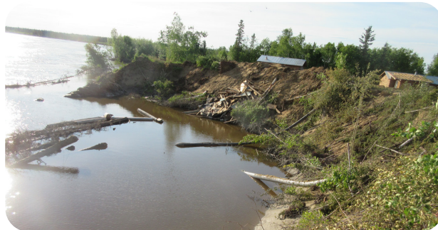
Riverbank erosion near Huslia.
