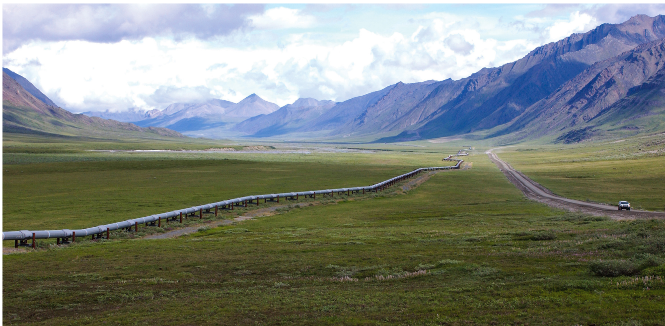
Alaska pipeline. ADF&G.
