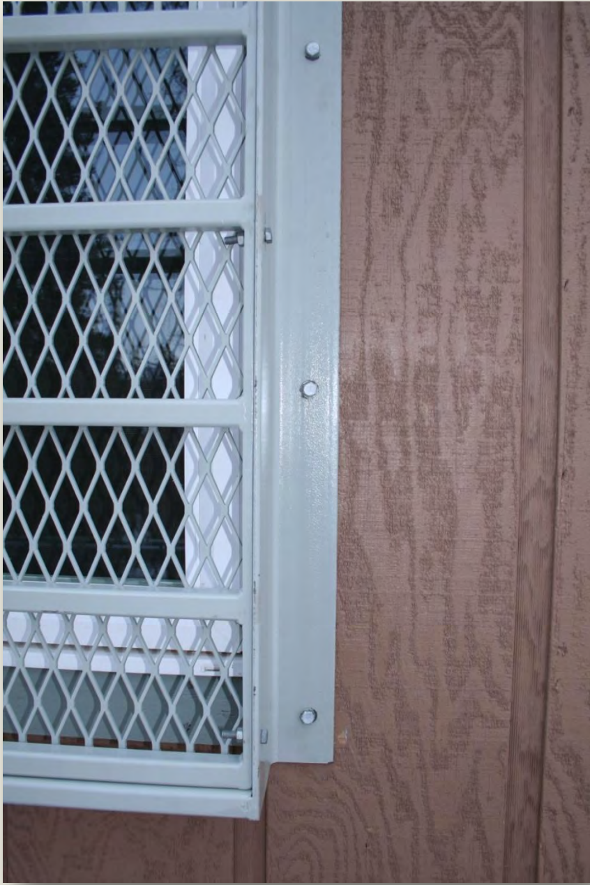
Photo by Sheldon Ewing, Weld Air
