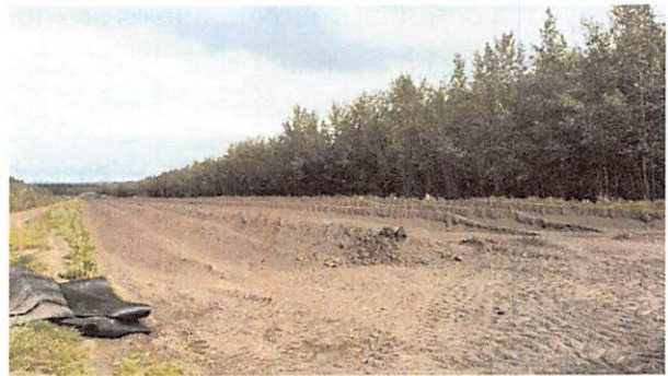
The BRAC group operates a landfarm at the former Campion AFS airstrip, approximately 6 miles east of Galena. This photo shows windrows of petroleum-contaminated soil that were undergoing treatment in the landfarm. Once soil concentrations meet the most stringent 18 AAC 75 Table B1 and B2 cleanup levels, the Solid Waste and Contaminated Sites Program coordinate with the City of Galena to use the clean soil as cover material in the city landfill. The landfarm operates from approximately June through September each year.
