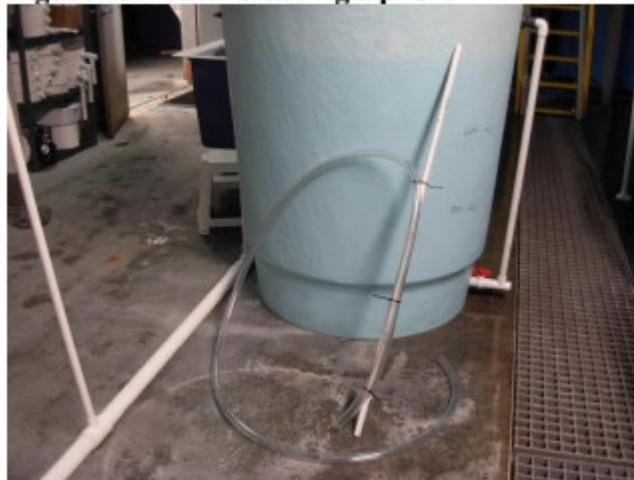
Figure 23. Tank cleaning siphon.
