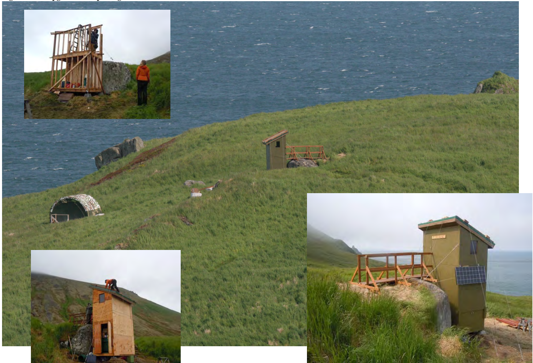
Figure 9. Campground composting toilet / outhouse construction.
