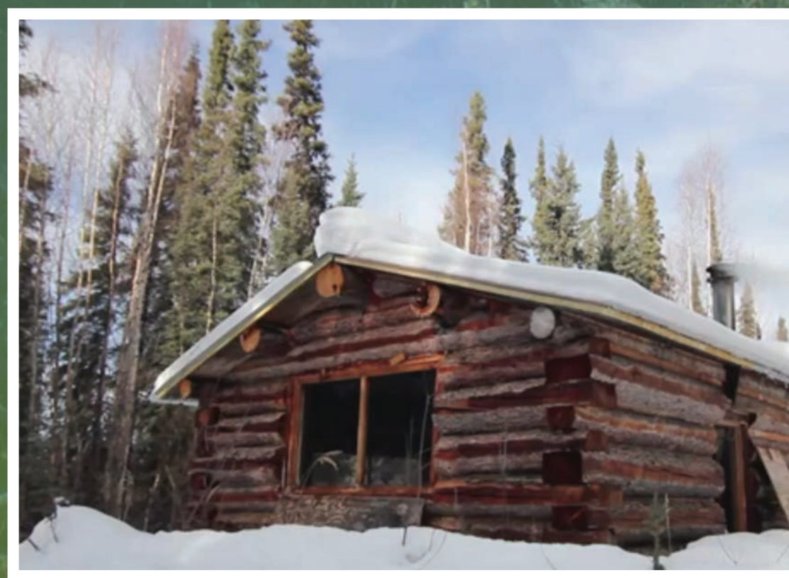
Nugget Creek Public-use Cabin at mile 12 of the Mastodon Trail
