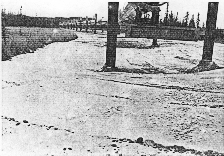
View of an excavated Designated Big Game Crossing, looking along the pipe.
