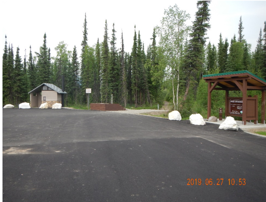
Figure 9 – Picture of Completed Orientation Kiosk, ATV/Snow-Machine Ramp, & CXT Concrete Vaulted Toilet at Upper Chena Dome Trailhead
