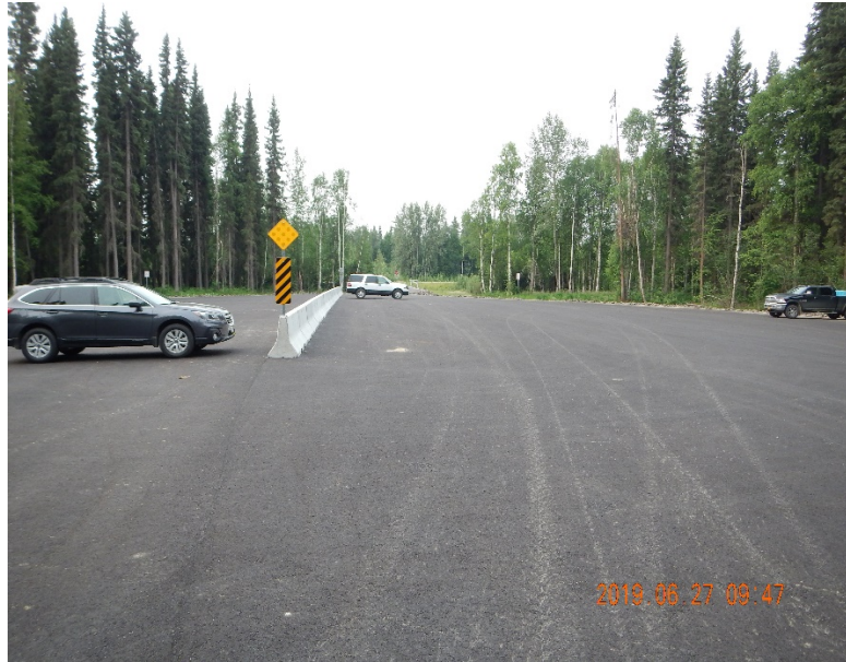
Figure 3 – Picture of Completed Parking Area at Compeau Trailhead
