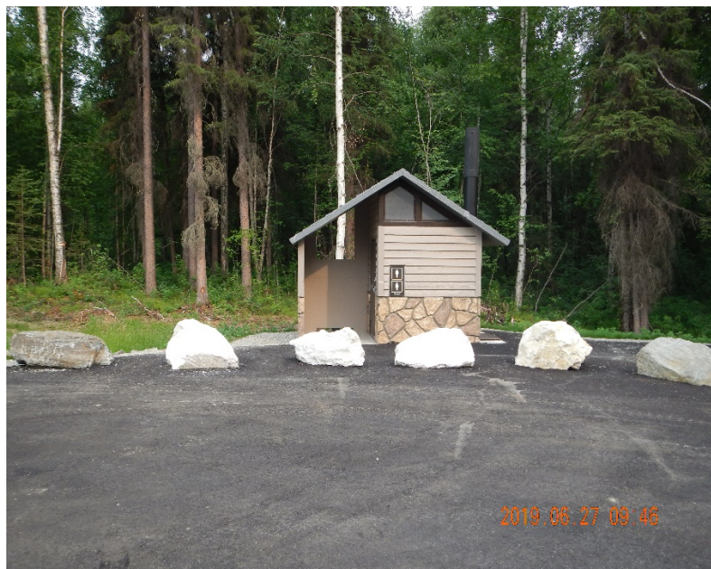
Figure 2 – Picture of Completed CXT Concrete Vaulted Toilet at Compeau Trailhead
