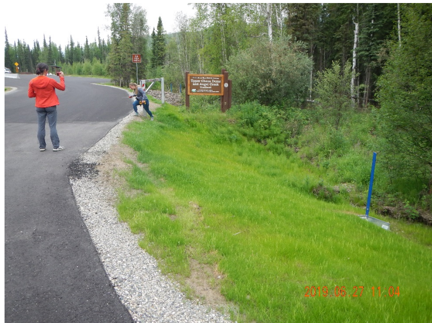
Figure 10 – Picture of Completed Entrance Sign at Upper Chena Dome Trailhead
