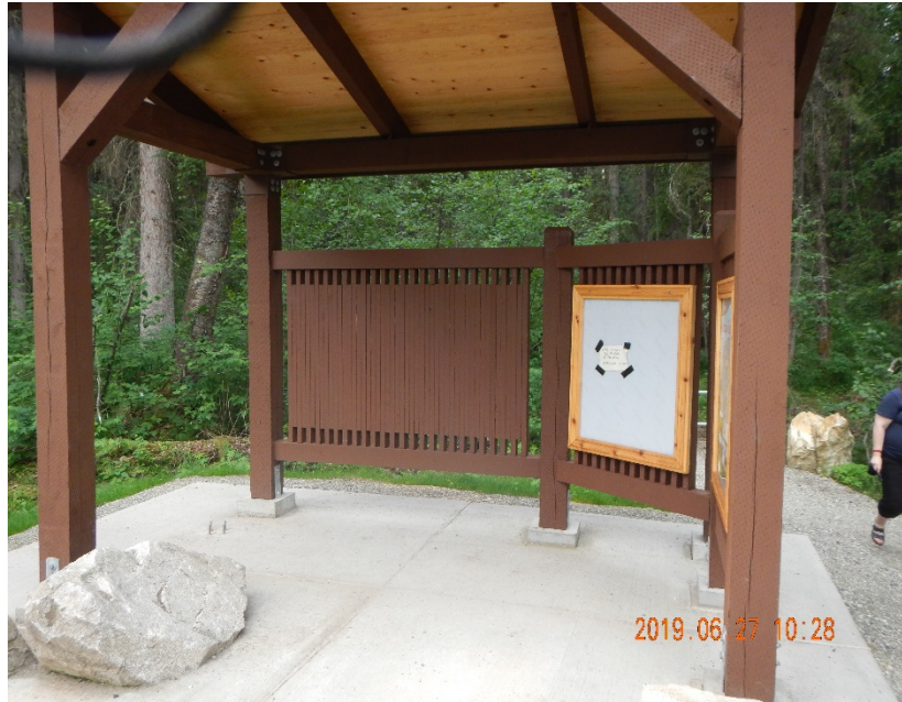
Figure 7 – Picture of Completed Orientation Kiosk at Mastodon Trailhead
