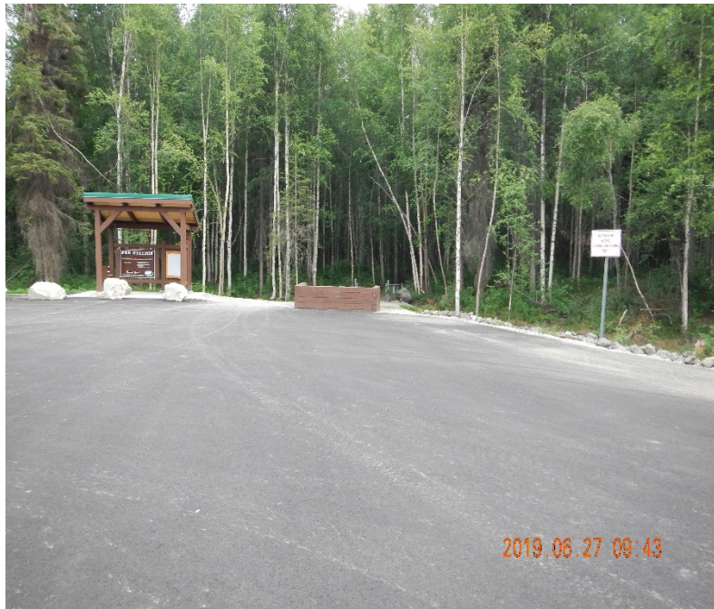
Figure 1 – Picture of Completed Orientation Kiosk & ATV/Snow-Machine Ramp at Compeau TH
