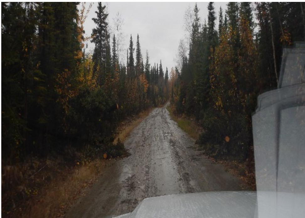
Figure 2.—September 2019 survey trip. Road conditions did not allow the group to complete the survey.
