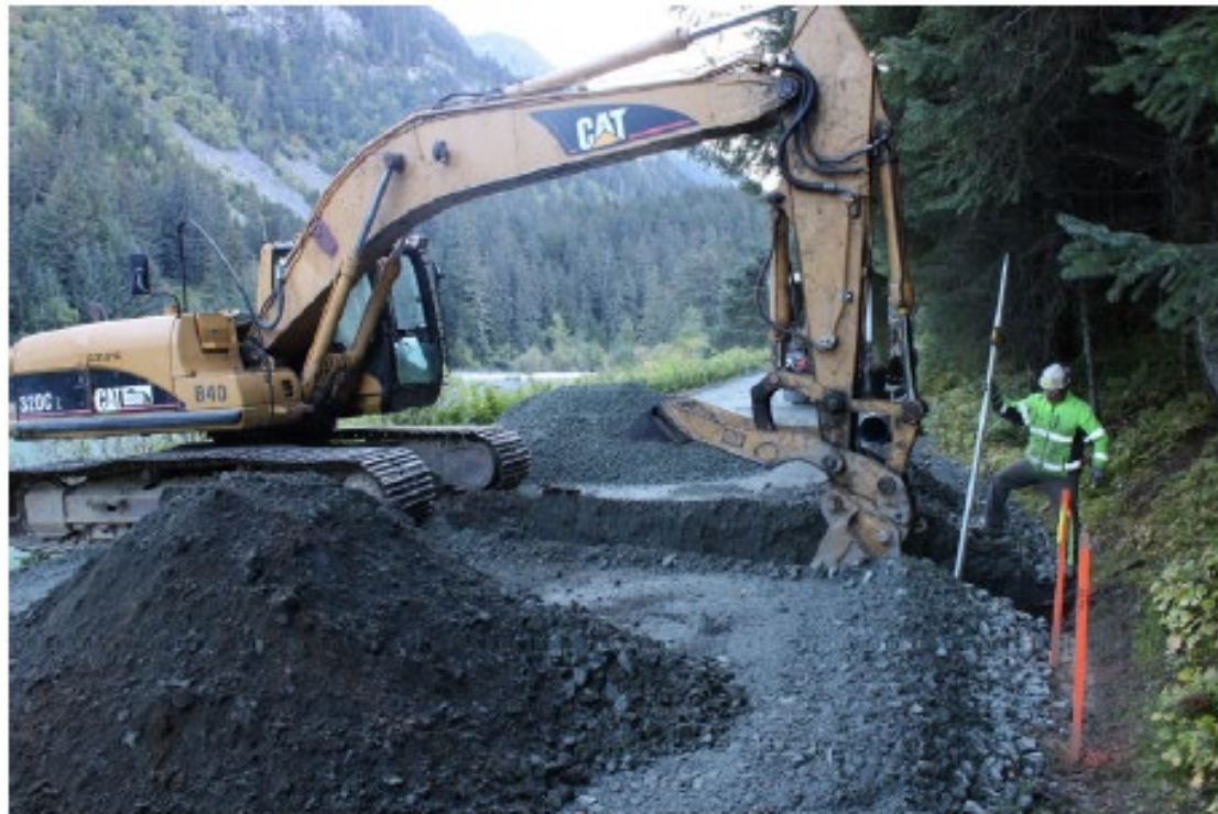
Figure 5.—Excavating material fill for culvert installation.
