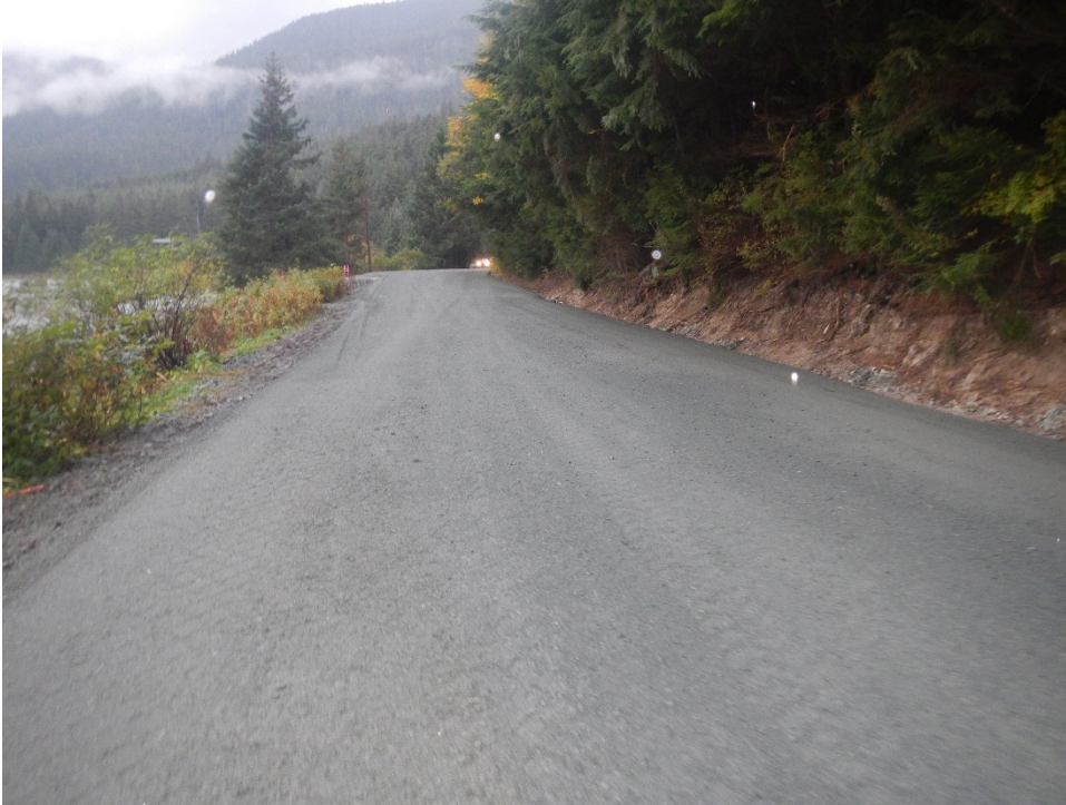
Figure 6.—During construction smooth aggregate surface roadway and pullout with ditches.
