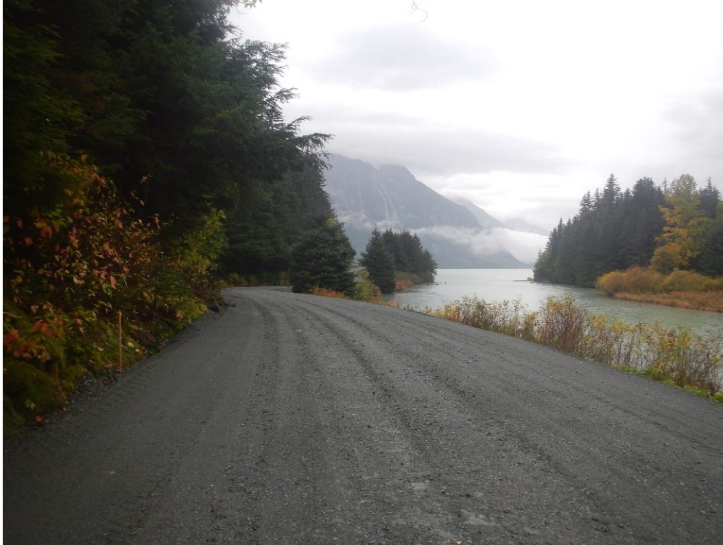
Figure 2.—During construction road surface smoothing.
