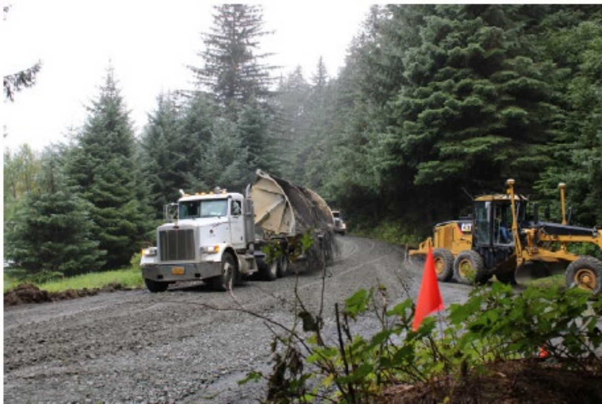
Figure 1.–Placing gravel fill on the roadbed.
