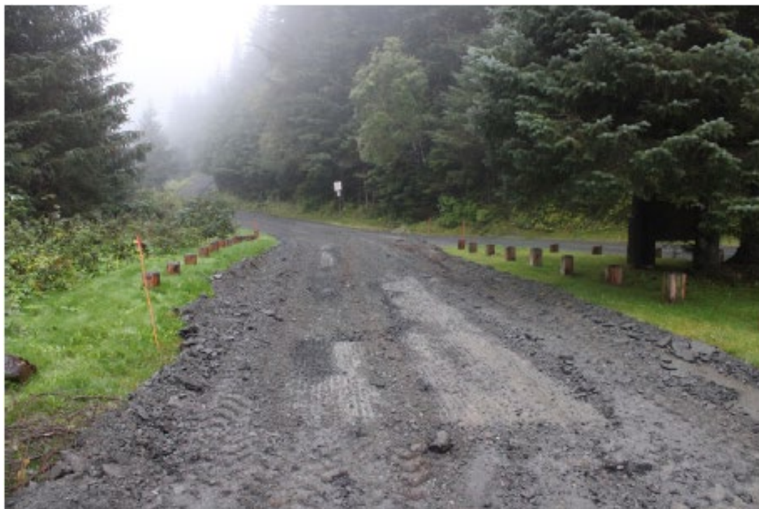
Figure 3.—Milled roadbed near the boat launch parking lot.
