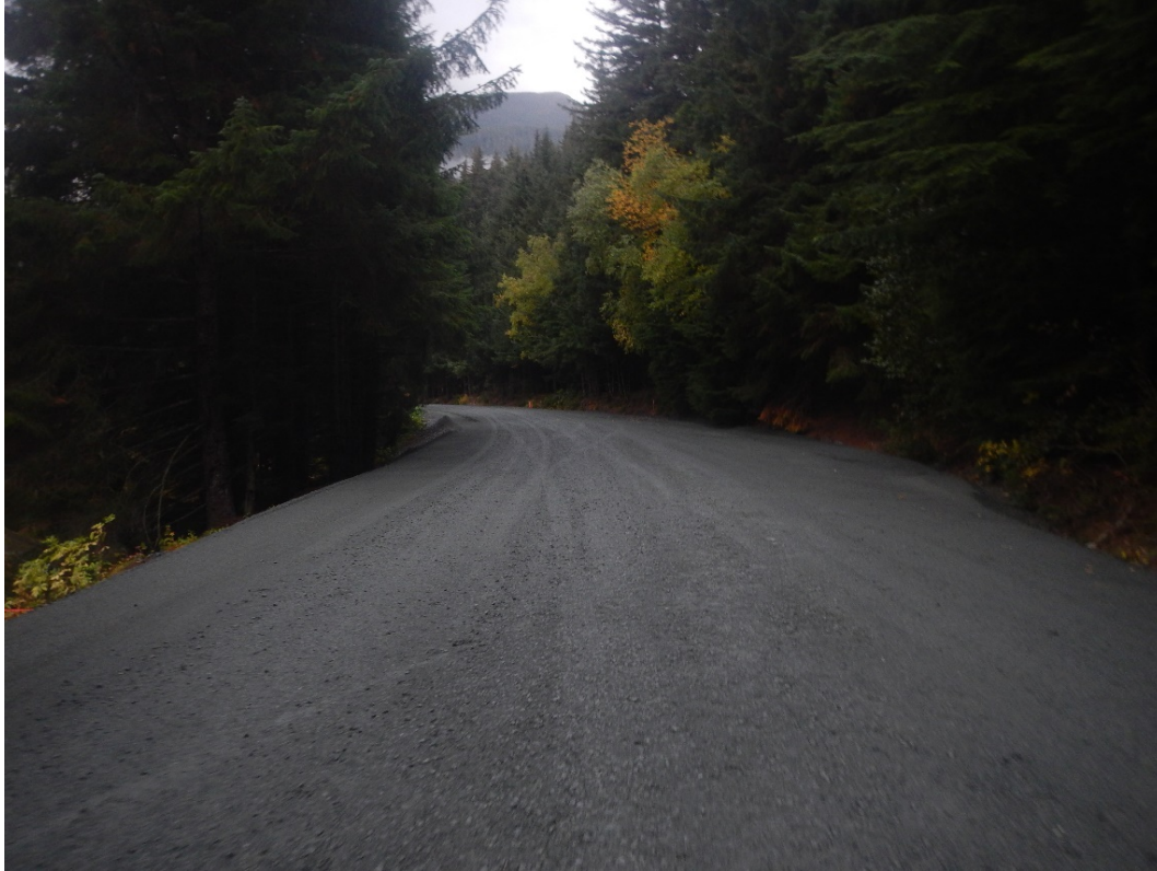
Figure 4.—During construction slope roadway and pullout with ditches.
