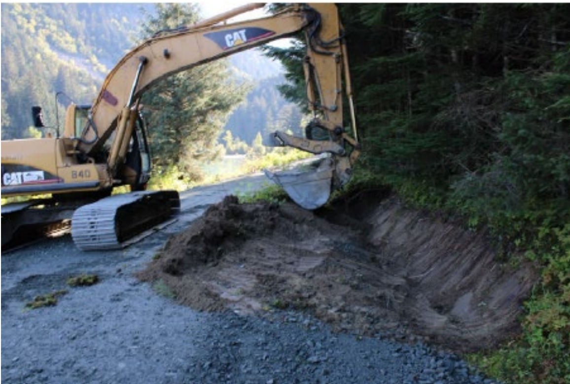
Figure 7.—Excavating drainage ditching along the road leading to a culvert.
