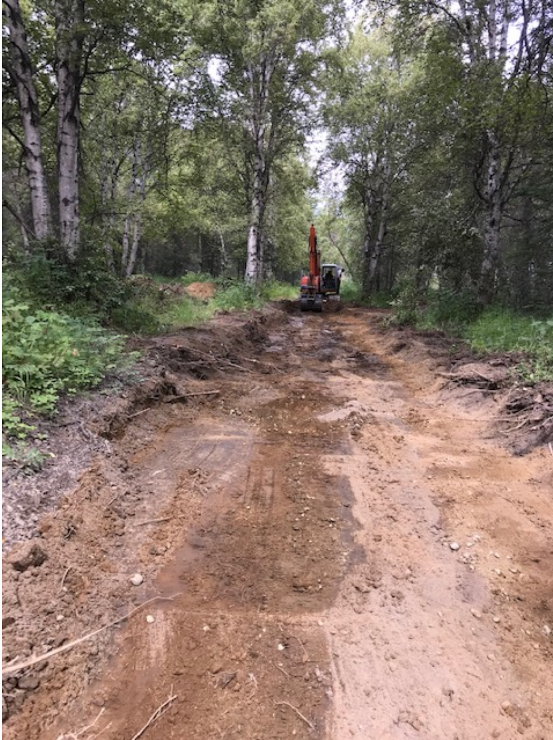
Figure 1.—Contractor filled in and leveled out rutted areas and improved drainage at historically wet and soft locations on the DOF Wendt Road access in the Matanuska Valley Moose Range (MVMR).
