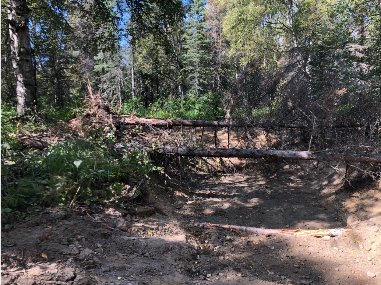
Figure 2.—Drain sumps were installed as part of DOF road improvements in the MVMR. Some were protected by trees laid over the top to prevent damage from ATV traffic. Buried logs serve as water bars to slow runoff and allow water to percolate into soil.
