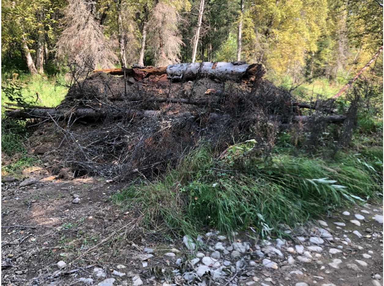
Figure 3.—Soil and log berms along MVMR road improvements redirect traffic from social trails to the improved road. Dirt piled over logs is intended to deter users from cutting logs in these piles.
