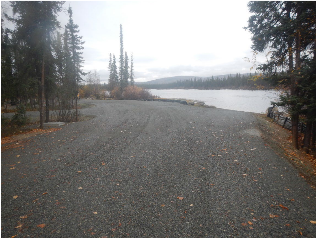
Figure 1.– Completed boat launch and roadway with additional parking
