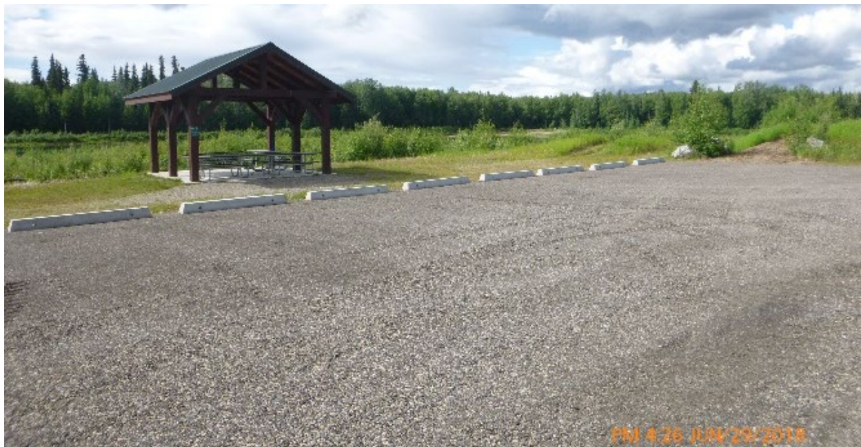
Figure 4.—Completed day use parking area at Olnes Pond.
