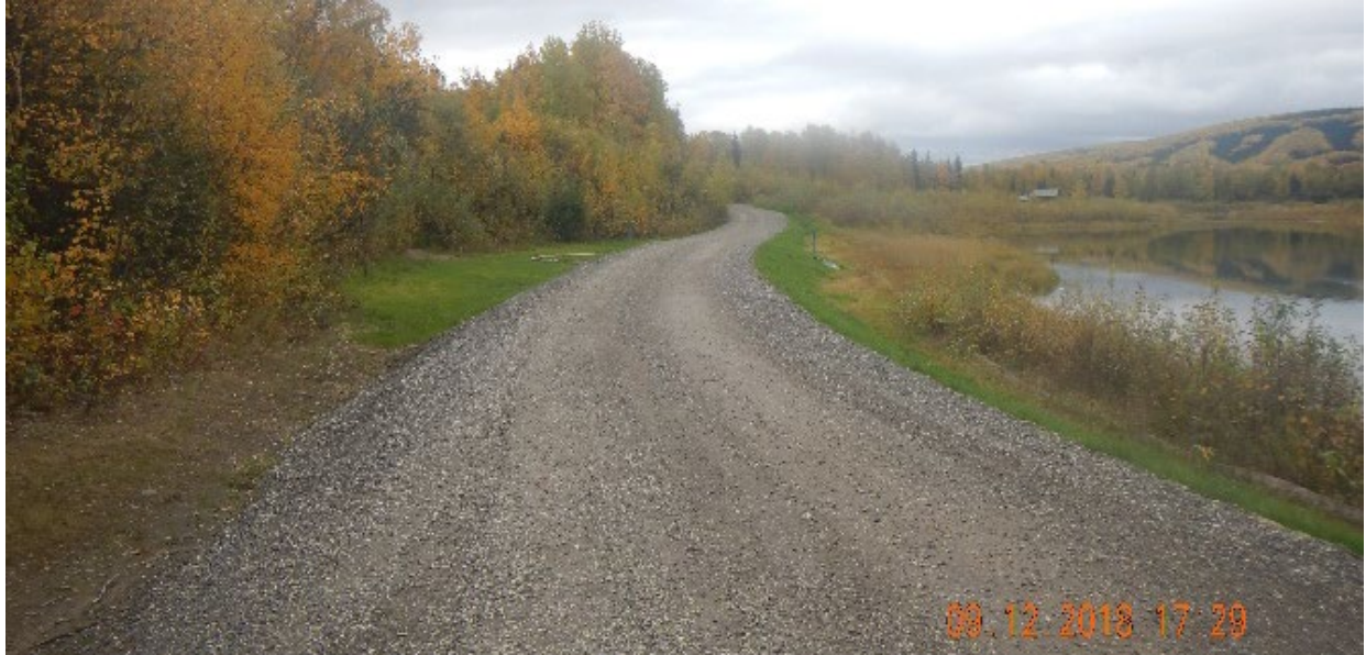
Figure 3.—Completed roadway at Olnes Pond.
