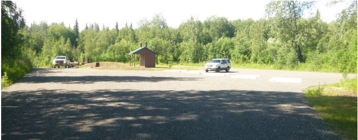
Figure 1.—Completed boat launch parking area at Whitefish campground.
