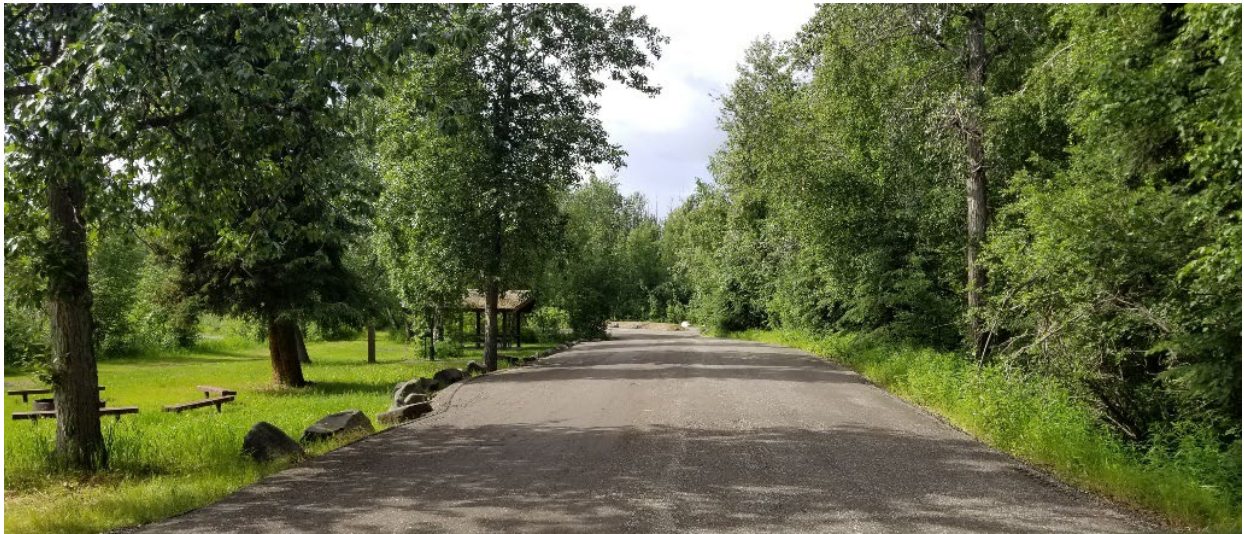
Figure 2.—Completed roadway at Whitefish campground.
