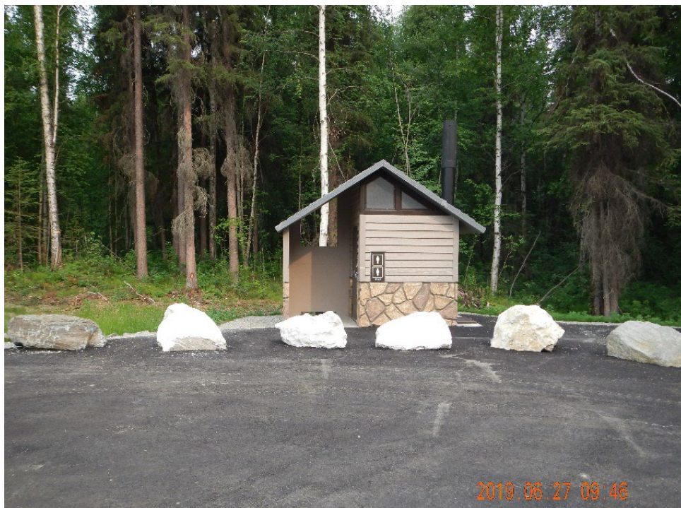
Figure 2.–Picture of completed CXT concrete vaulted toilet at Compeau Trailhead.
