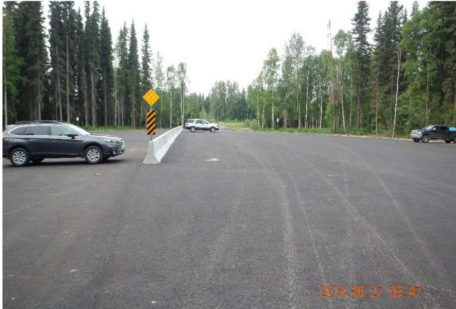
Figure 3.—Picture of completed parking area at Compeau Trailhead.
