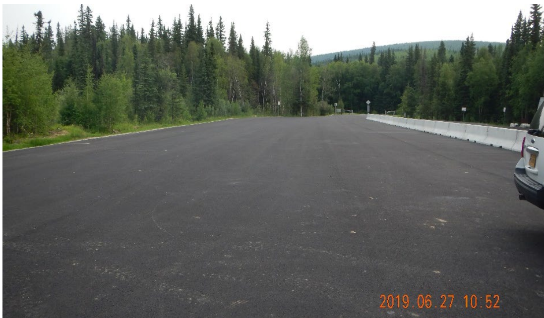
Figure 8.—Picture of completed parking area at Upper Chena Dome Trailhead.
