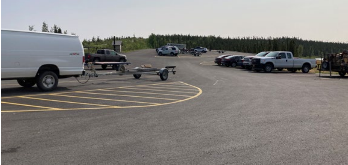
Figure 2.—Freshly paved and striped parking area at Lake Louise Recreation site, 2021.
