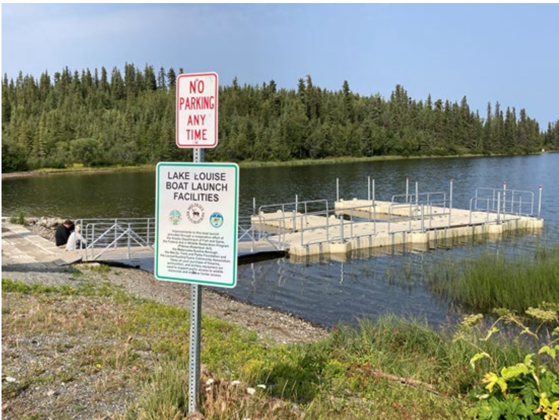
Figure 1.–New accessible floating dock at Lake Louise Recreation site, 2021.
