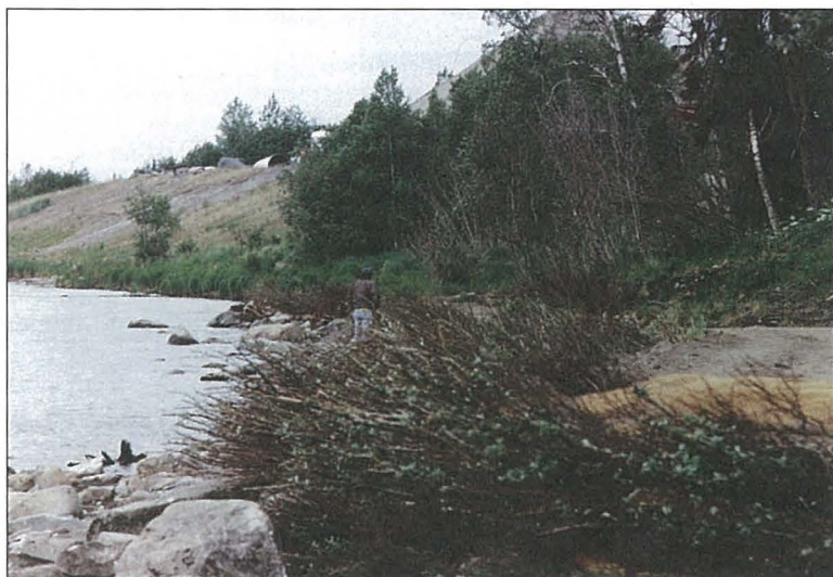
Vegetated cribbing three weeks after installation
