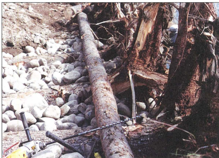
Root wad, rock layer with header log pinning, Pioneer Lodge
