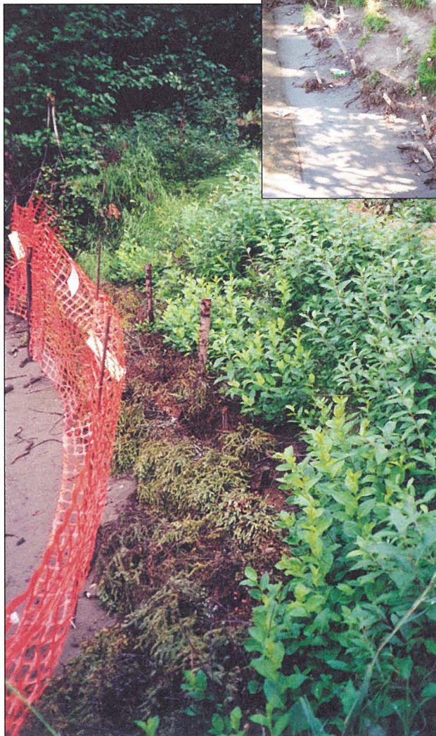
Little Susitna Recreation Site, cabled spruce trees and brush layering, three months after installation.
