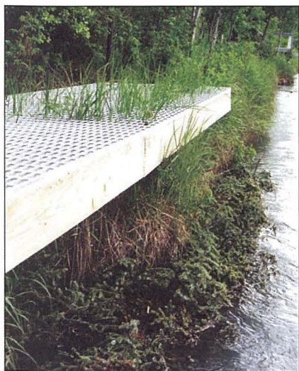
Gratewalk and cabled spruce trees, Kenai River
