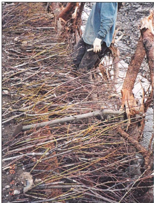
Brush layering installation prior to trimming, Centennial Park, Kenai River
