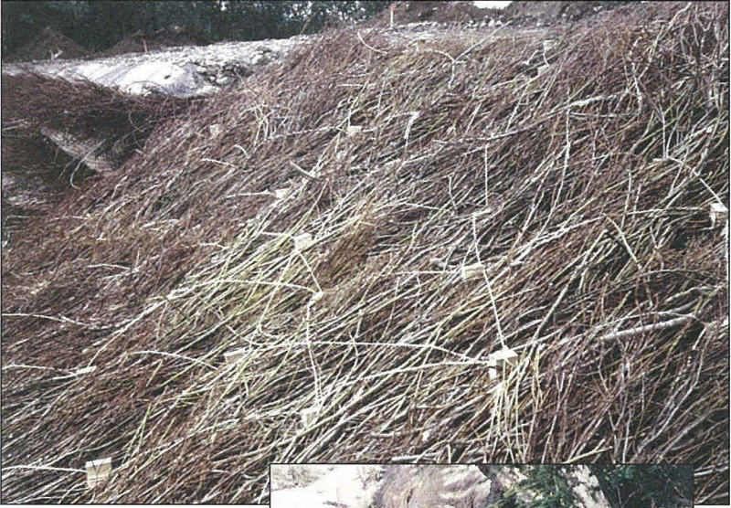
Brush mat - note the criss-cross pattern of the jute used to anchor the mat to the bank.
