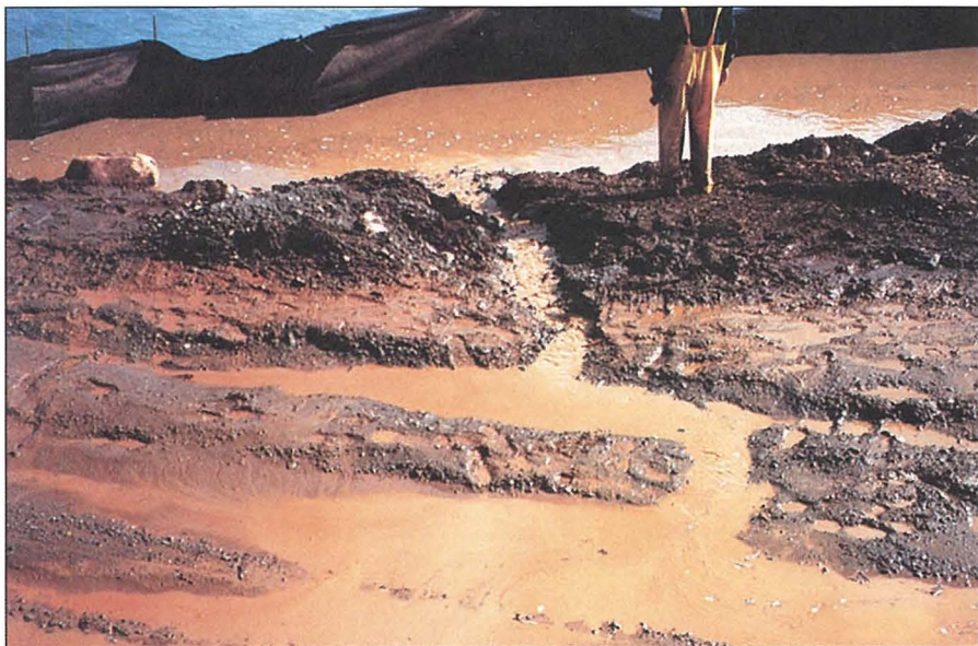
Centennial Park erosion control, Soldotna, Alaska
