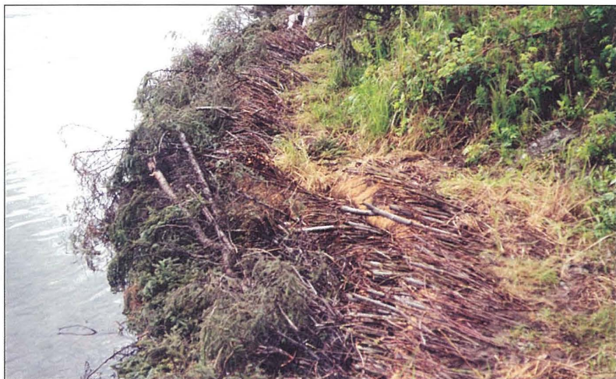
Cabled spruce trees and brush layering immediately after installation, Ciechanski Recreation Site, Kenai River
