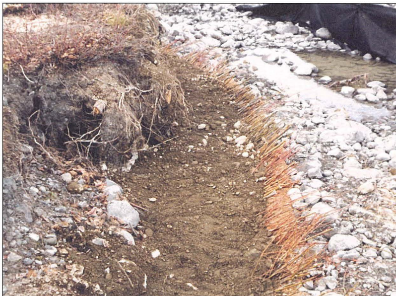
Live siltation during construction
