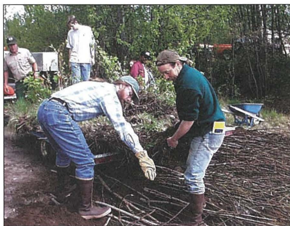
Placement of vegetative mat after harvesting
