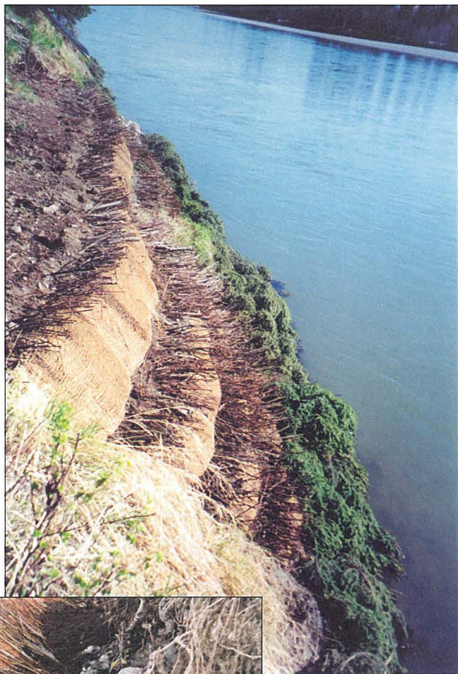
Brush layering and cabled spruce trees, Kenai River
