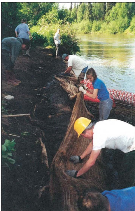
Installation of brush layering, Little Susitna River, Youth Restoration Corp.
