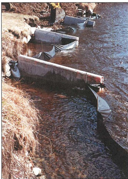
Jersey barriers and silt fence isolating the work area, Willow Creek
