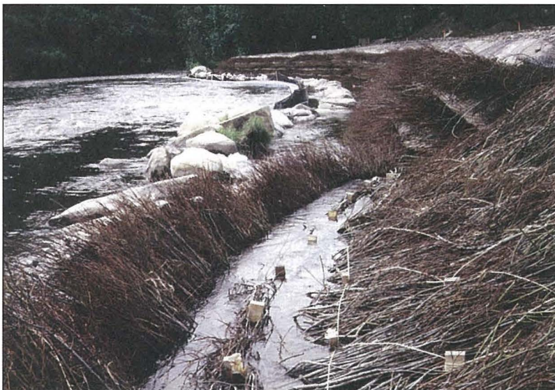
Brush mat and live siltation constructed at Deep Creek in 1994. Note bundle was used to provide a transition between the two techniques.
