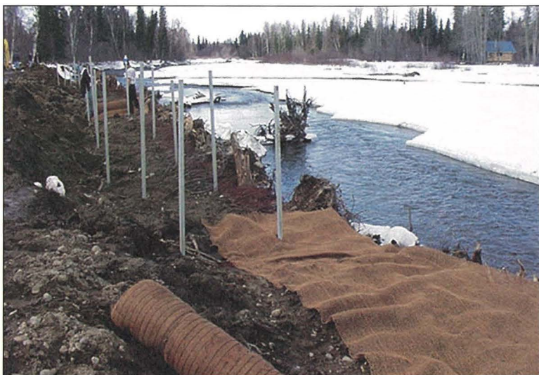
Installation of subsequent brush layering/soil wraps above root wads; the picture shows walkway supports installed. Pioneer Lodge, Willow Creek April 10-11, 2001
