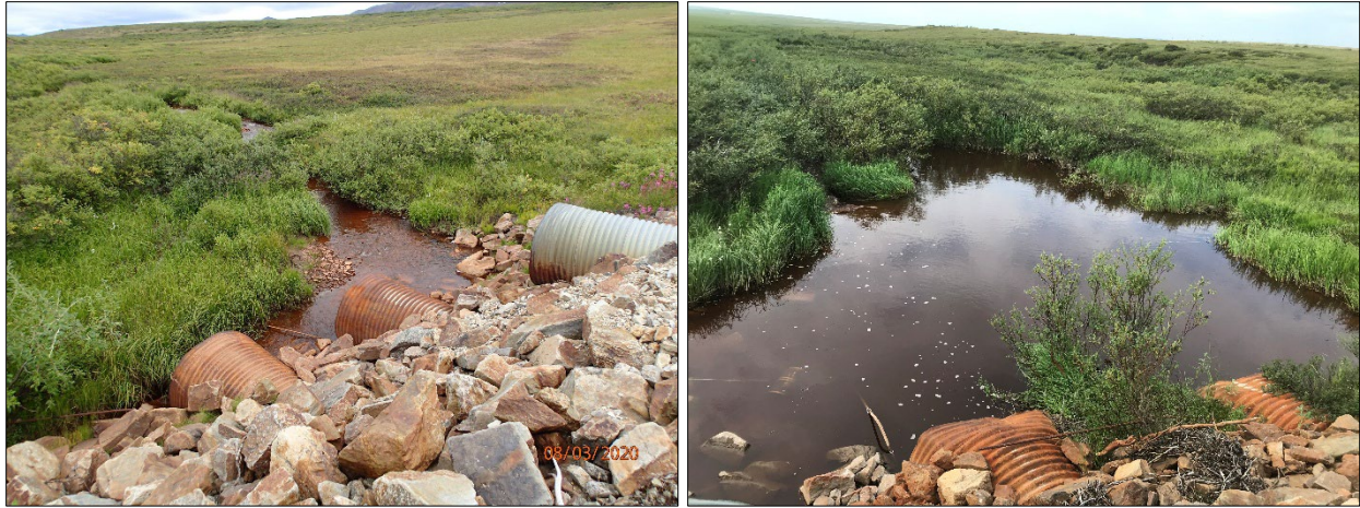
Figure 9.—Evangiknuk Creek upstream of the road (left) and downstream of the road (right).
