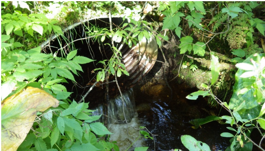
Figure 2.—Perch at culvert outlet.
