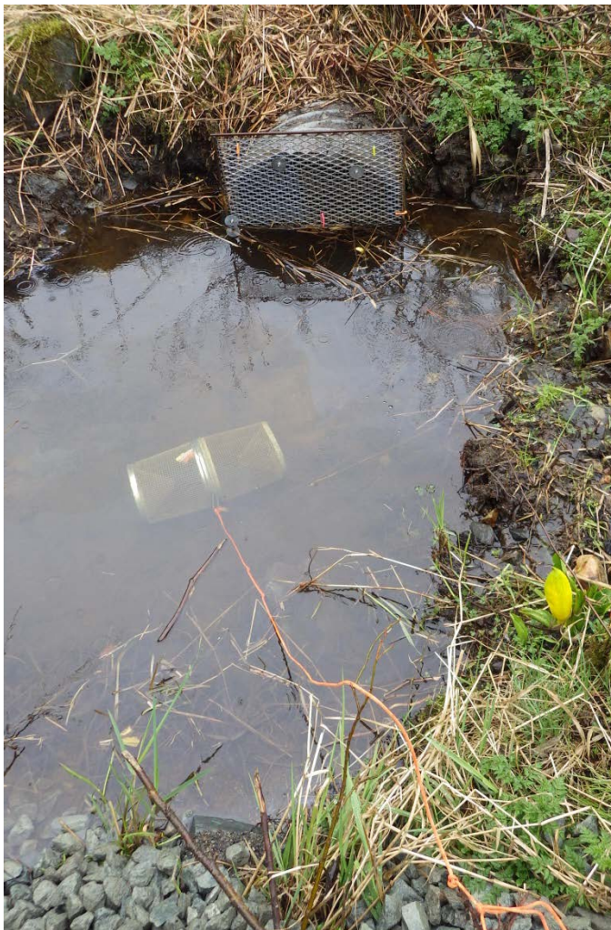
Figure 1.–Culvert with fish exclusion screen.
