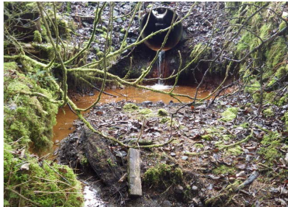
Figure 4.–CMP outlet under LDS parking lot.
