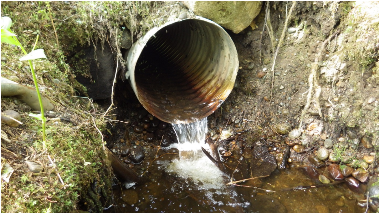
Figure 3.–Perched culvert at Black Bear Road.
