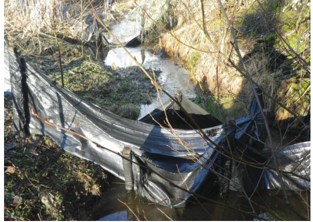
Figure 2.—Three sediment screens in stream that fish can pass.
