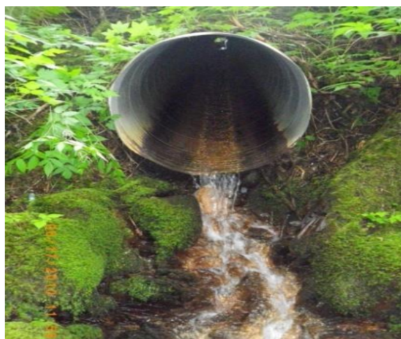
Figure 1.—Outlet of perched culvert.
