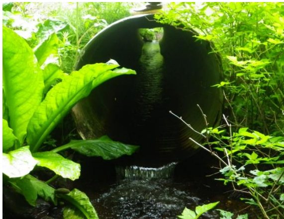
Figure 1.–Perched culvert conveying flows beneath Lena Loop road.
