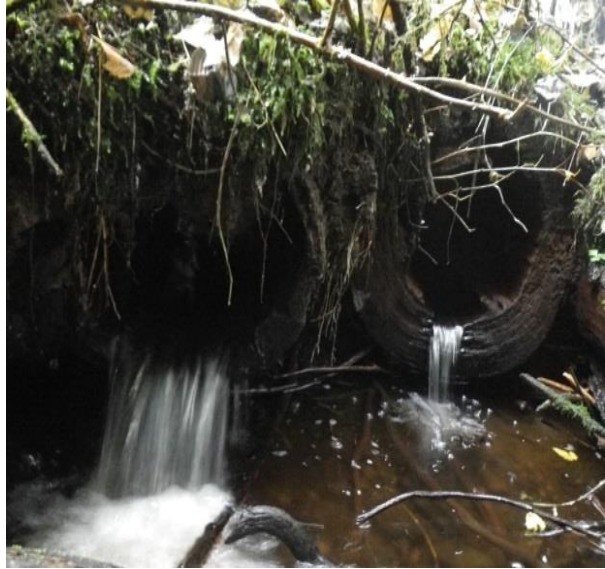
Figure 3.–Wood culverts under Switzer Trail.
