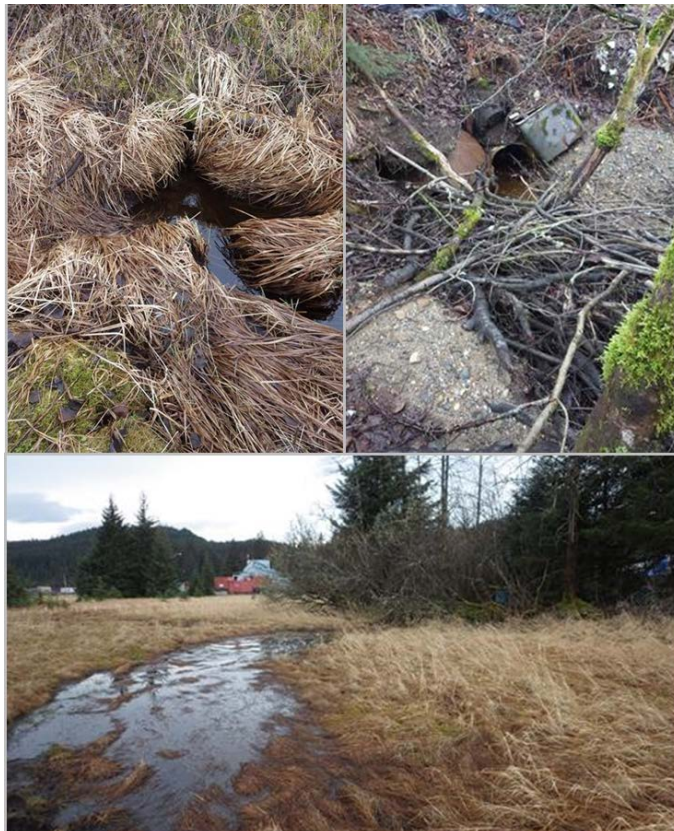
Figure 1.–Culvert inlet (left), outlet (right) and ponded wetland area (bottom).
