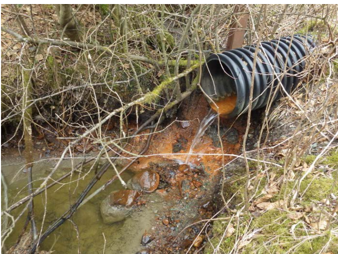
Figure 1.–Barrier culvert at waypoint 1.
