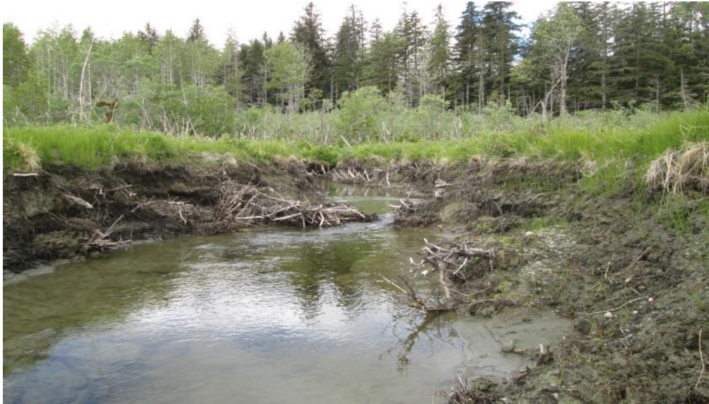
Figure 3.—The stream is cutting back through the sediment layer that had been deposited here when beavers were active in area.
