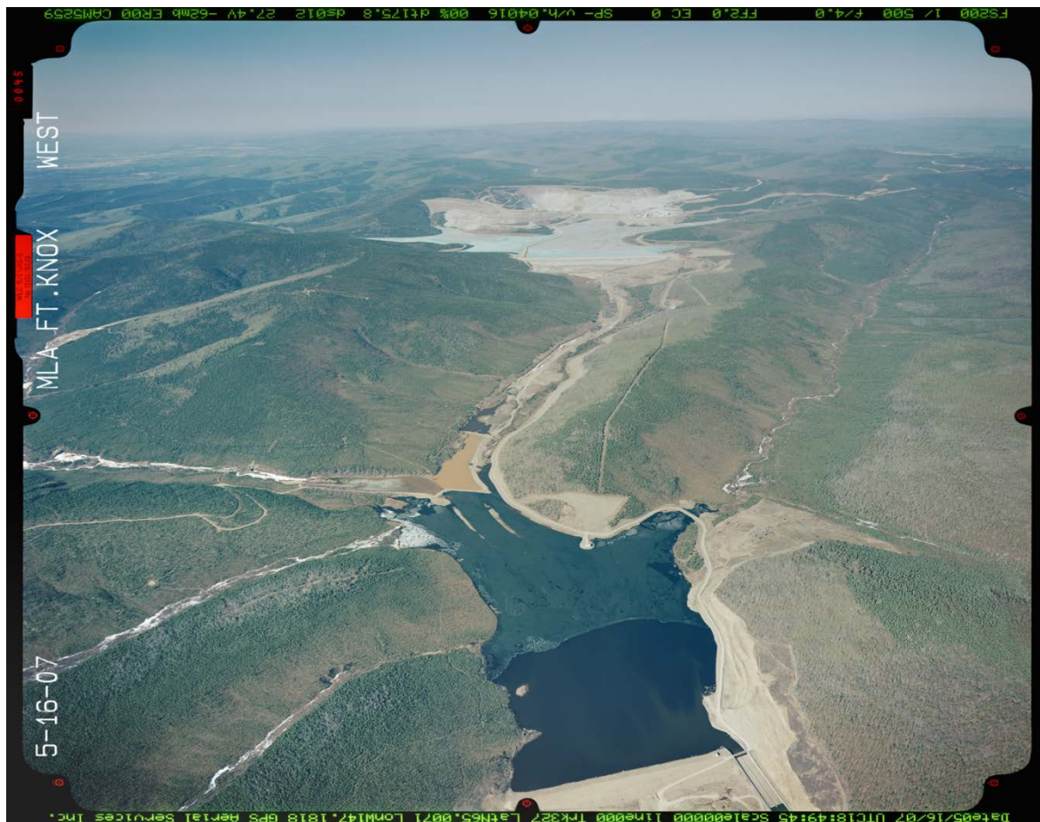
Figure 1. Aerial photograph of the Fort Knox Gold Mine WSR, tailings facility and pit – water supply reservoir in lower part of photo and the tailings dam and impoundment in the upper Fish Creek valley, photograph provided by FGMI.
