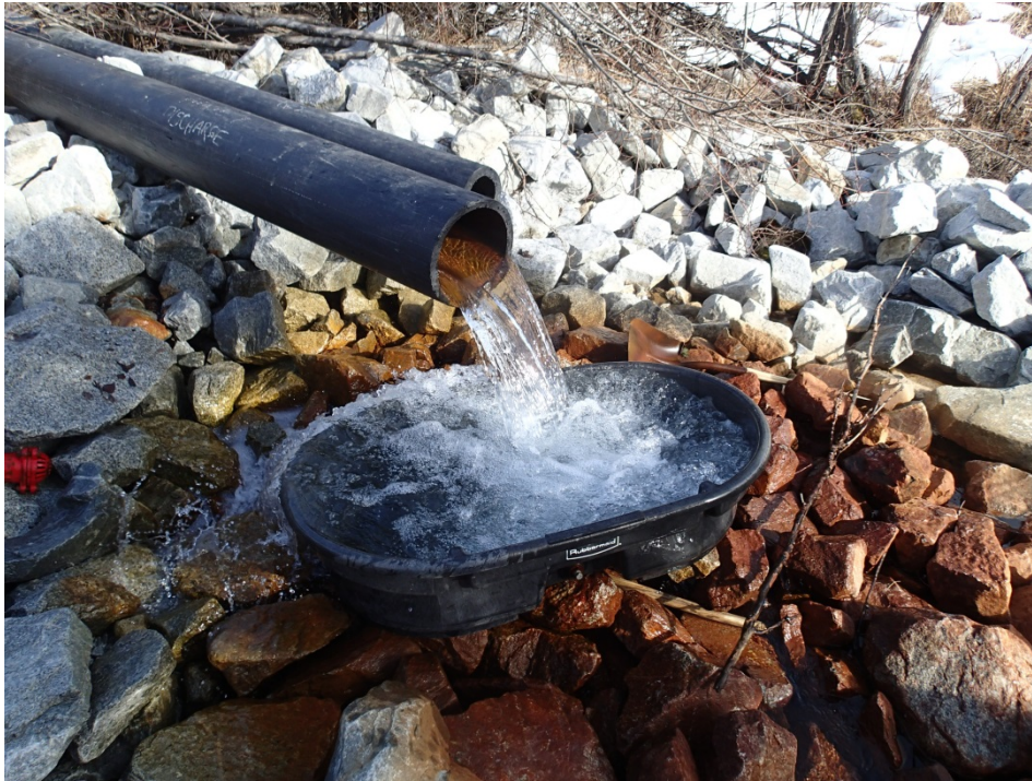
Figure 9. Discharge point for non-contact water from dewatering wells around the Fort Knox open pit.
