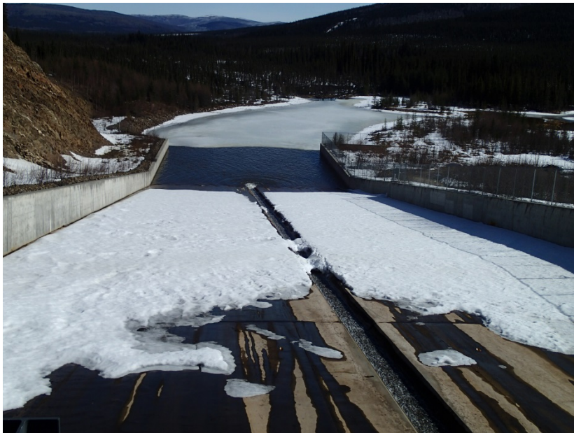
Figure 3. Spillway in water supply reservoir in late April, 2017.
