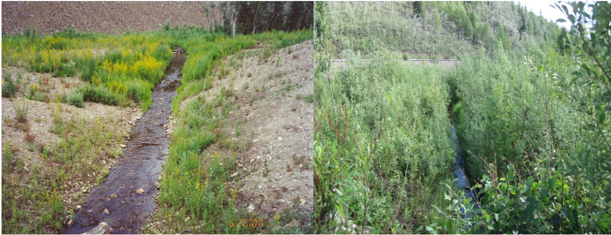
Figure 2. Pond F outlet channel in 2000 (left photo) and in 2010 (right photo).
