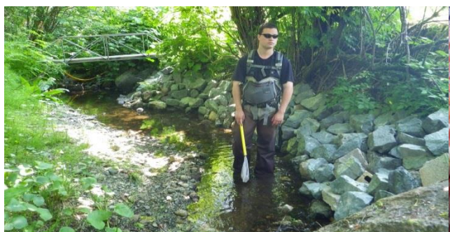
Figure 3.–Residential rock revetment to prevent stream bank erosion.
