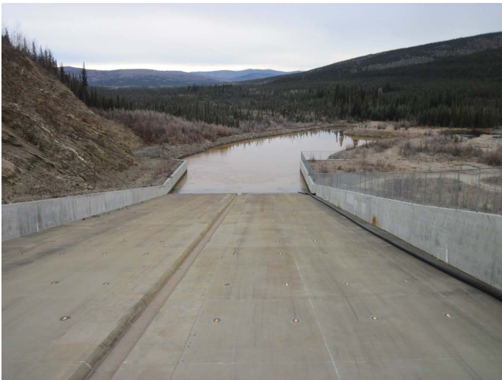
Figure 7. Spillway, looking downstream, at Ft. Knox freshwater dam (October 2010).
