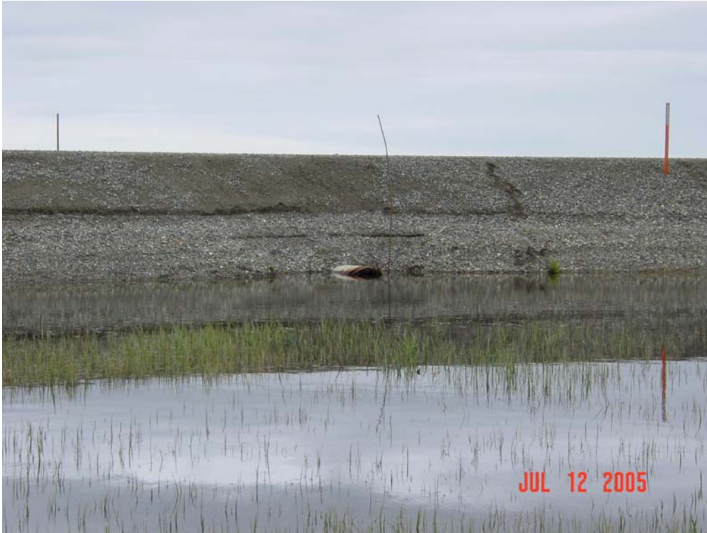
Photograph 43. Unnamed Drill Site 16 Creek culvert inlet. Highwater mark can be observed significantly above the culvert inlet.
