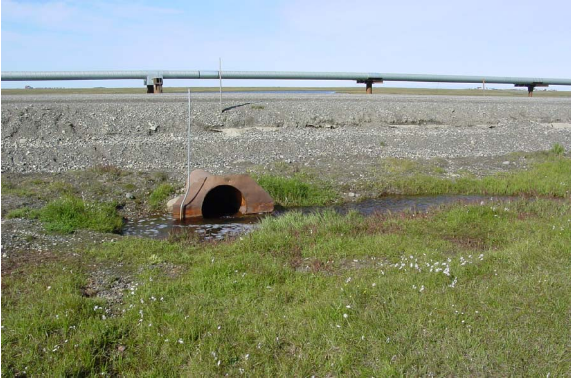
Photograph 213. Milne B Pad Creek culvert inlet with high water mark several feet above the culvert.
