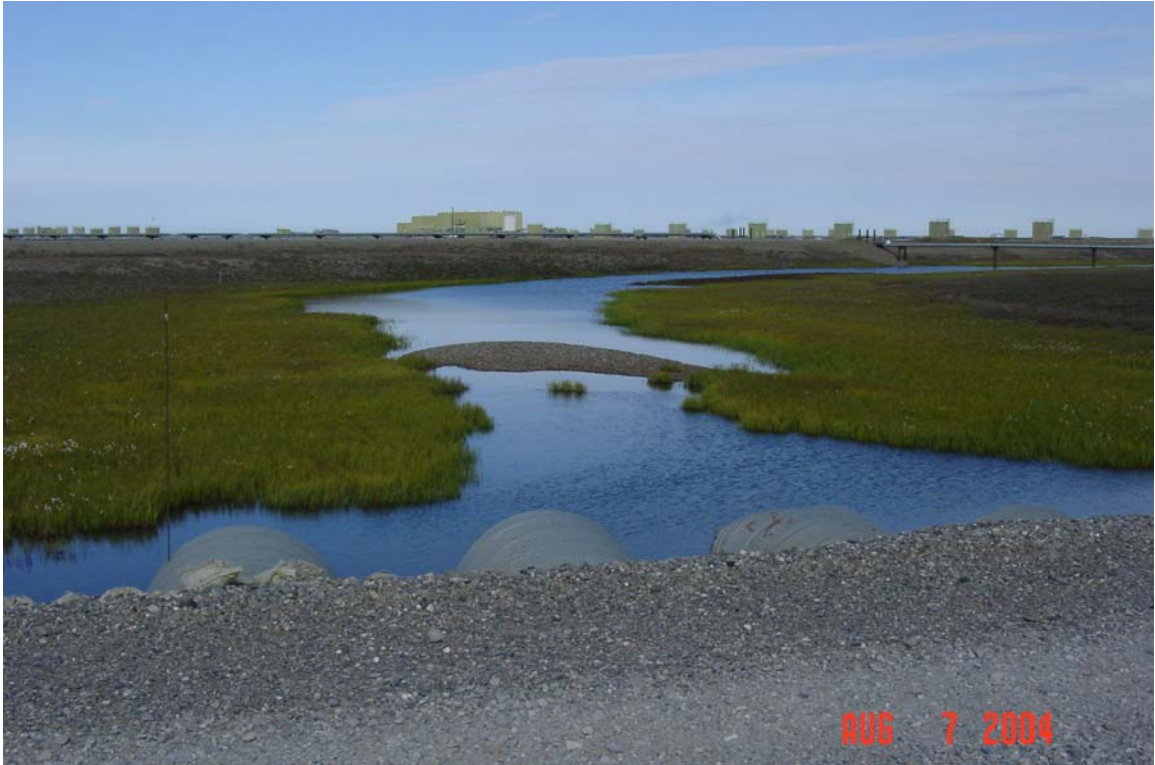
Photograph 4. Washout Creek downstream of road. Gravel outwash is blocking the entire stream channel at the flow conditions present during the inspection.
