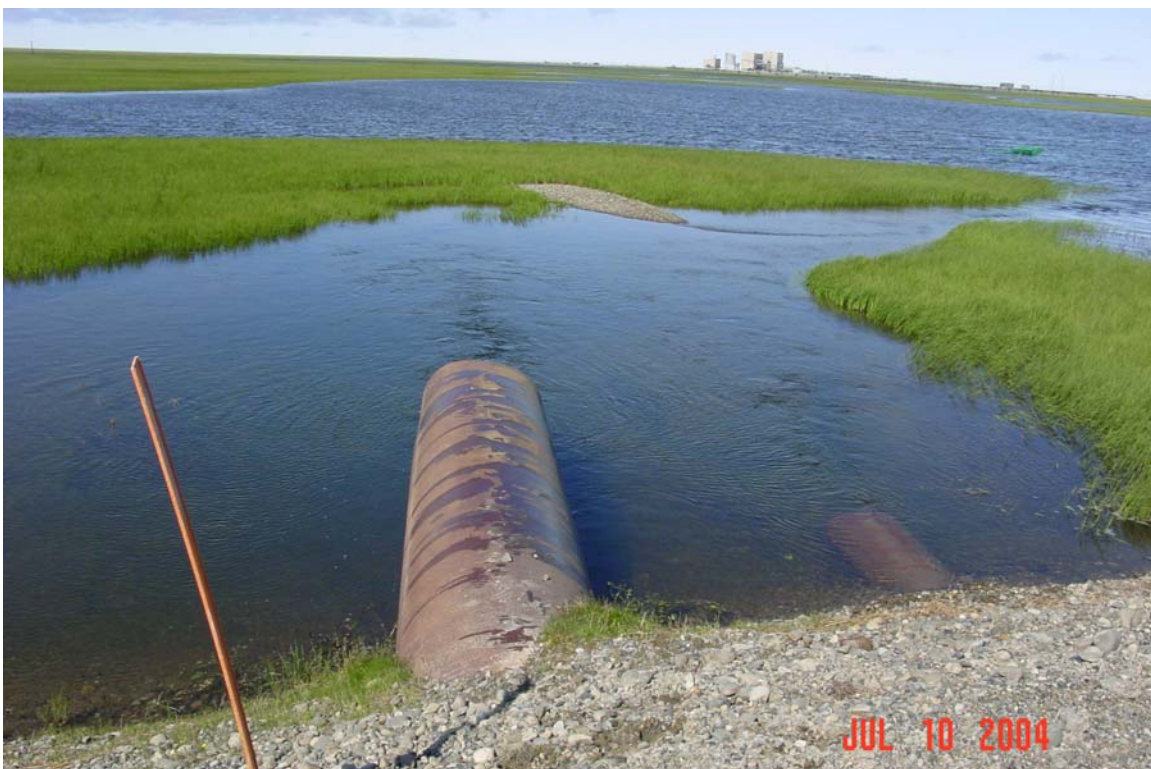
Photograph 111. Fawn Creek downstream of the Spine Road to F-Pad Road access. Limited gravel outwash and deep scour pool present. The larger pipe is elevated considerably above the scoured stream bed.
