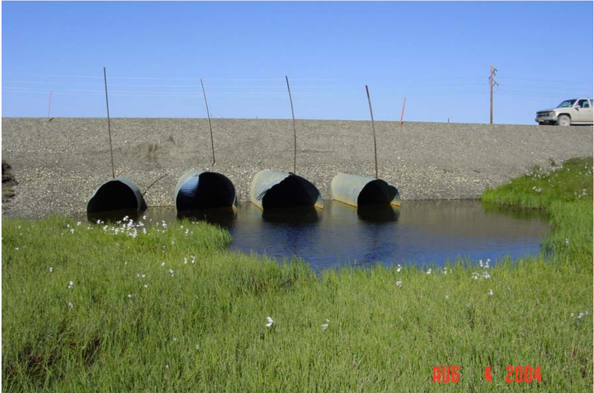
Photograph 313. West Fork Nowhere Creek culvert inlets with the high water mark about 1 foot above the inlets.
