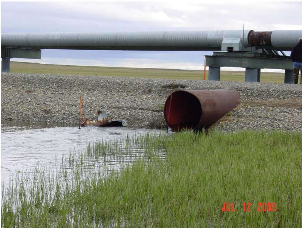
Photograph 47. Unnamed Drill Site 16 Creek culvert outlets at the work pad crossing. Note the damaged to corrugated pipe and the perched smooth wall pipe.
