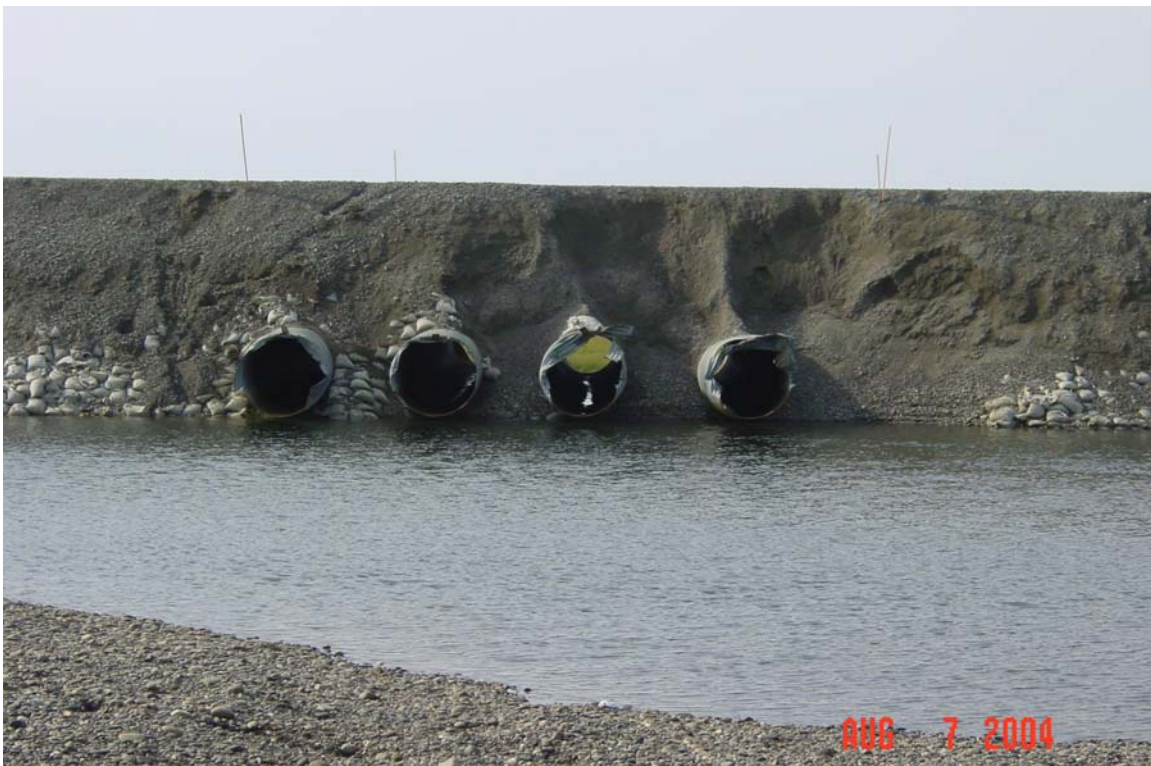
Photograph 99. Little Putuligayuk River culvert outlets, with gravel outwash berm, road erosion and severe culvert damage.
