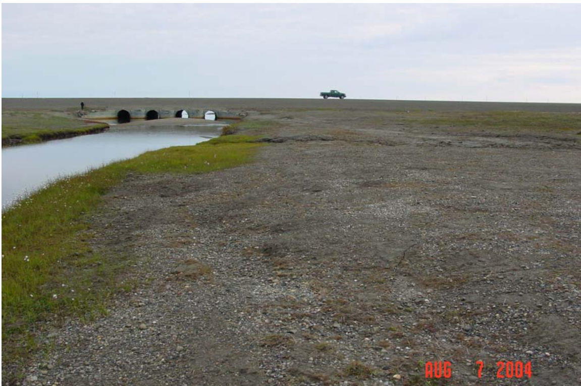
Photograph 87. Little Putuligayuk River old low water crossing looking downstream to the West Dock Road. Significant gravel outwash onto surrounding tundra is present.
