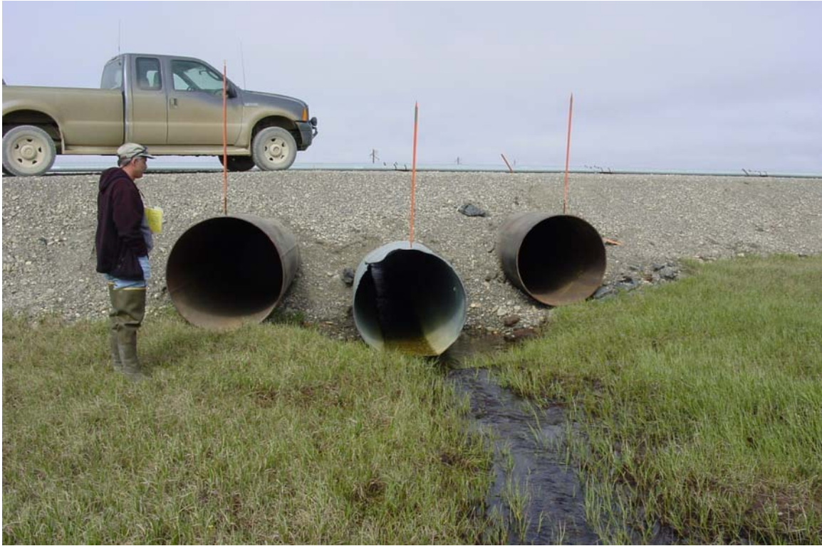
Photograph 380. Kalubik Creek tributary culvert inlets.
