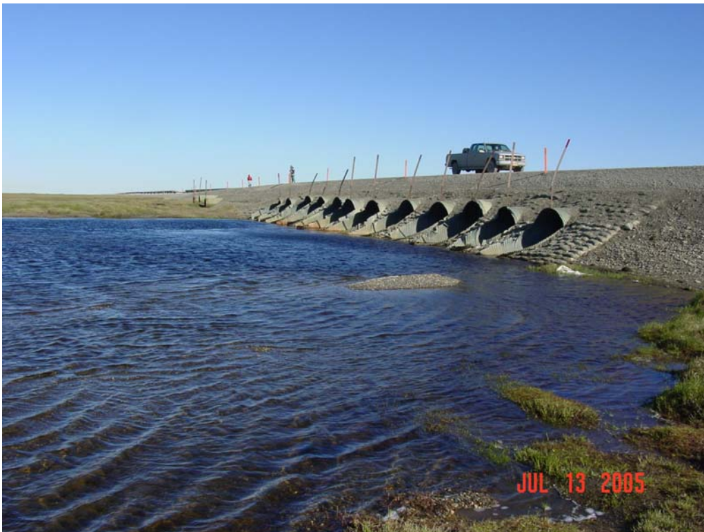
Photograph 143. Sakonowak River culvert outlets, with gravel outwash in the foreground and additional highwater pipes in the background.
