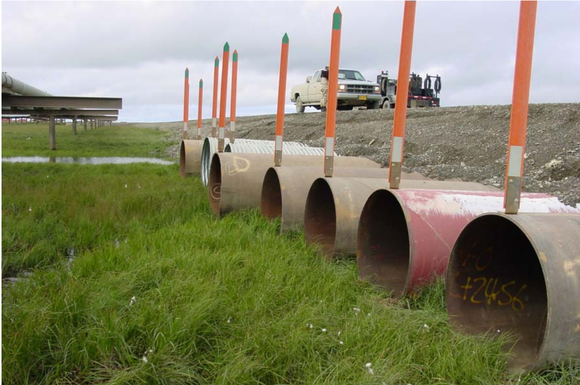
Photograph 227. West Fork West Fork Central Creek culvert inlets misaligned with creek and blocked by vegetation, August 8, 2006.
