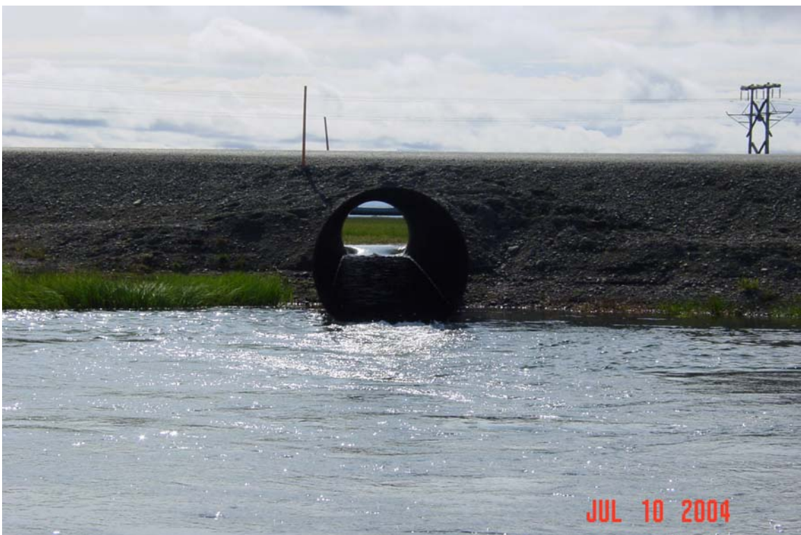
Photograph 125. Fawn Creek culvert outlet. Significant drop in elevation as water enters the pipe at the upstream side of the crossing occurs with a resultant increased velocity.
