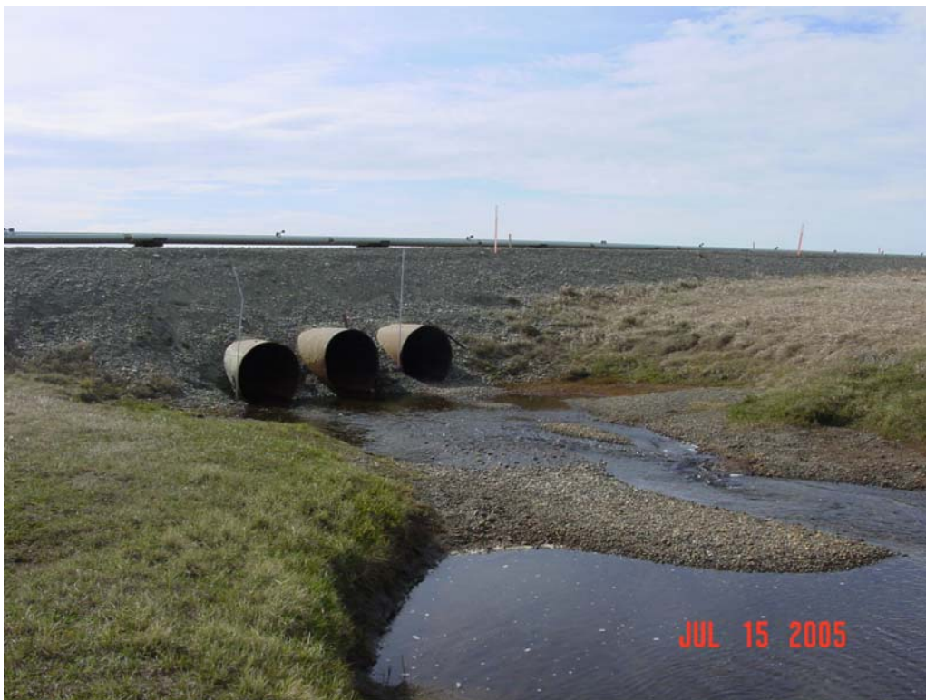
Photograph 208. Lower West Central Creek culvert outlets with outwash gravels.
