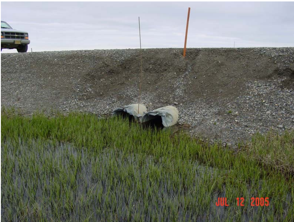
Photograph 40. Damaged culvert inlets of an unnamed Drill Site 16 Creek.
