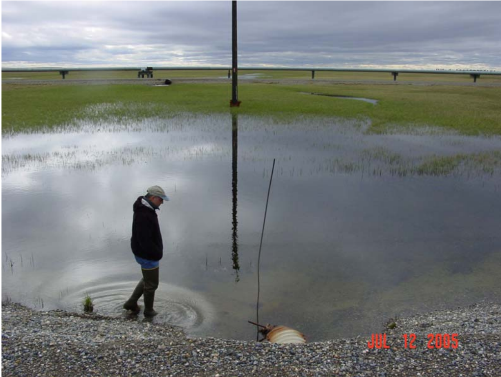
Photograph 41. Unnamed Drill Site 16 Creek upstream of road. Culvert inlet is partially blocked.
