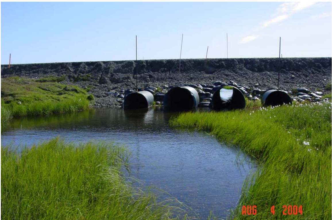
Photograph 314. West Fork Nowhere Creek culvert outlets.
