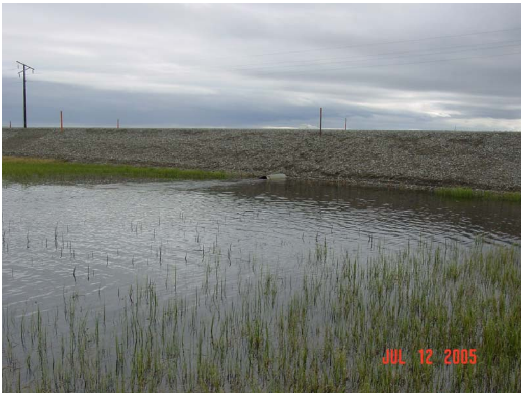
Photograph 44. Unnamed Drill Site 16 Creek culvert outlet. Highwater mark is present above outlet.
