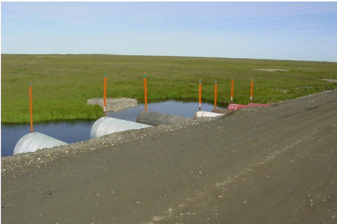
Photograph 248. West Fork Central Creek scour pool and outwash gravels, August 9, 2006.
