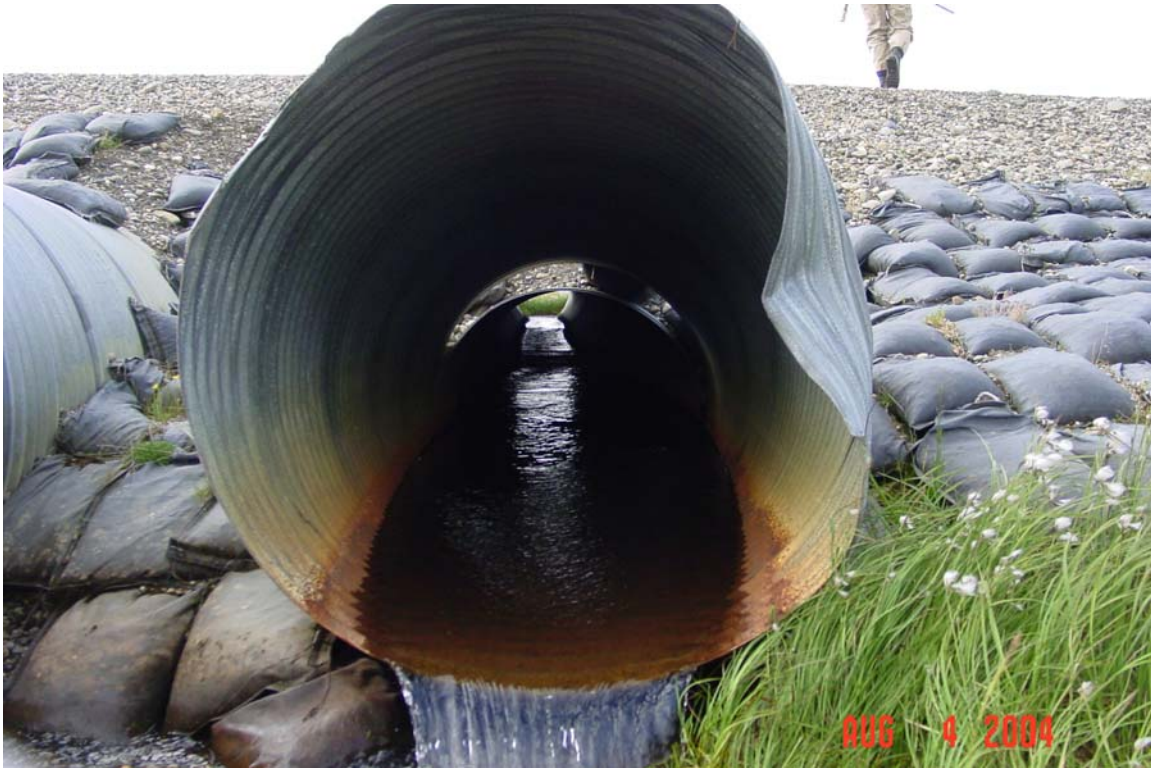
Photograph 362. Perched, split, and bowed culvert in the West Fork Ugnuravik River crossing.
