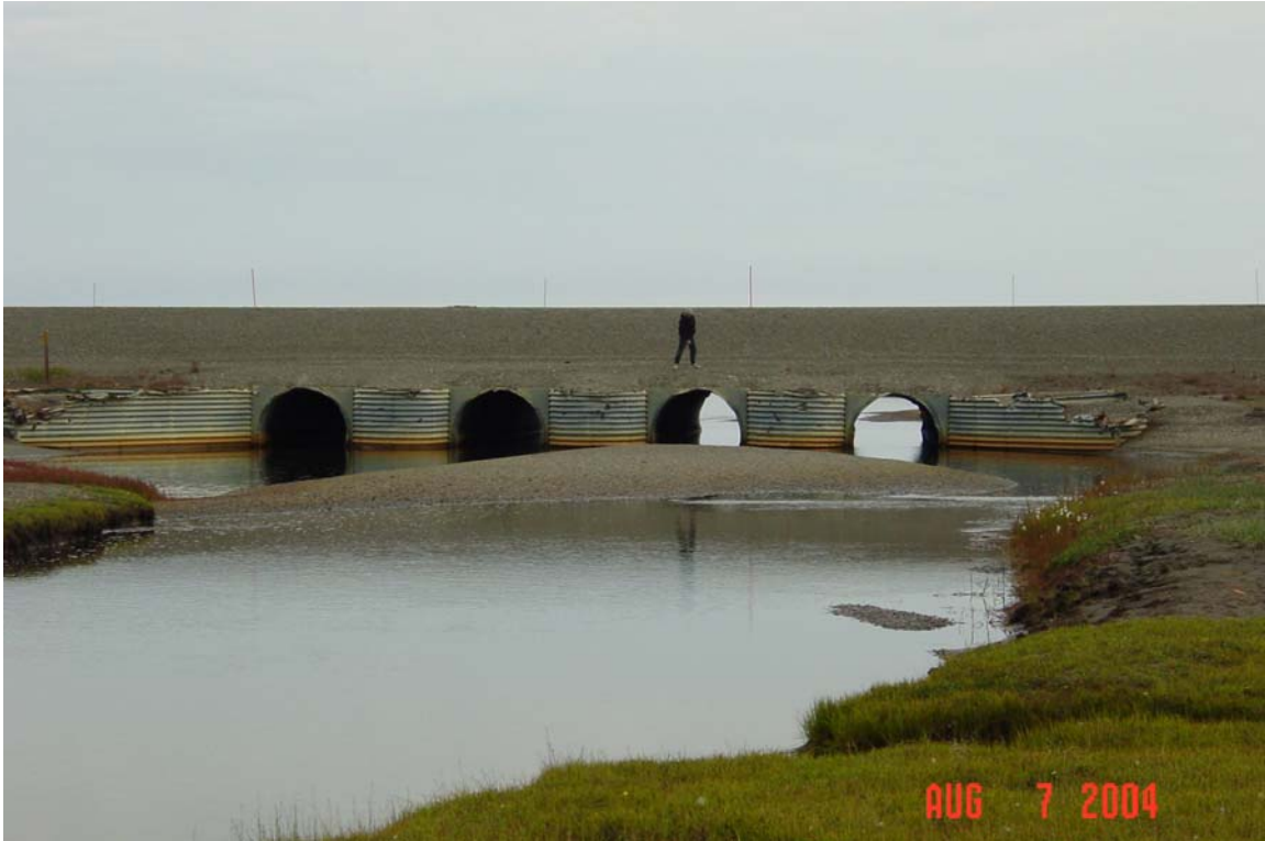
Photograph 84. Little Putuligayuk River culvert inlets. A significant gravel bar has formed in front of the culverts. Damaged inlet armoring is present. The high water mark is above the culverts.
