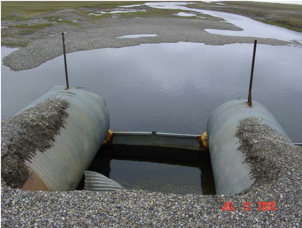
Photograph 33. Washout Creek looking downstream at damaged culvert armoring and gravel outwash.
