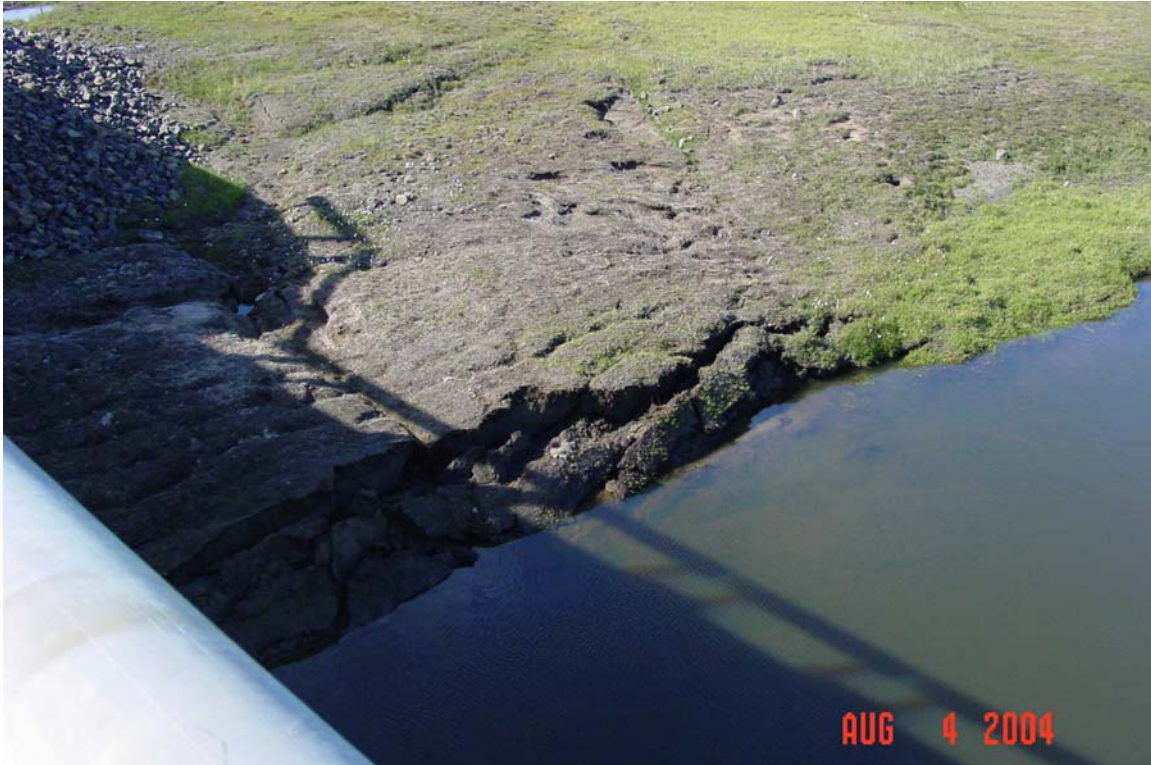
Photograph 317. Bank scour and slumping on the west bank downstream of the bridge.
