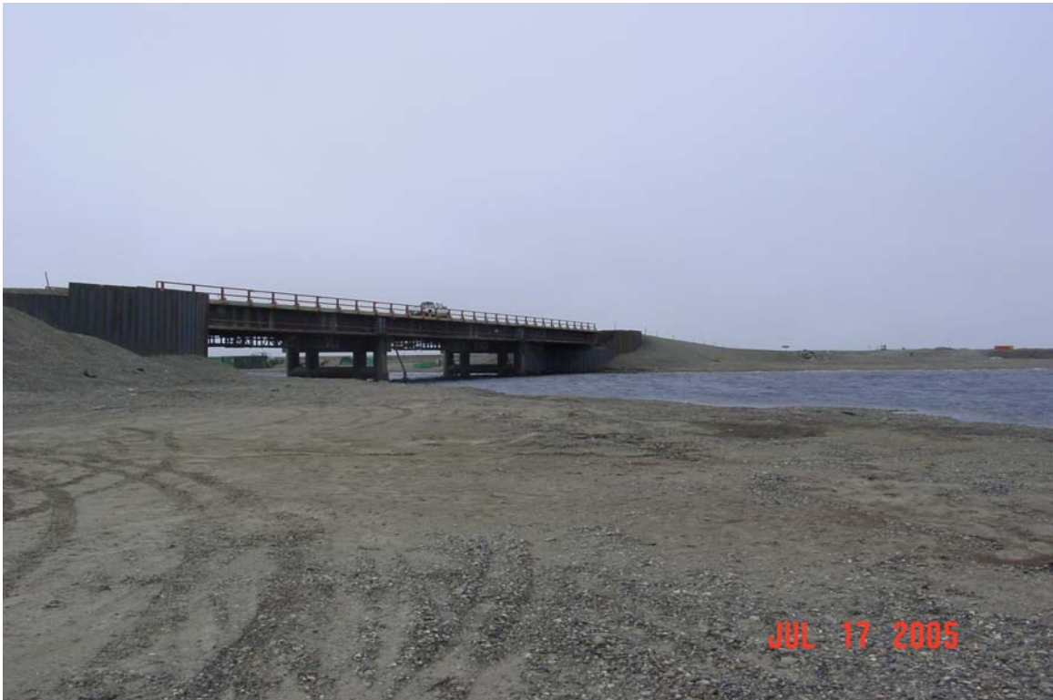
Photograph 186. Kugaruk River Central Channel bridge final repair with sheet pile abutments.
