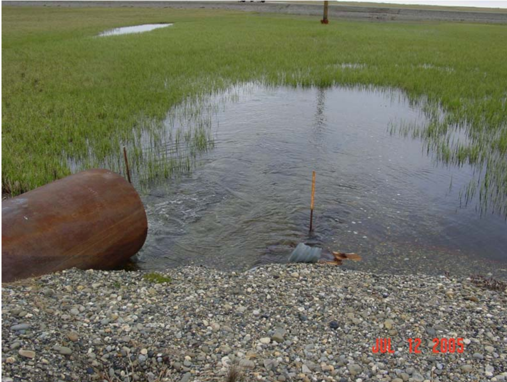
Photograph 45. Unnamed Drill Site 16 Creek downstream of the work pad crossing. Damage to the corrugated pipe can be seen along with significant flow from the perched smooth wall pipe.
