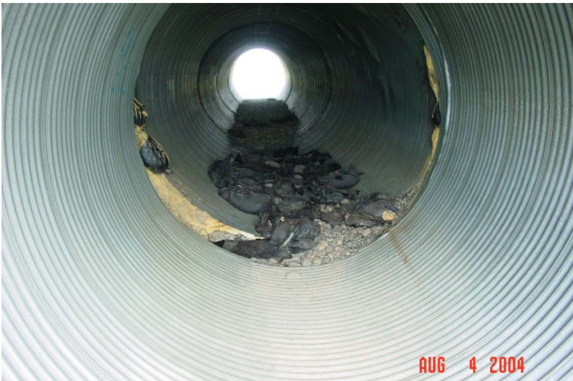
Photograph 387. Kalubik Creek Spine Road crossing split culvert with the split sealed with PolyShield. Sand bags present from inlet erosion.
