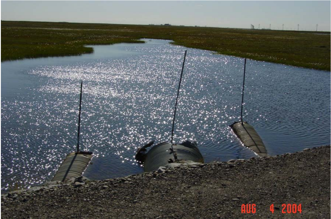
Photograph 296. Caribou Creek upstream of the access road at Drill Site 3B. Damaged inlets.
