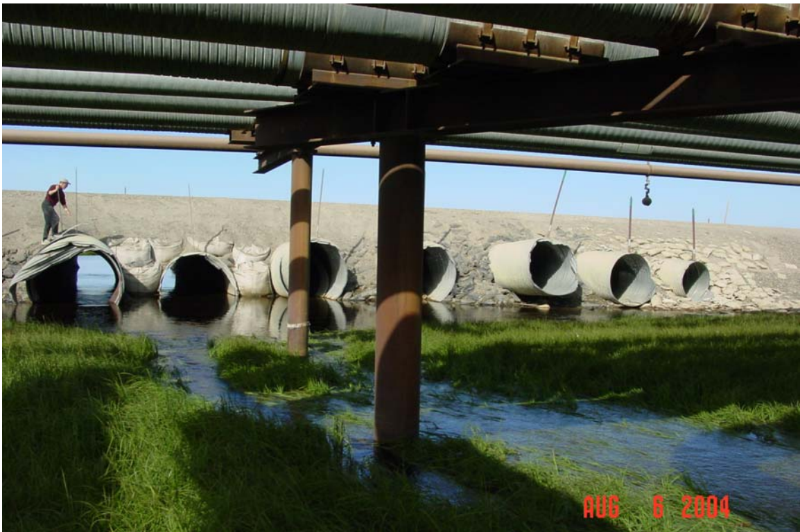
Photograph 258. The eastern half of the Ugnuravik River culvert battery inlets.
