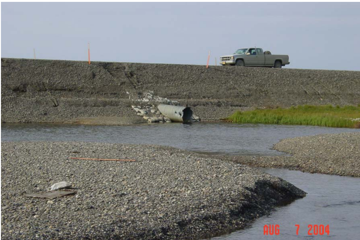
Photograph 101. Little Putuligayuk River culvert outlet, with gravel outwash berm, road erosion and severe culvert damage.
