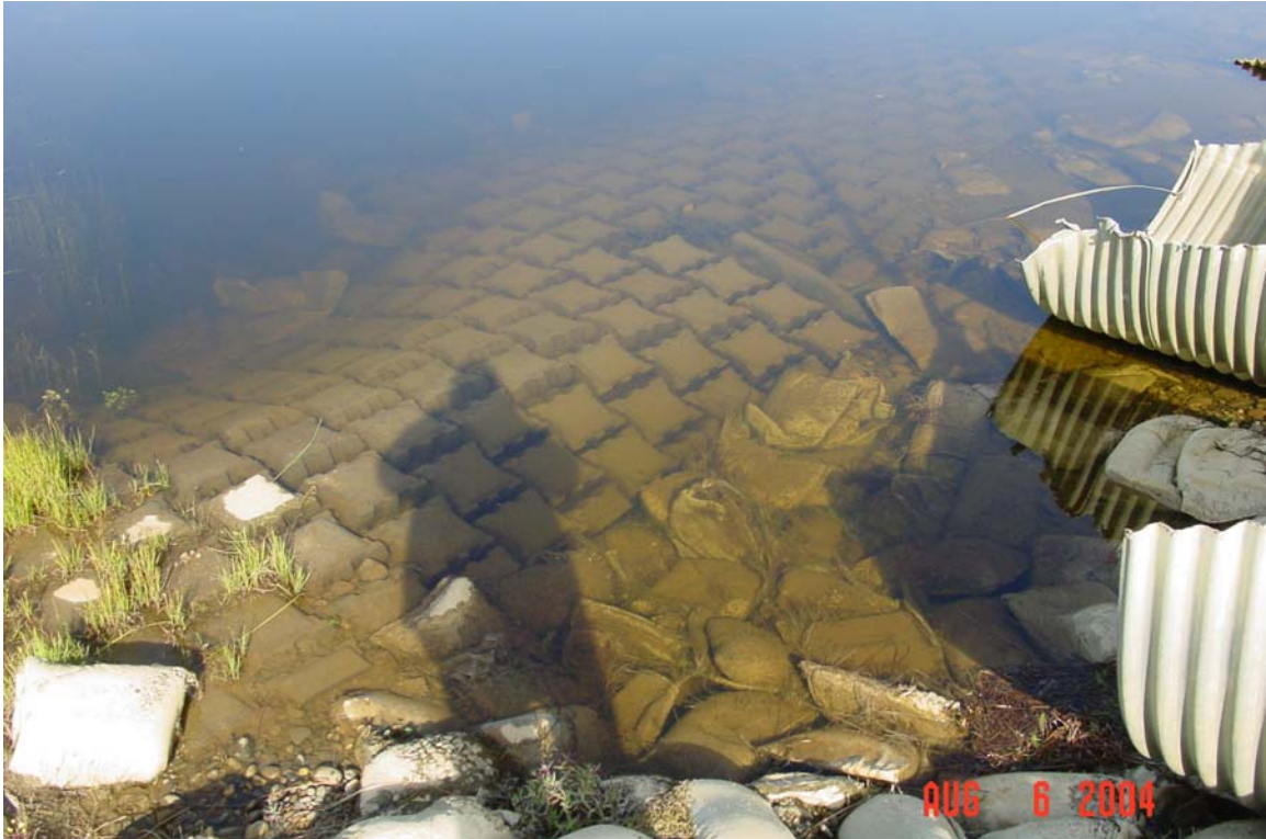
Photograph 259. Slumped and scoured gobi mat, and displaced sand bags at the culvert outlets.
