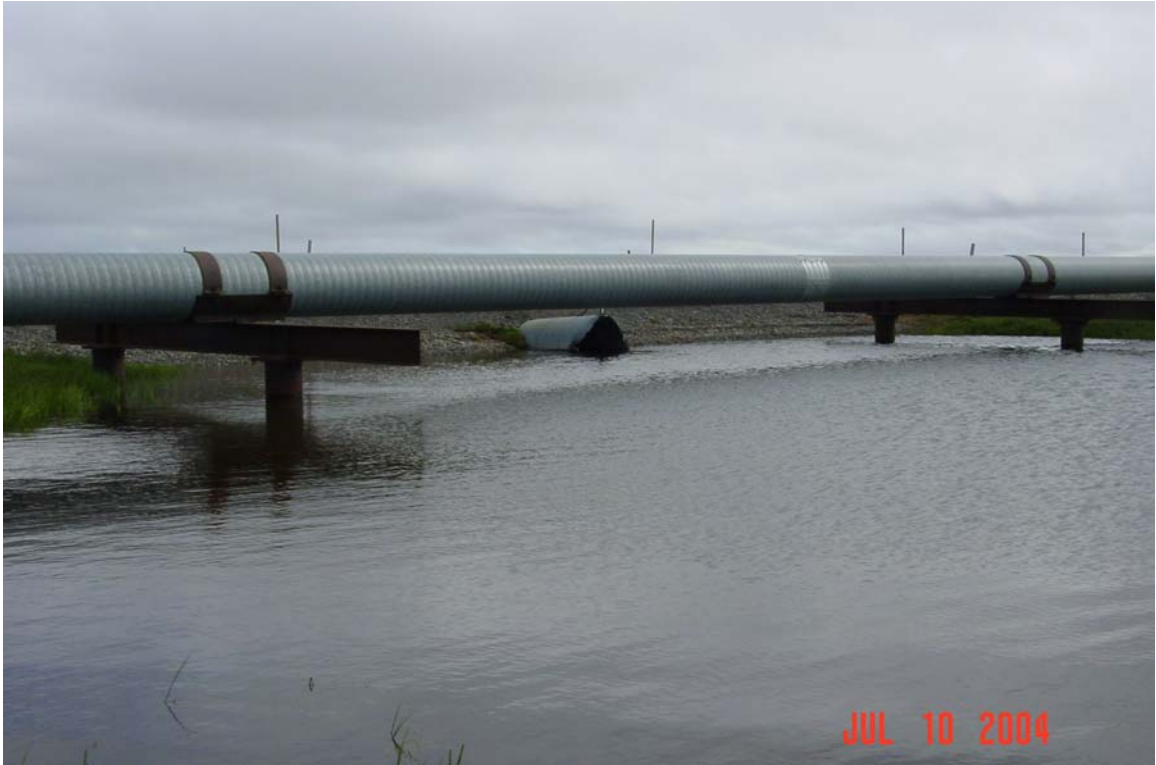
Photograph 116. Fawn Creek culvert inlet. Minimal inlet damage.
