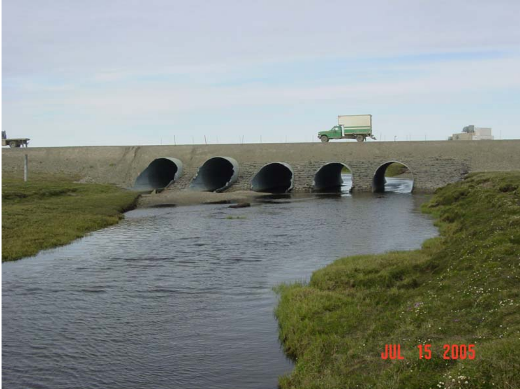
Photograph 161. Smith Creek culvert inlets. The gravel bar was blocking 4 of the 5 culverts during the low flows observed in July 2007.
