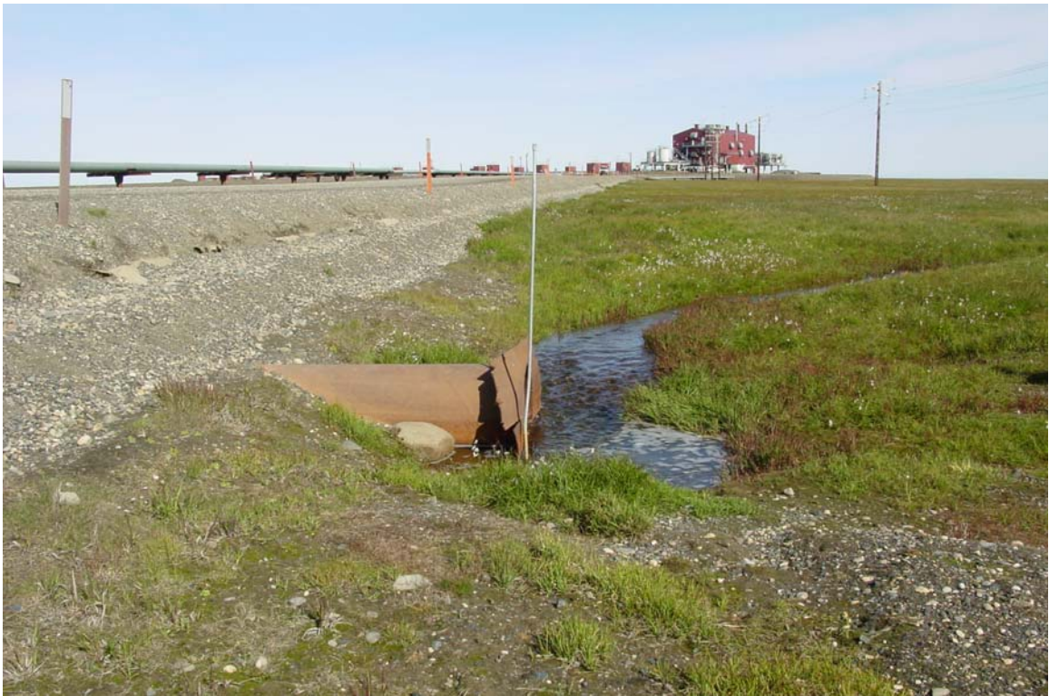
Photograph 214. Milne B Pad Creek culvert inlet misaligned with creek.
