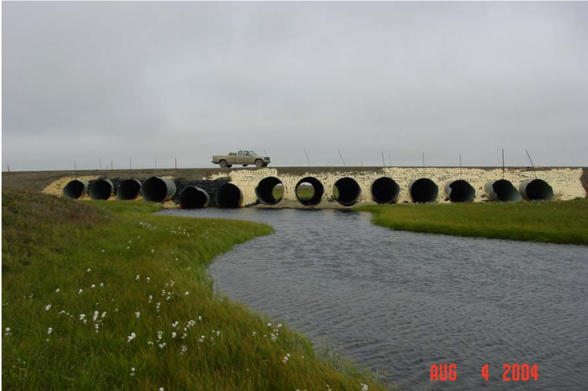
Photograph 384. Culvert inlets at the Kalubik Creek Spine Road crossing. Erosion protection measures include gobi mat, sand bags, concrete aprons, and sand bags sprayed with PolyShield urethane.
