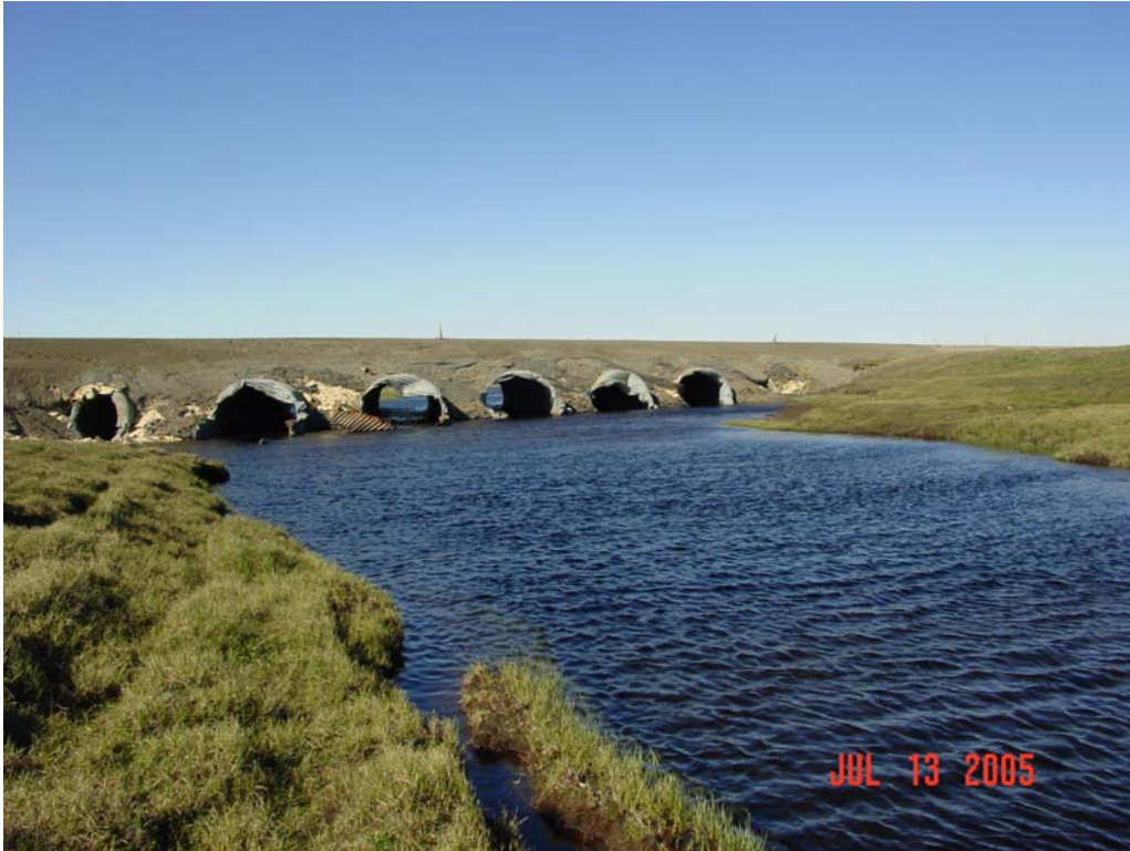
Photograph 146. Smith Creek culvert inlets at the Spine Road crossing.
