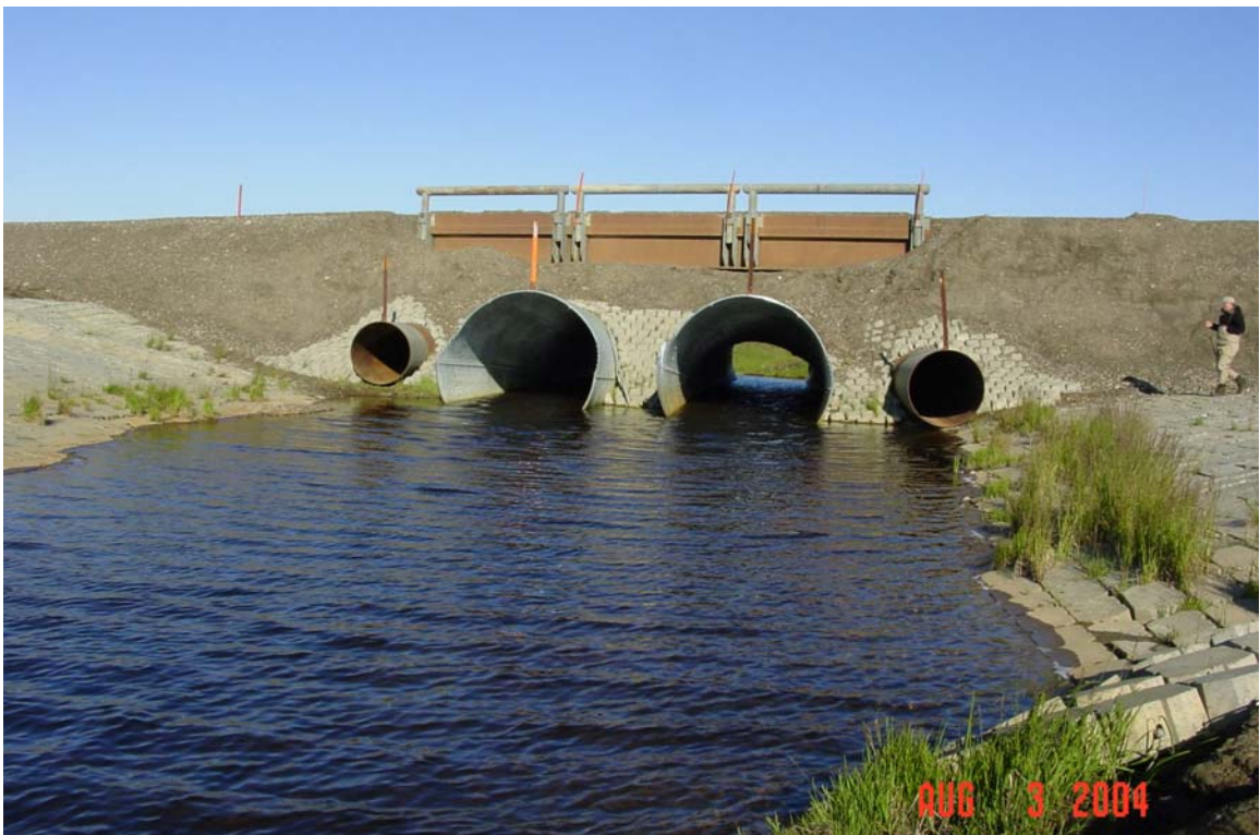
Photograph 409. Kachemach River tributary culvert outlets with extensive gobi mat armoring. Note the steel bridge decking over the partially collapsed 12 foot multiplate culverts.
