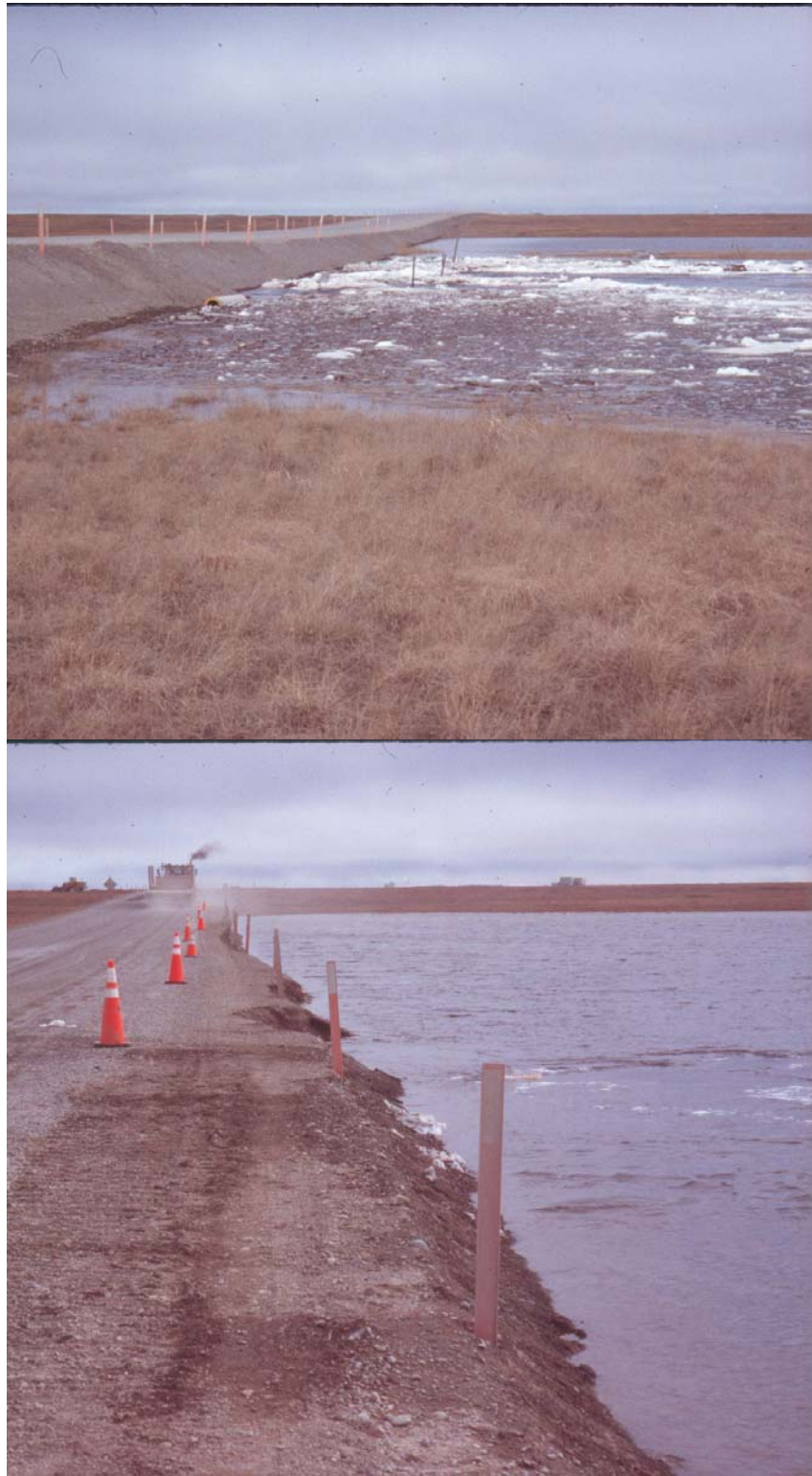
Photograph 148. Smith Creek at Spine road at the upstream side of crossing during break-up, June 9, 2005 (top) and June 10, 2005 (bottom). Flow is significantly impeded, road erosion is occurring and ice is jamming at the crossing.
