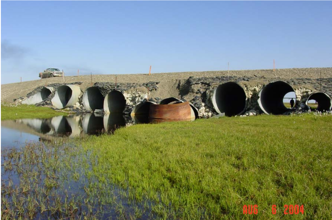
Photograph 264. Ugnuravik River culvert inlets. Note the road prism erosion, sand bag armor destruction, and the culvert apron completely blocking the inlet of one culvert (Repaired by 2006).
