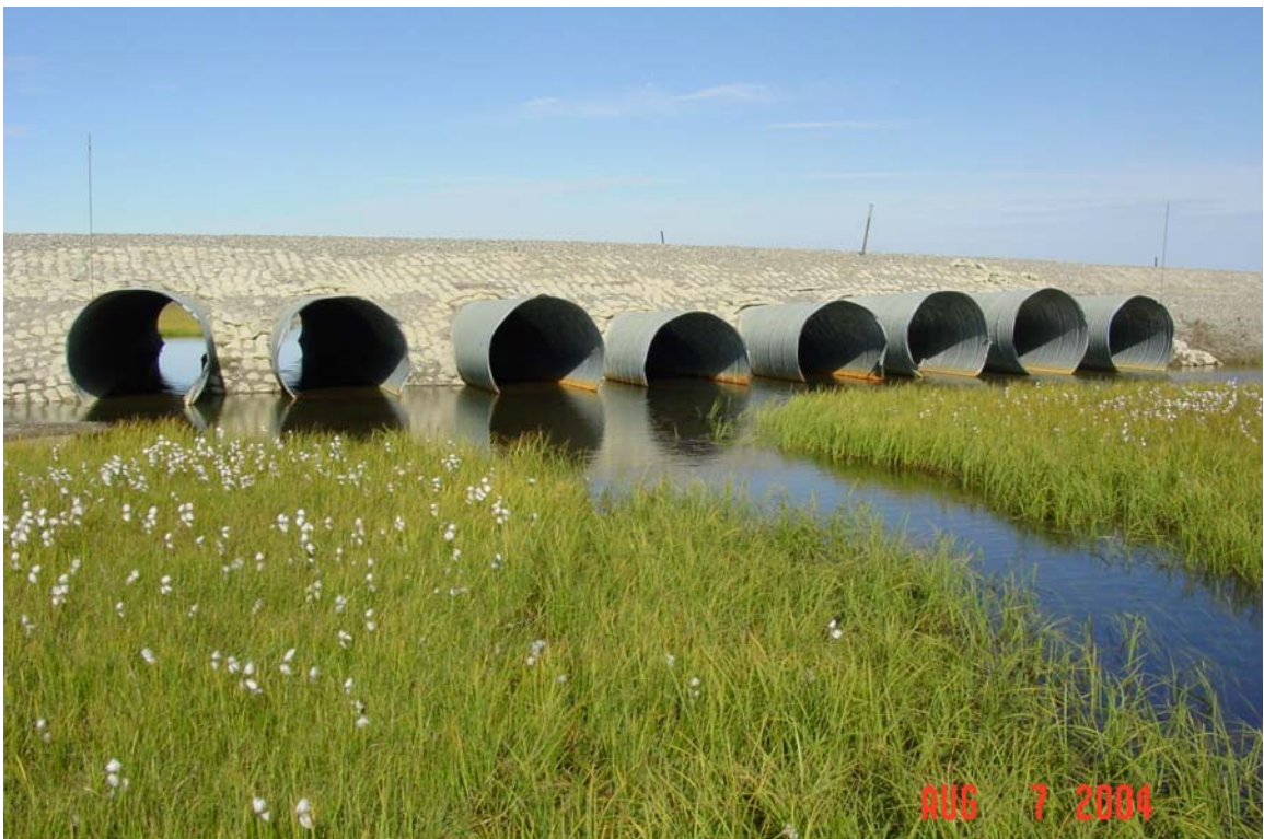
Photograph 7. Washout Creek culvert inlets.
