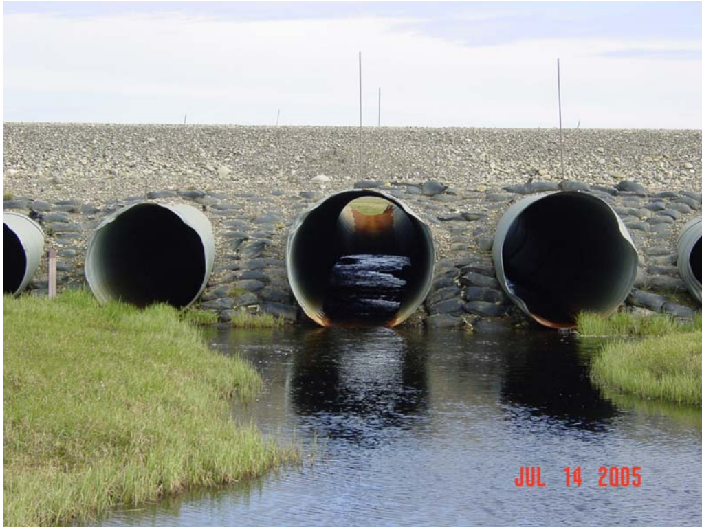
Photograph 373. Water emanating from the center of the Kalubik Creek tributary culvert with the severely bowed and perched inlet.
