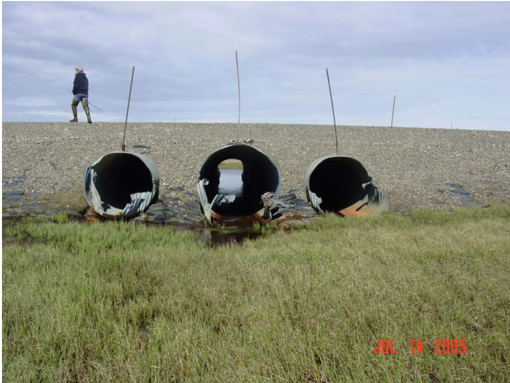
Photograph 339. Damaged Ugnuravik River tributary culvert inlets.
