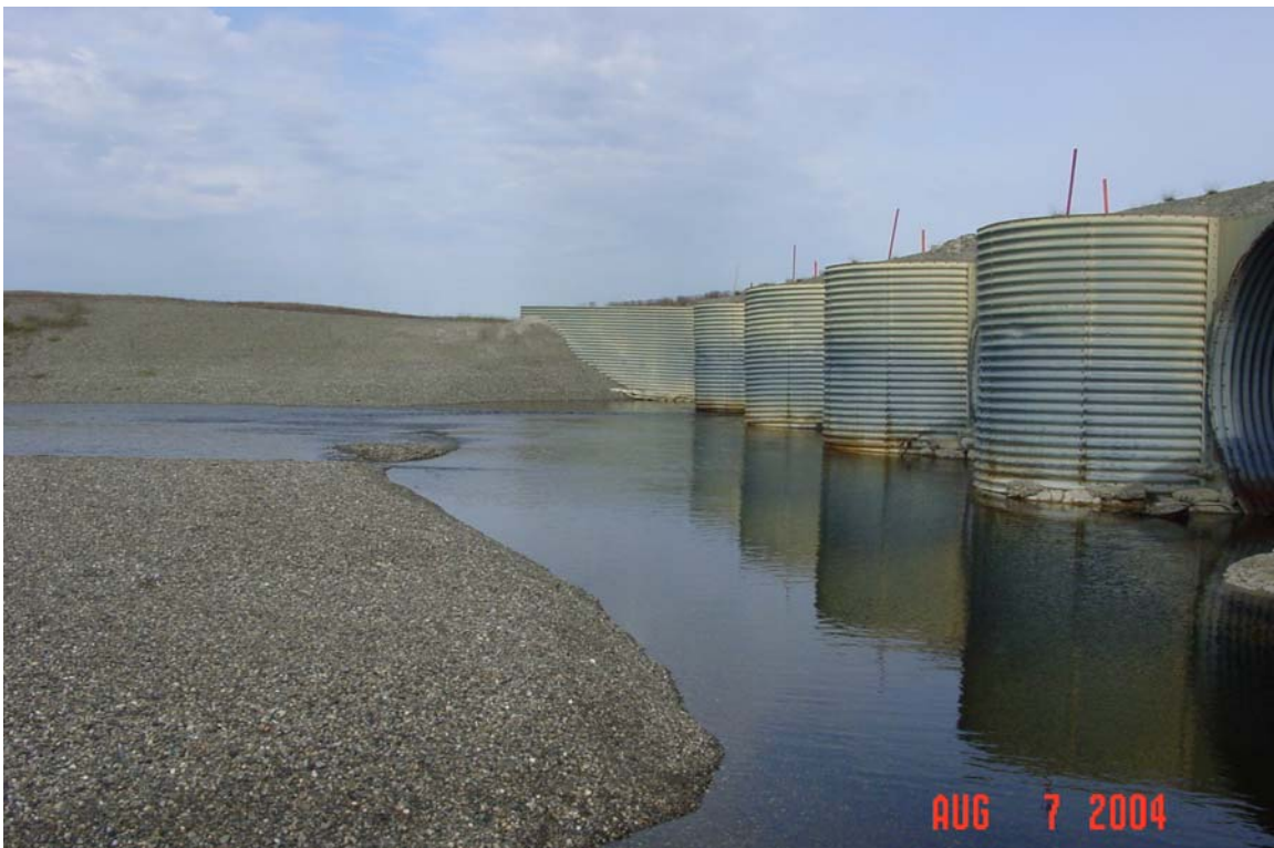
Photograph 71. Putuligayuk River culvert inlets, with extensive gravel bars at the inlets and scour immediately upstream of the culverts.
