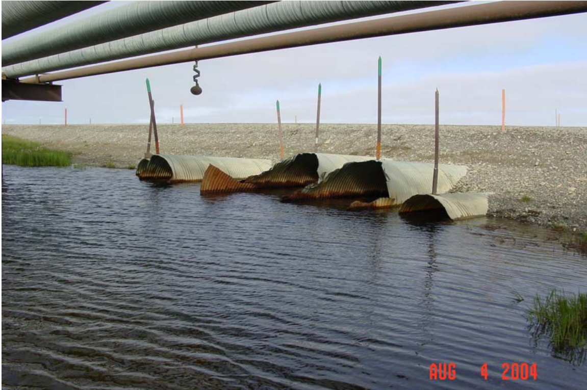
Photograph 358. West Fork Ugnuravik River culvert inlets. Note the high water mark above the culverts and the damaged culvert aprons.
