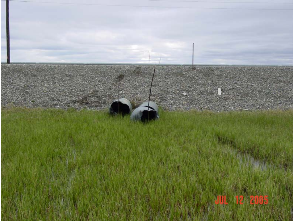
Photograph 39. Damaged culvert outlets of an unnamed Drill Site 16 Creek.
