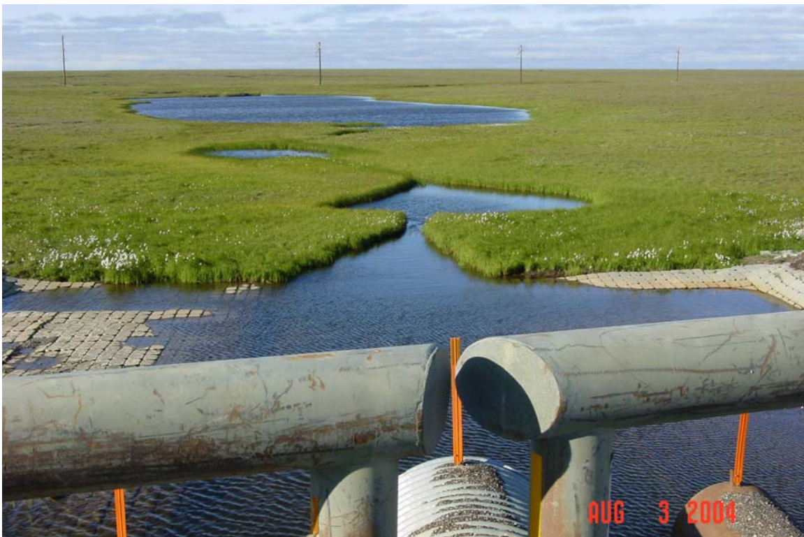
Photograph 402. Miluveach River tributary looking downstream of the crossing structure. Note the extensive gobi mat armor erosion protection.
