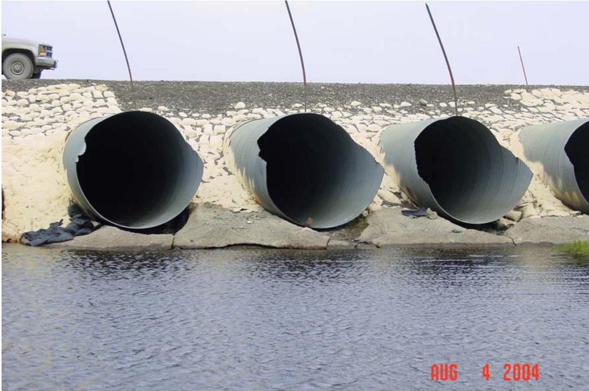
Photograph 386. Kalubik Creek Spine Road crossing culvert inlets with cracked and separated concrete aprons, and urethane coated sand bags.
