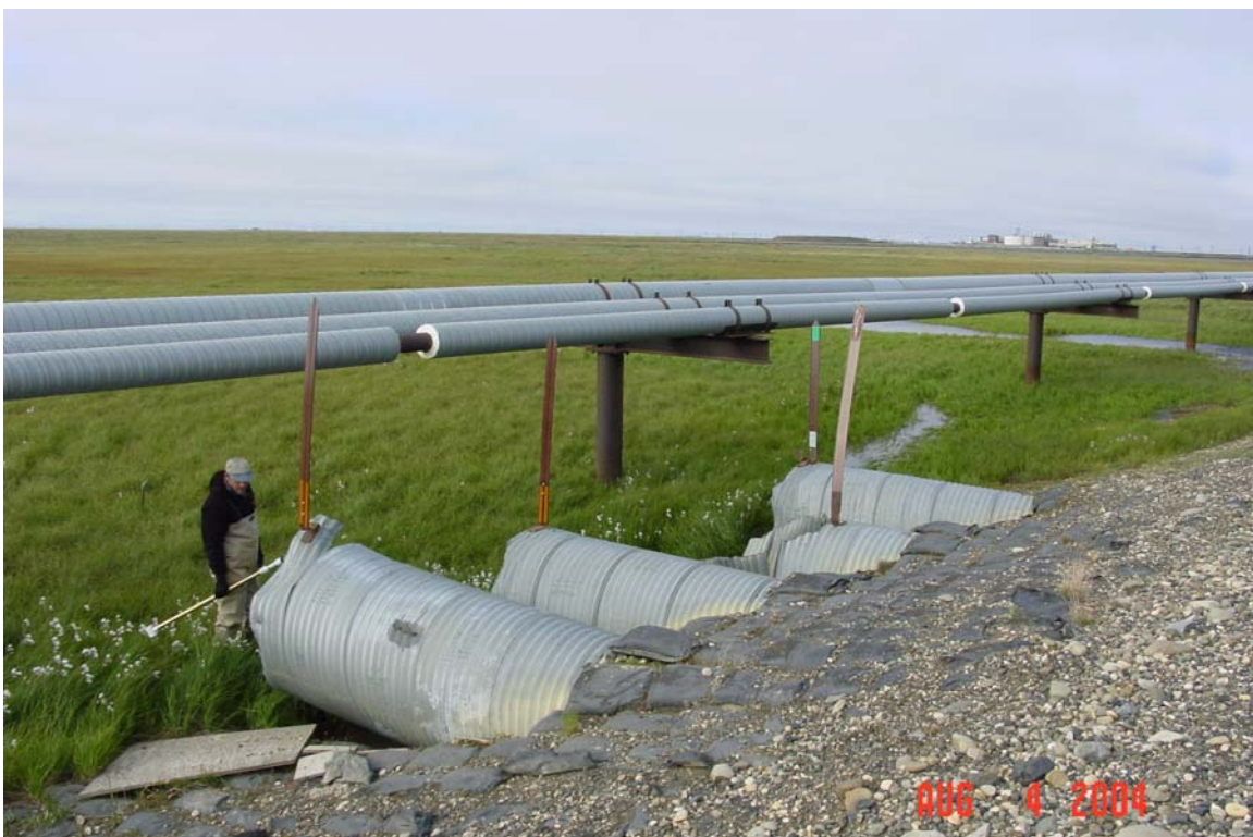
Photograph 363. West Fork Ugnuravik River culvert inlets. Note the stream approaching from the right, and the perched and damaged inlets.
