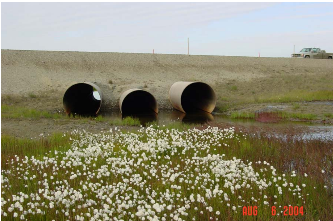
Photograph 130. Leach Creek culvert inlets. High water mark is at or just above pipes.
