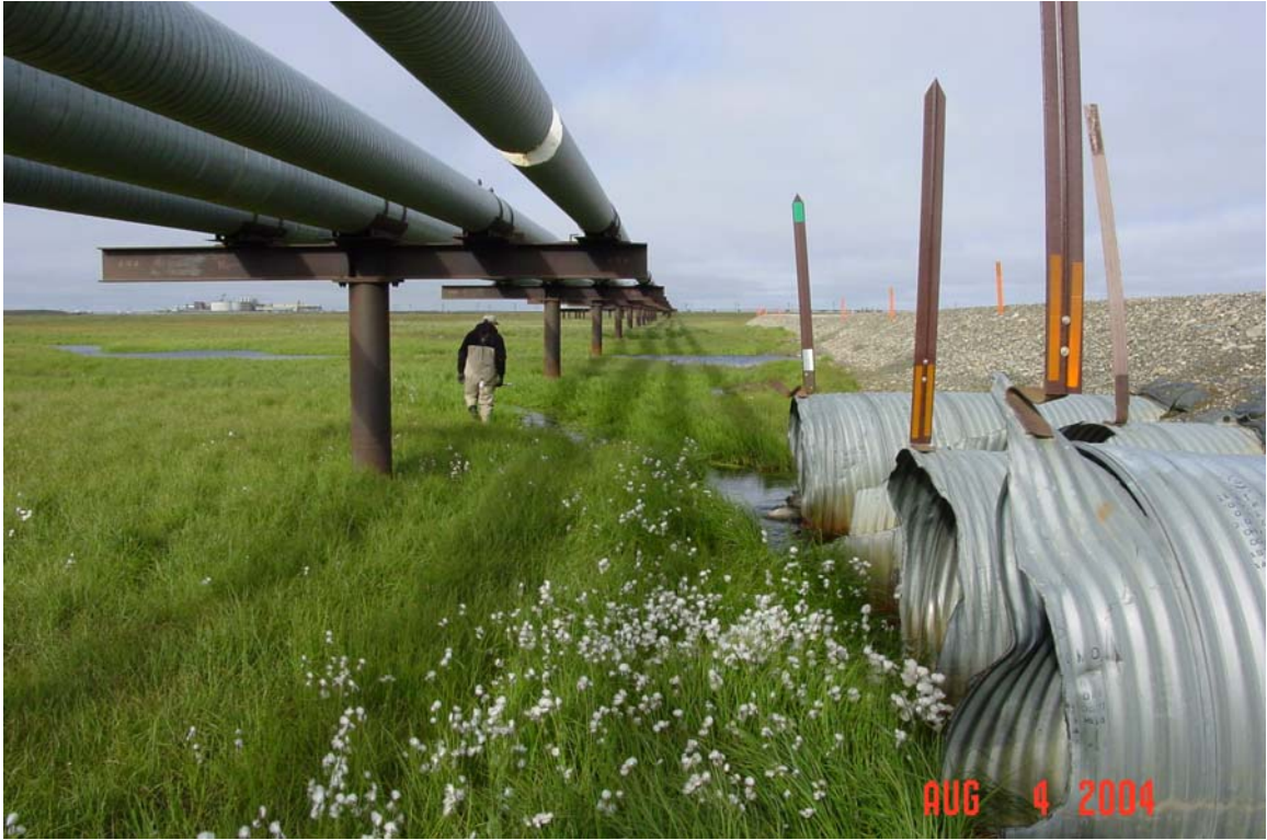
Photograph 364. West Fork Ugnuravik River damaged culvert inlets.
