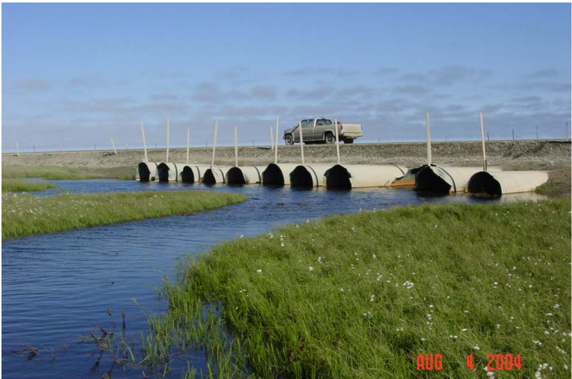
Photograph 289. West Fork Ugnuravik River tributary culvert inlets.
