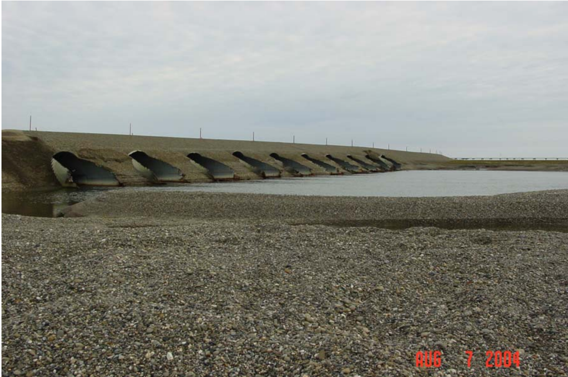
Photograph 66. Putuligayuk River looking at the downstream side of crossing. Damage to outlets, significant gravel outwash and road prism erosion is evident.
