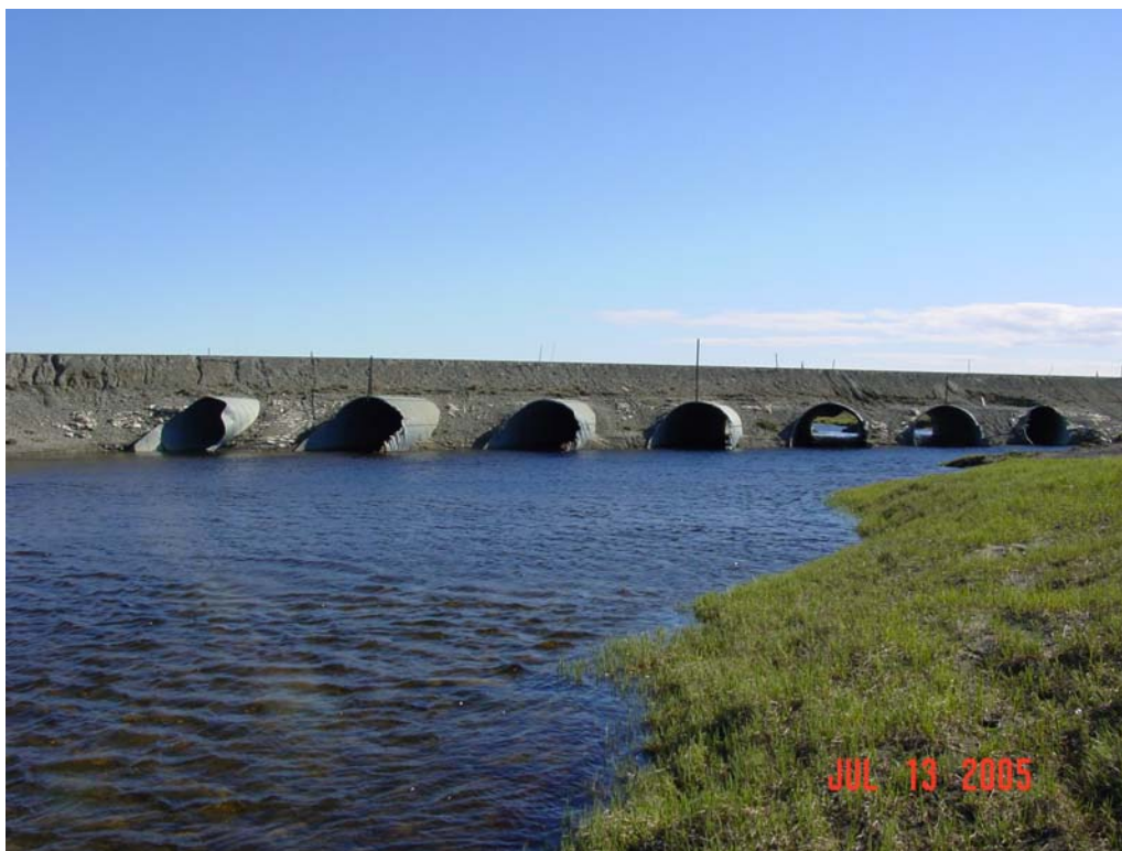
Photograph 149. Smith Creek culvert outlets. Some damage to outlets can be seen as well as some minimal road erosion.
