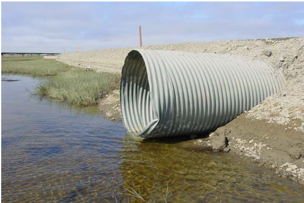
Photograph 236. East Fork Central Creek 48 inch culvert inlet, July 8, 2007. This pipe replaced an existing 24 inch culvert.
