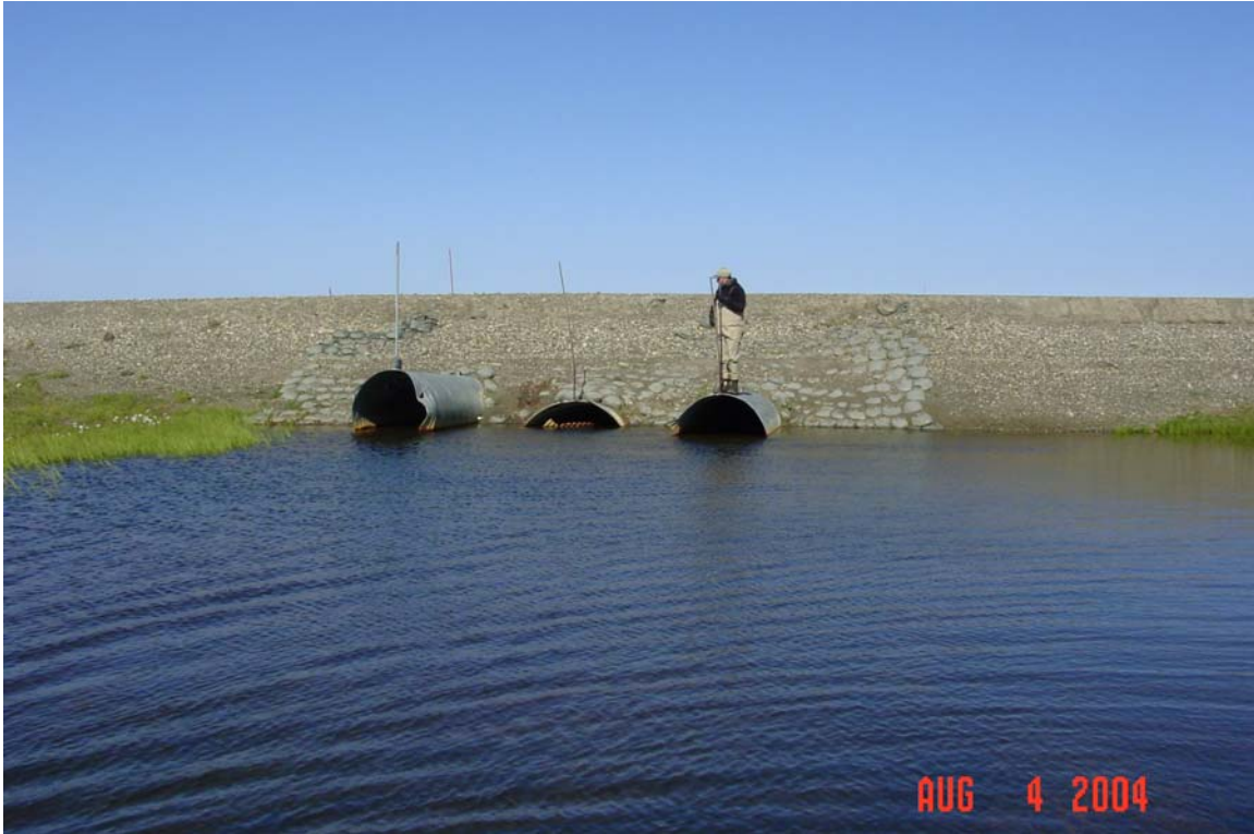
Photograph 302. Kalubik Creek tributary (East Fork Nowhere Creek) damaged culvert inlets and a high water mark about 1 foot above the inlets.
