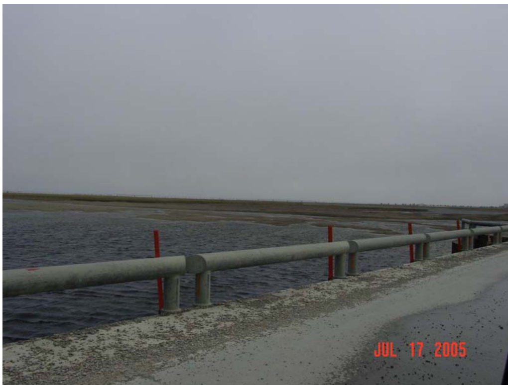
Photograph 190. Kuparuk River West Channel bridge looking downstream and east from bridge. At normal summer water levels, water passes under the bridge into the large scour hole and then is diverted east flowing along the toe of the road prior to regaining northward flow.
