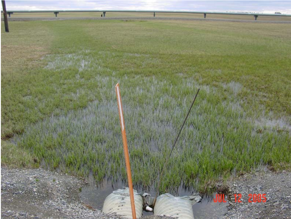
Photograph 37. Unnamed Drill Site 16 Creek upstream of road. Damaged culvert inlets.
