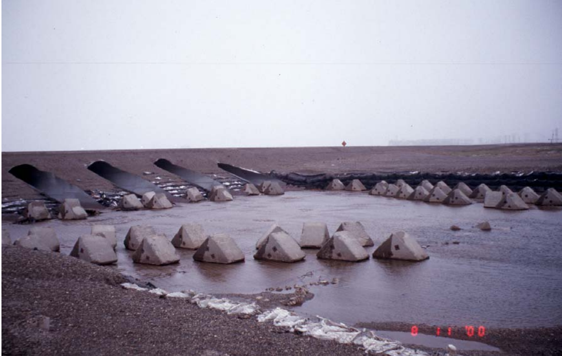
Photograph 76. Putuligayuk River downstream of the Spine Road crossing. Exposed goby mat can be observed at these flow conditions. The structure is likely a complete blockage to both upstream and downstream movement of fish at low flows.
