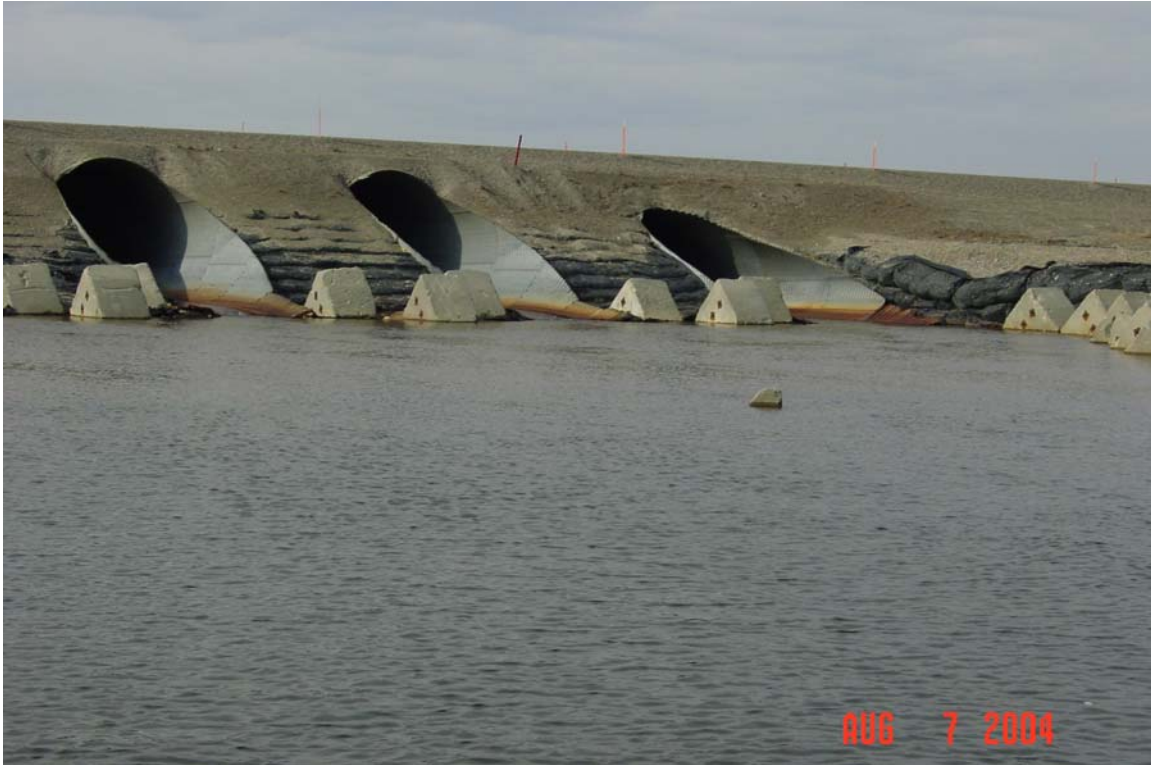
Photograph 74. Putuligayuk River culvert outlets. Culvert aprons slope down to gobi mat creating a chute of water.
