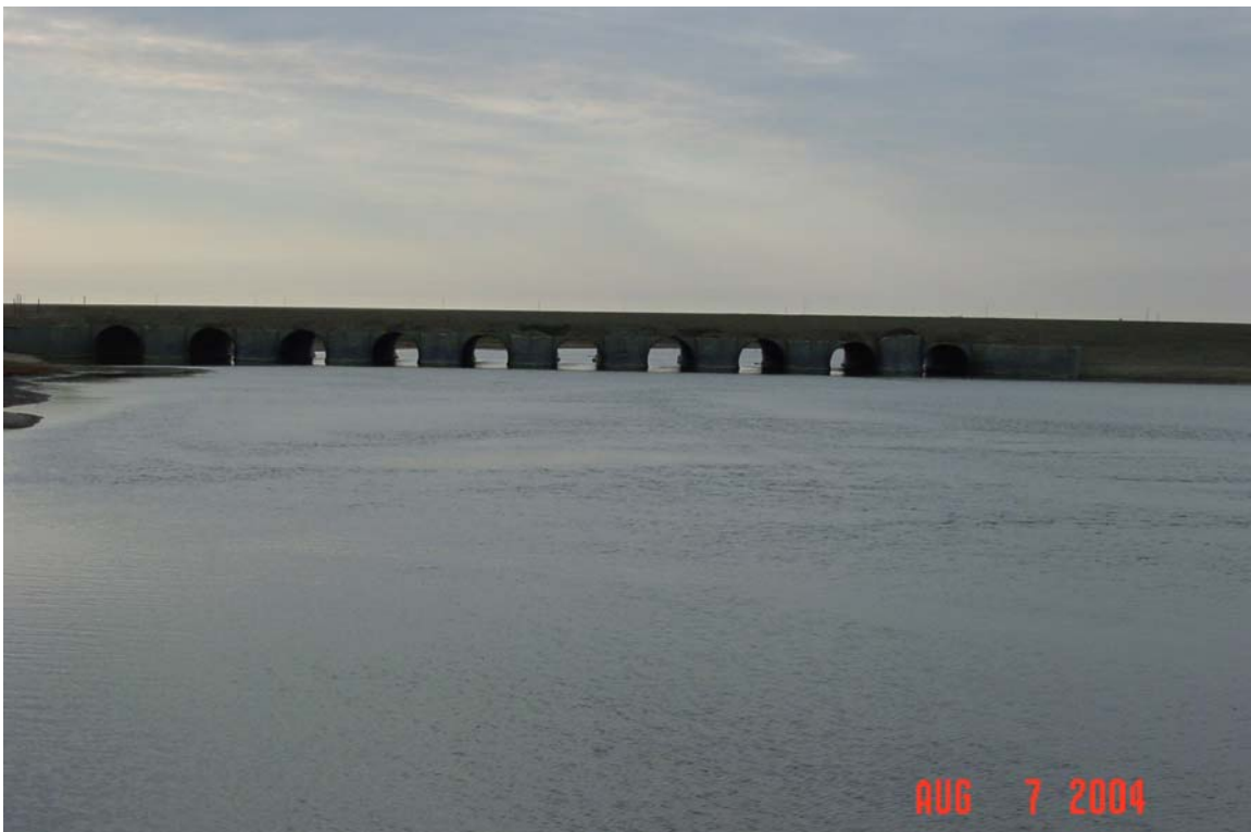
Photograph 67. Putuligayuk River looking at the upstream side of the road crossing. Damage to armor and upstream gravel deposition can be seen.
