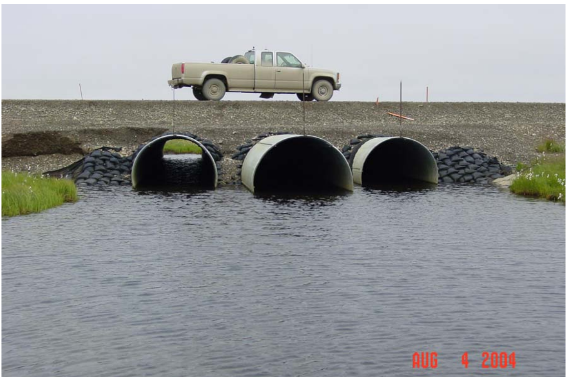
Photograph 392. West Fork Kalubik Creek culvert inlets. Note the road prism erosion.
