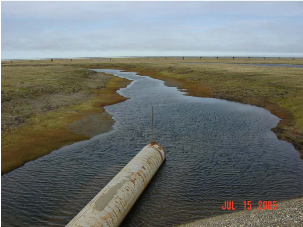
Photograph 209. No Point Creek downstream of the Milne Point F Pad road. Note the excessively long visible pipe with two submerged pipes beneath it.
