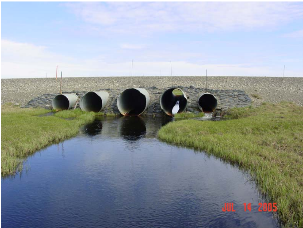
Photograph 372. Kalubik Creek tributary culvert outlets, some of which are perched.
