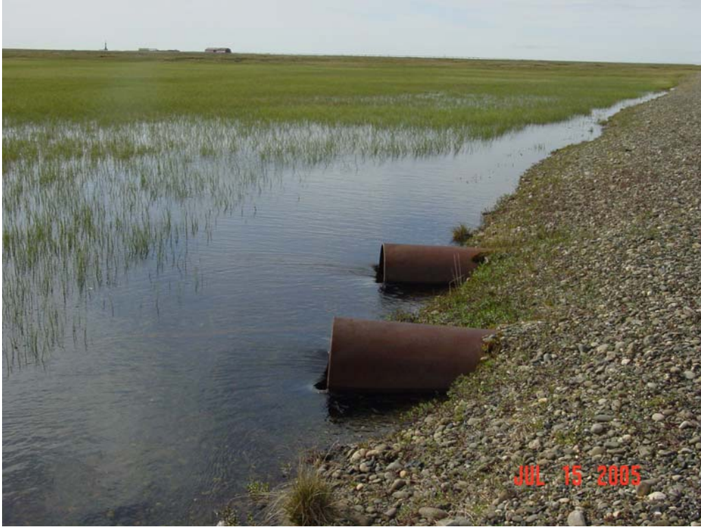
Photograph 174. Exposed Pebble Creek culvert inlets.
