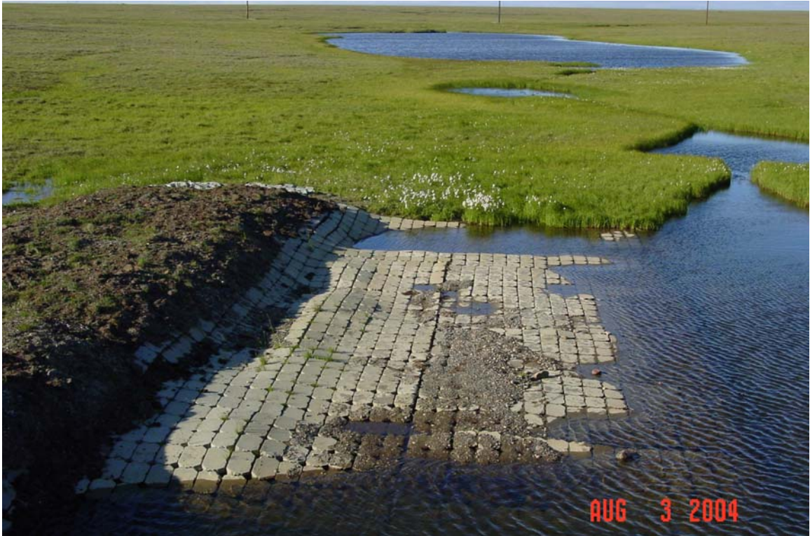
Photograph 405. Soil berms holding the downstream gobi mat armor erosion protection.
