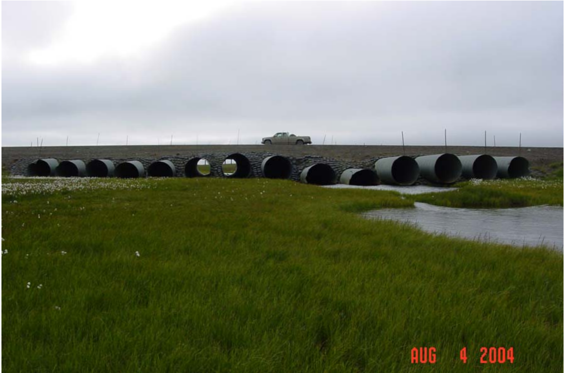
Photograph 388. Kalubik Creek Spine Road culvert outlets.
