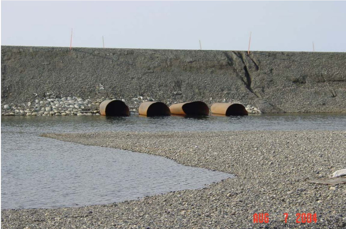
Photograph 100. Little Putuligayuk River culvert outlets, with gravel outwash berm, road erosion and severe culvert damage.
