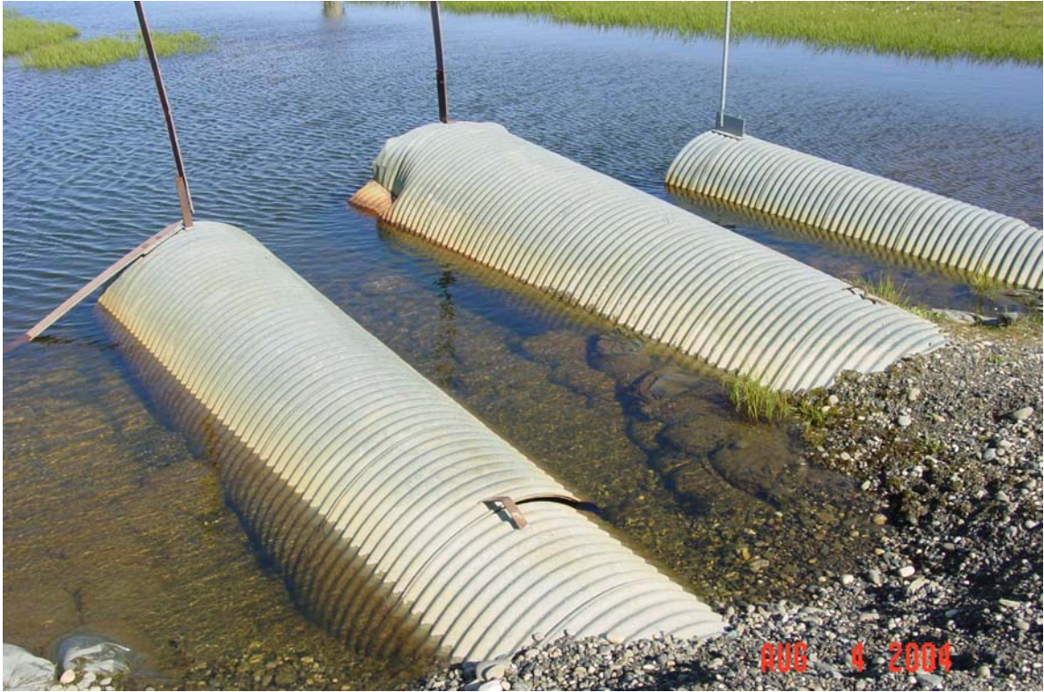
Photograph 304. Kalubik Creek tributary (East Fork Nowhere Creek) culvert outlets that are excessively long, damaged and split.
