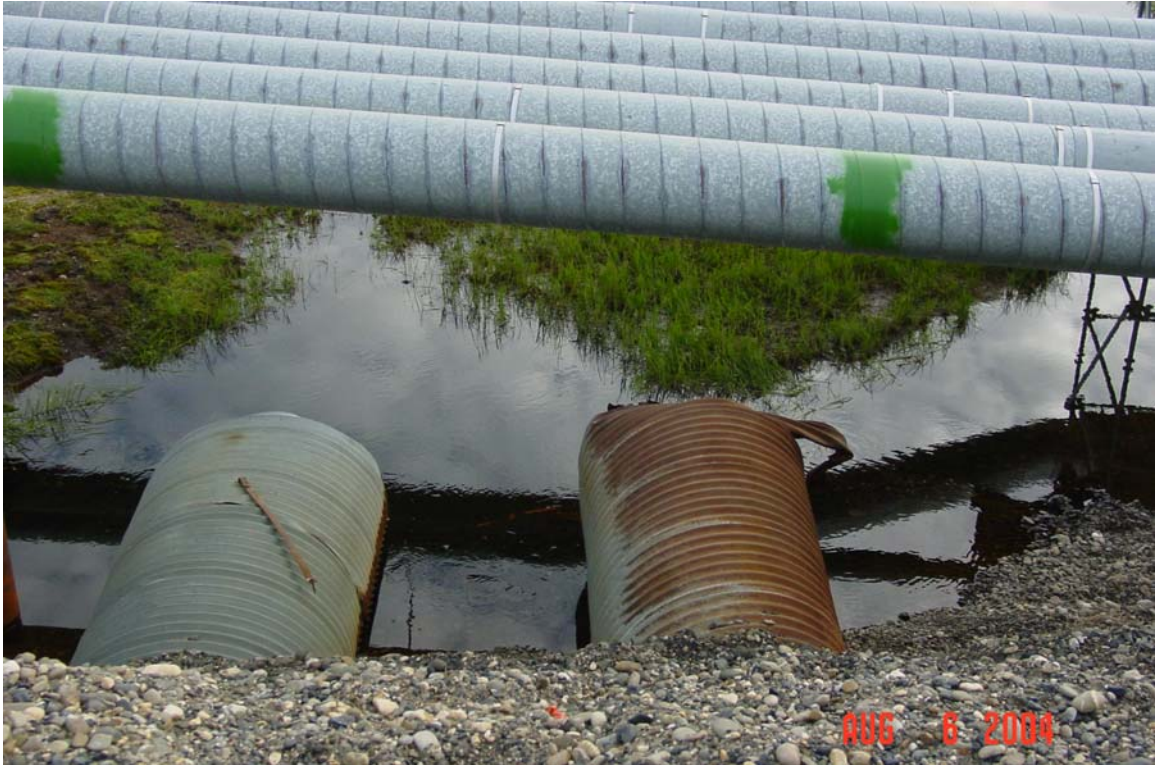
Photograph 133. Misaligned and damaged Leach Creek culvert inlets at the R Pad Road.
