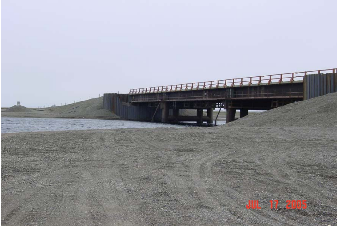
Photograph 185. Kugaruk River Central Channel bridge final repair with sheet pile abutments.
