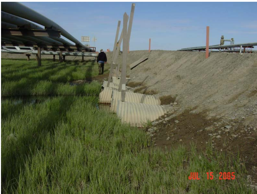
Photograph 253. East Fork Ugnuravik River culvert inlets.
