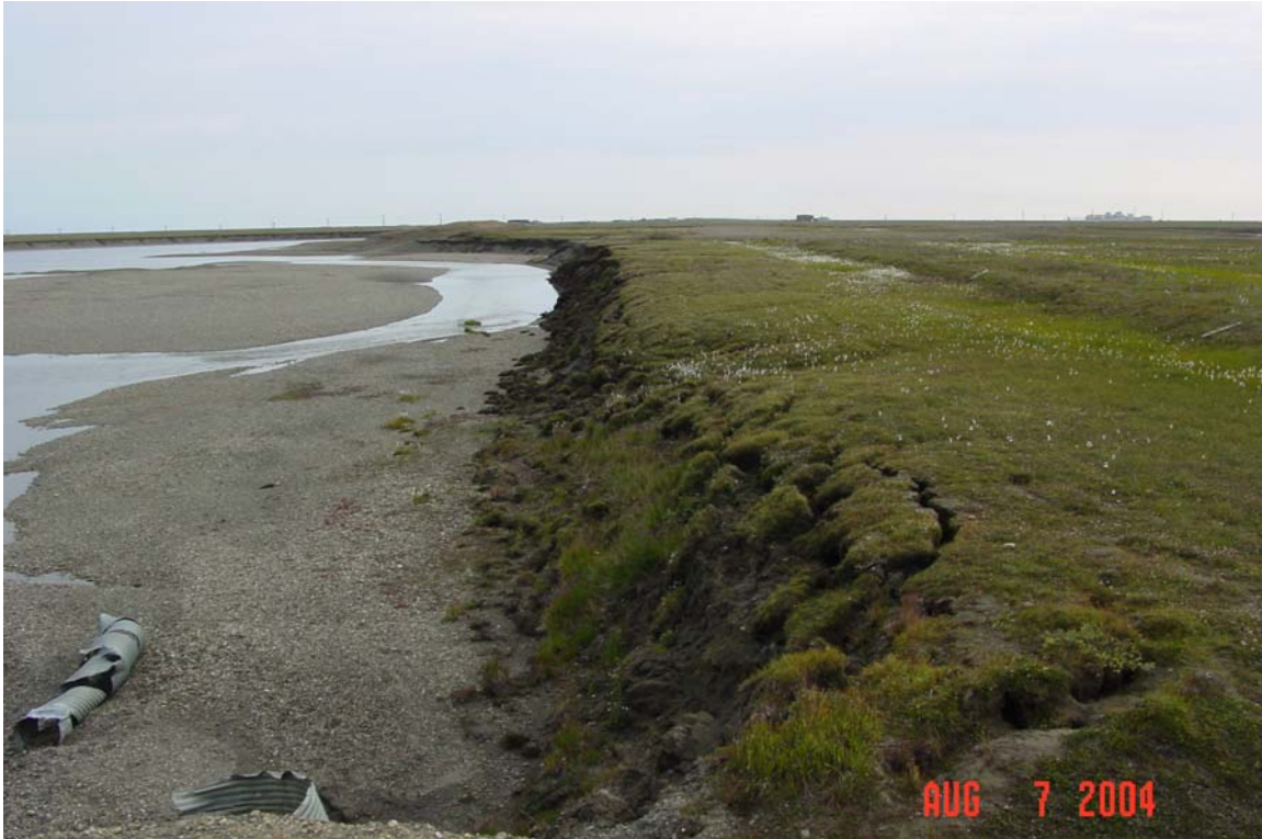
Photograph 61. Putuligayuk River downstream of the Drill Site 15 Road. Actively eroding tundra banks and debris are present on the downstream side of the crossing.
