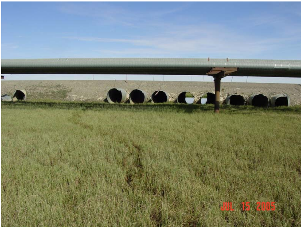
Photograph 240. Main culvert battery inlets of East Fork Central Creek along the Kuparuk Pipeline Road crossing between Drill Site 1C and CPF-1.
