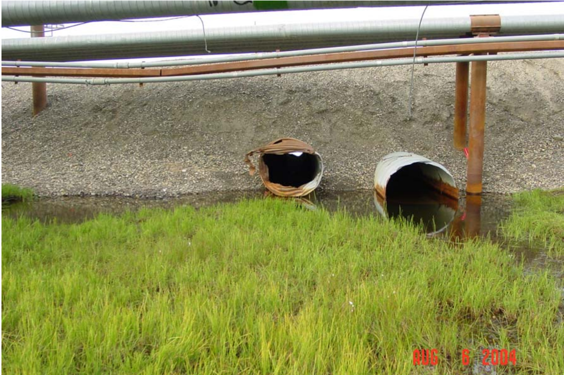
Photograph 135. Leach Creek culvert inlets. Significant damage and culvert misalignment (channel is to the left).
