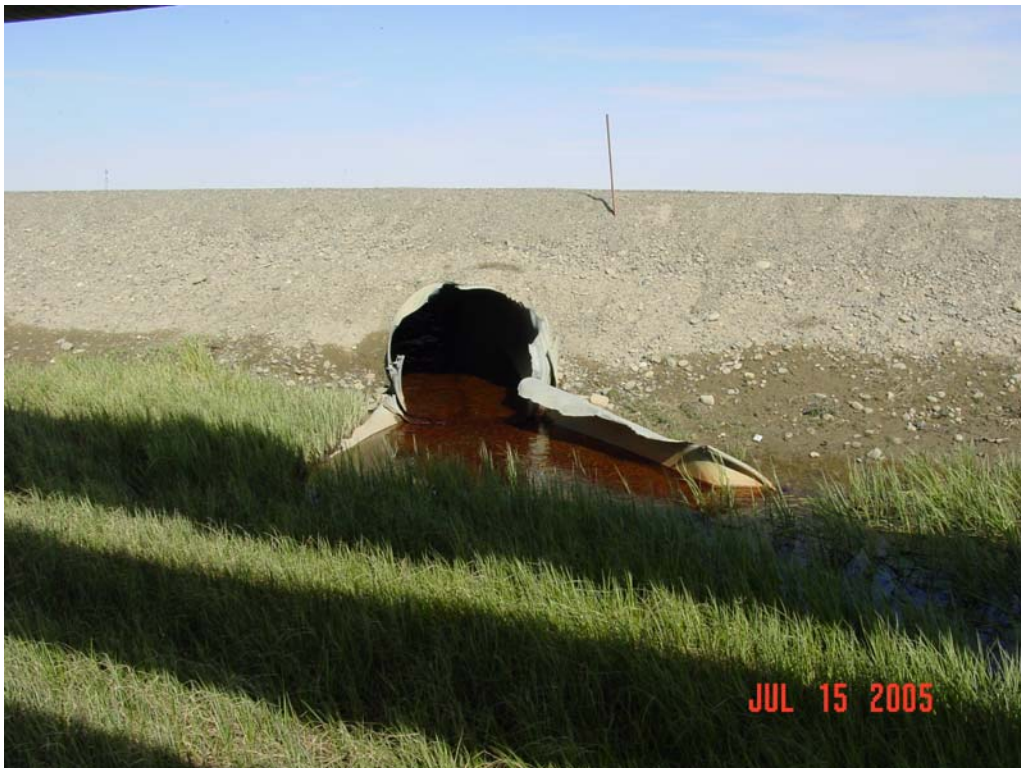
Photograph 244. Damaged culvert apron and inlet.
