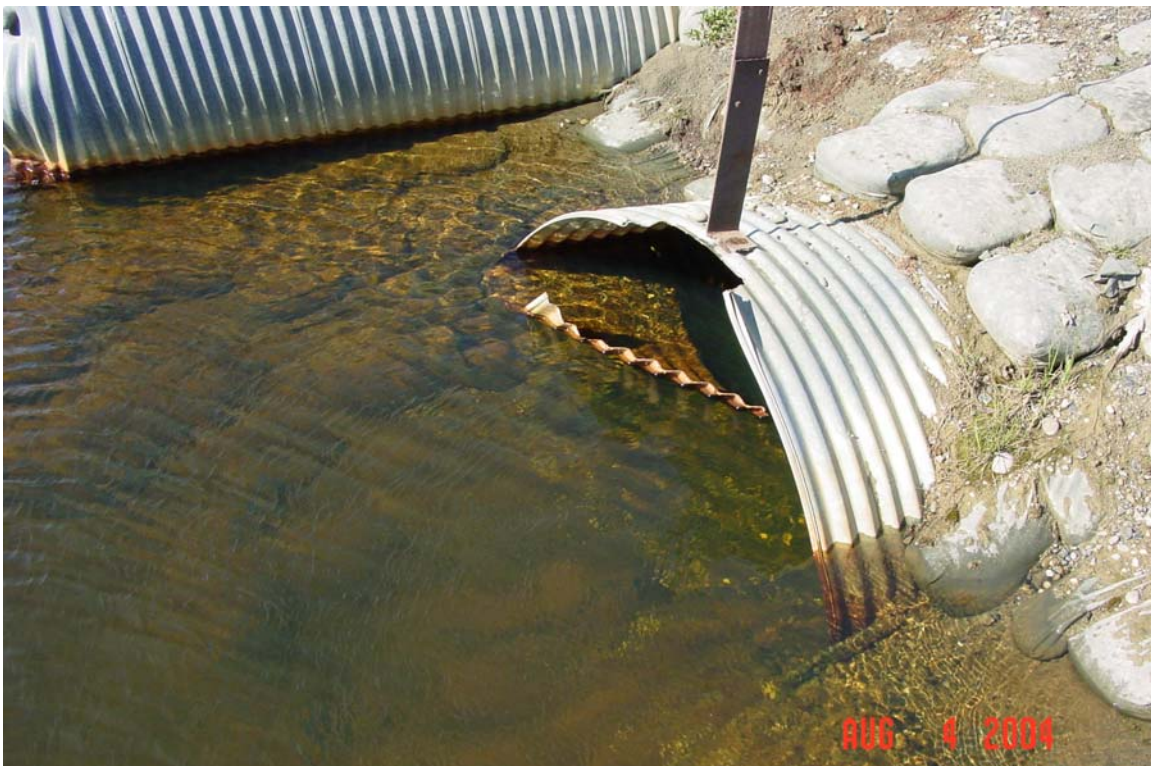
Photograph 303. Kalubik Creek tributary (East Fork Nowhere Creek) culvert inlet bottom upturned and blocking much of the flow through the culvert.
