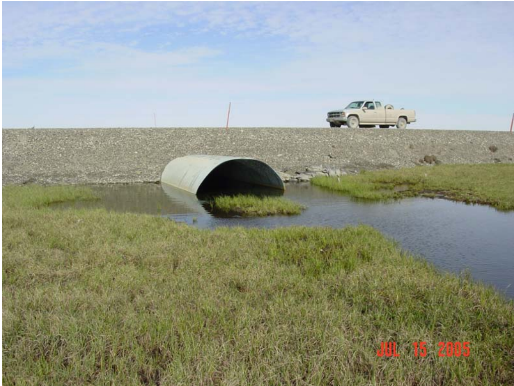
Photograph 193. Milne S Pad Creek culvert inlet.
