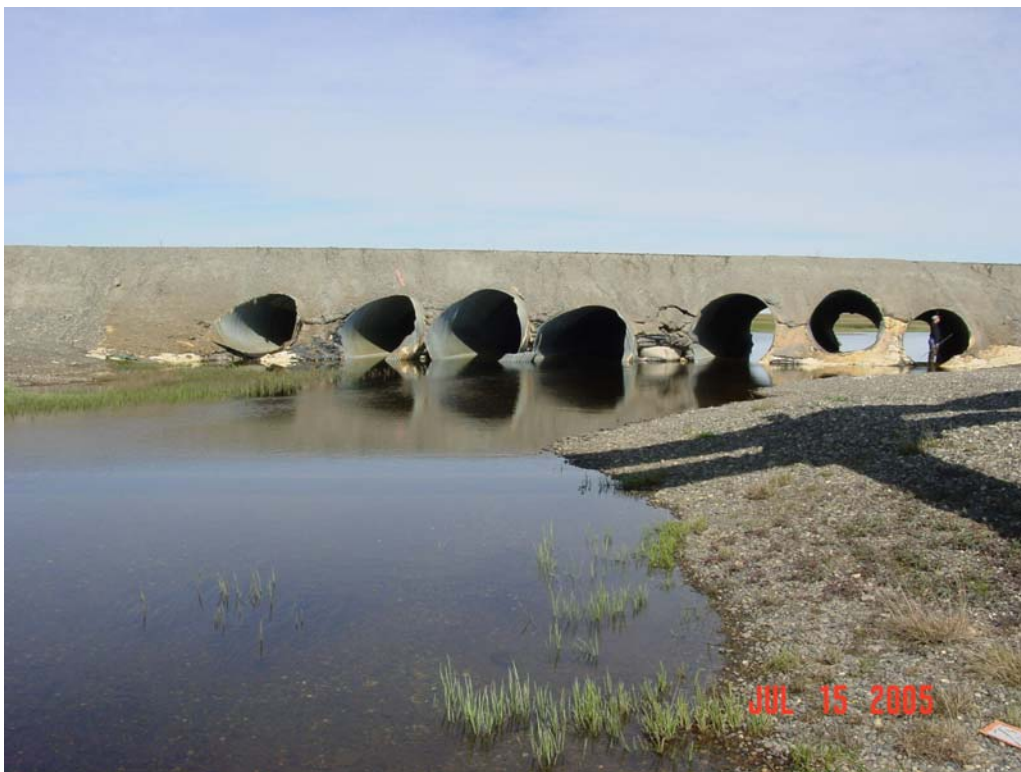
Photograph 217. East Creek culvert inlets with inlet damage, sand bag and road prism erosion and damaged armor overlay.
