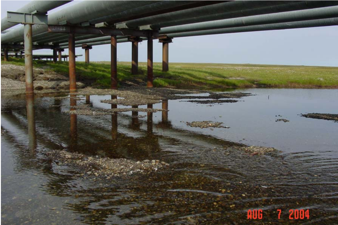
Photograph 104. Little Putuligayuk River old low water crossing. Significant gravel remains in stream channel creating a wide shallow bar across the width of the creek.
