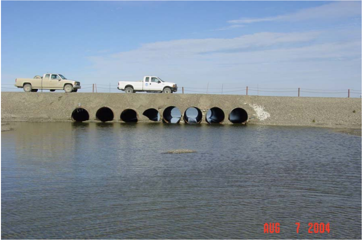
Photograph 3. Sag C Creek culvert inlets.
