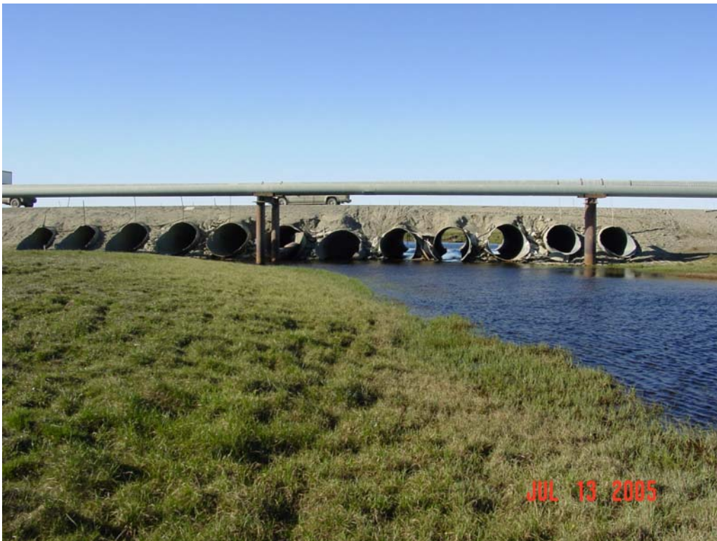
Photograph 141. Road erosion and damaged culvert inlets at the Sakonowiyak River Spine Road crossing.
