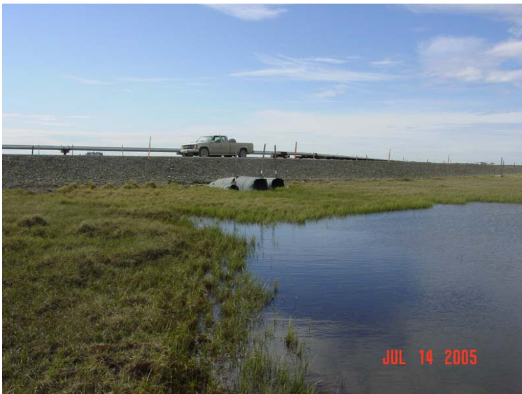
Photograph 336. Ugnuravik River tributary culvert inlets.
