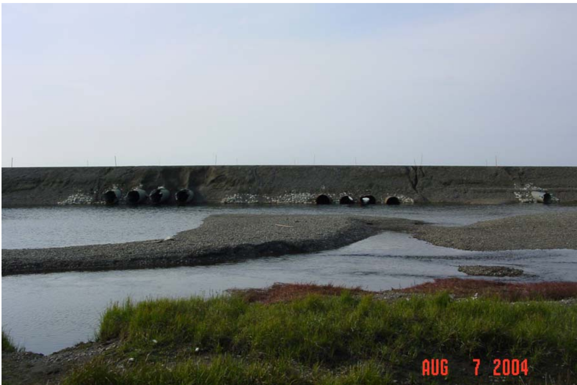
Photograph 97. Little Putuligayuk River culvert outlets, with a massive gravel outwash berm and road erosion.
