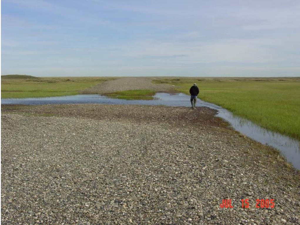
Photograph 170. Pebble Creek flowing over the breached access road.
