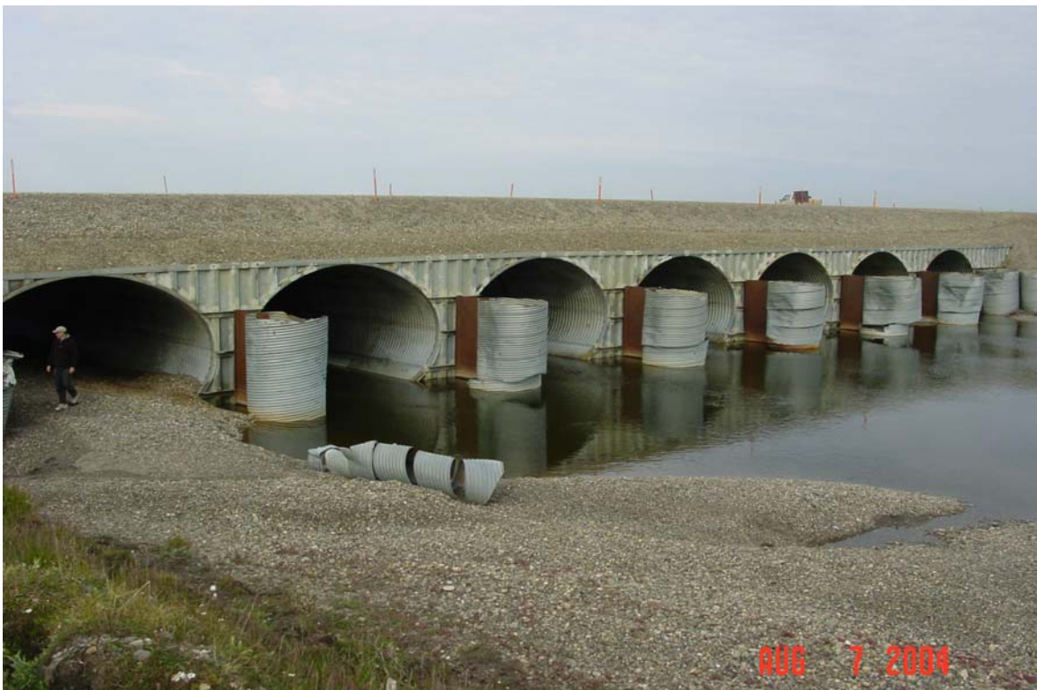
Photograph 62. Putuligayuk River culvert outlets, with gravel outwash, debris and culvert armor damage.
