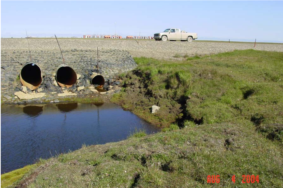
Photograph 309. Tundra erosion on the eastern margin of the Kalubik Creek tributary (Nowhere Creek) culvert battery inlet.
