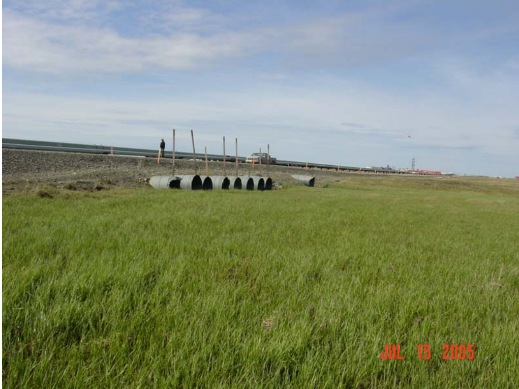
Photograph 239. Main culvert battery outlets of East Fork Central Creek along the Kuparuk Pipeline Road crossing between Drill Site 1C and CPF-1.
