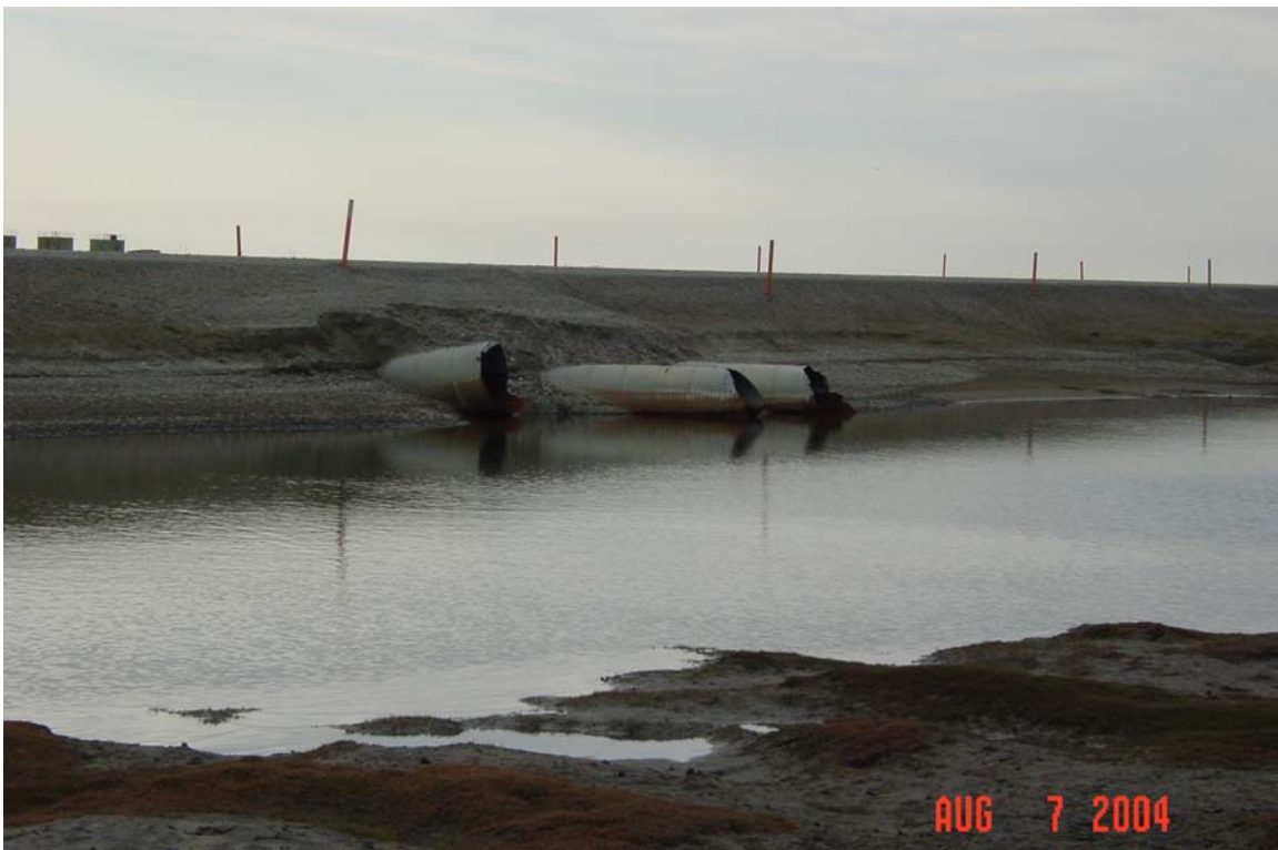
Photograph 58. LGI Estuary Creek culvert inlets. Significant road prism erosion can be seen as well as severe damage to some culverts. High water mark is above pipes.
