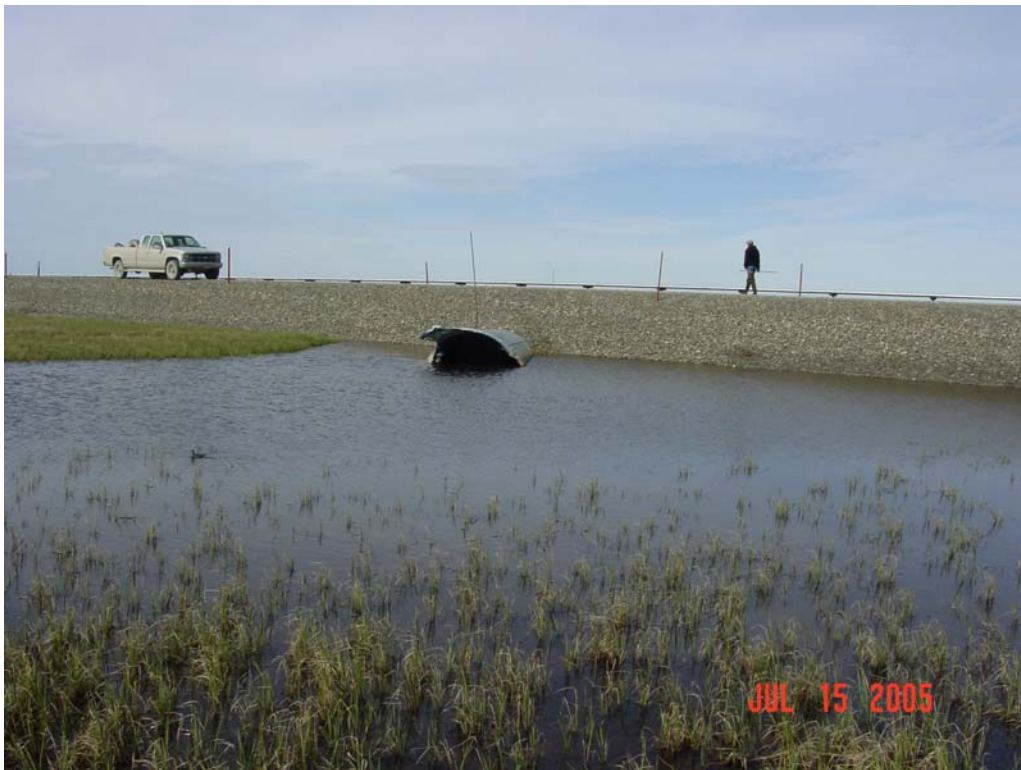
Photograph 196. Damaged Cascade Creek culvert inlet.
