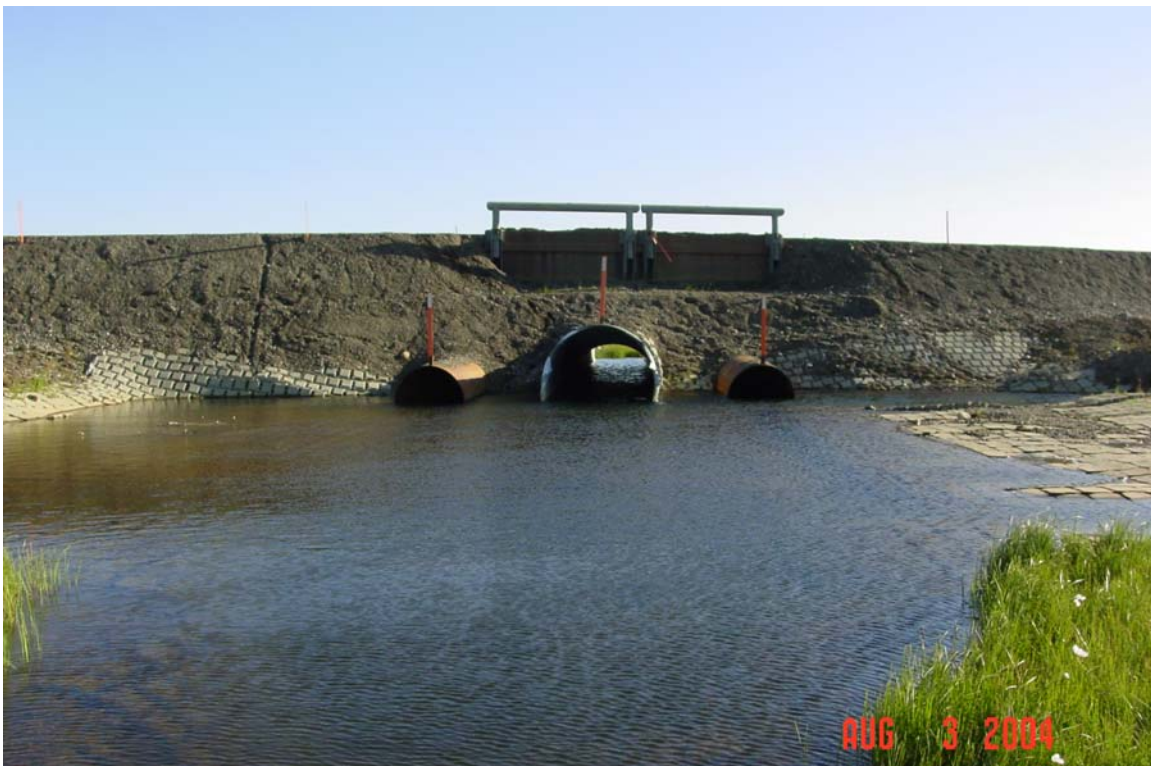
Photograph 404. Culvert outlets at the Miluveach River tributary. Note the extensive gobi mat armor erosion protection and the bridge decking over the partially collapsed 8 foot culvert.
