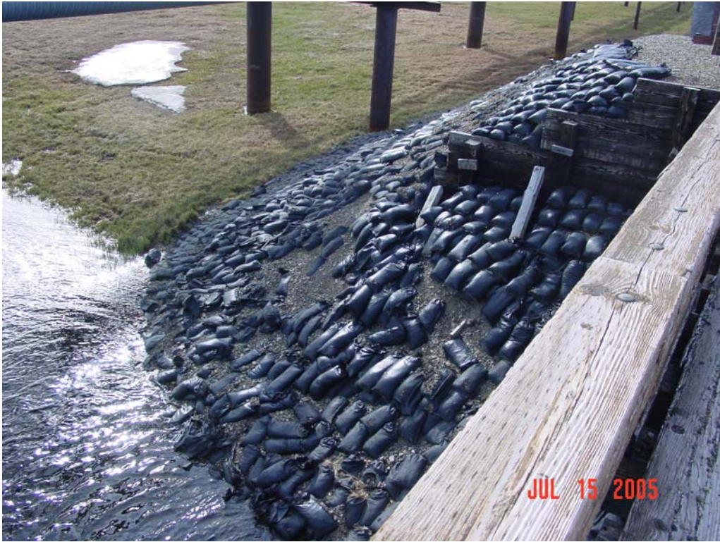
Photograph 169. Sand bag armor erosion on the upstream portion of the west abutment of the Pebble Creek bridge.
