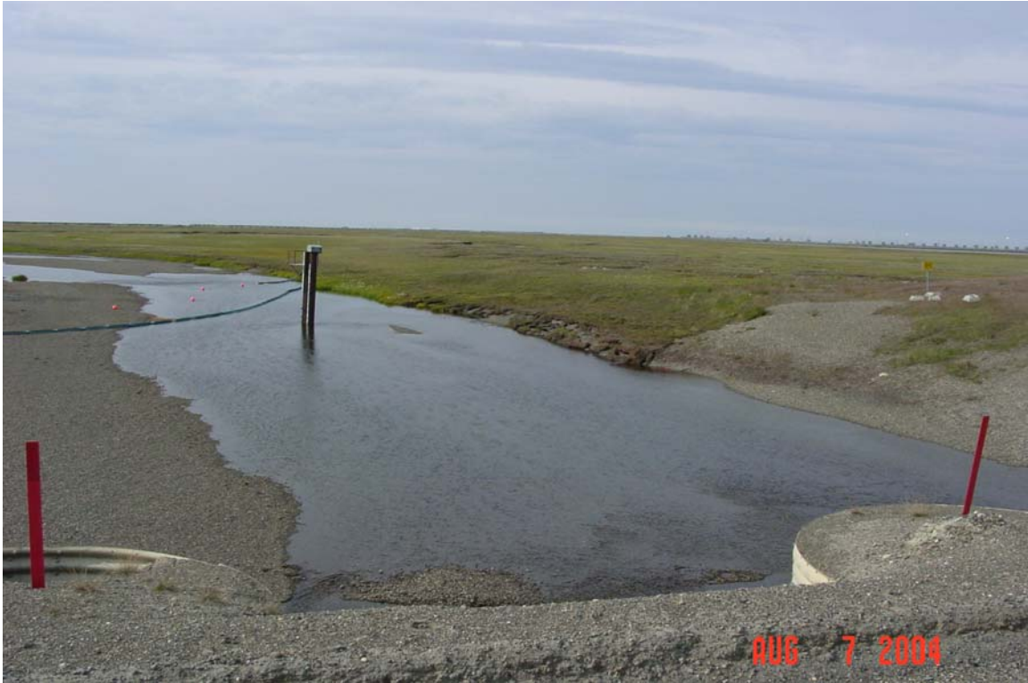
Photograph 68. Putuligayuk River upstream of the Spine Road Crossing. Upstream gravel deposition (accretion) can be observed as well as some tundra erosion.
