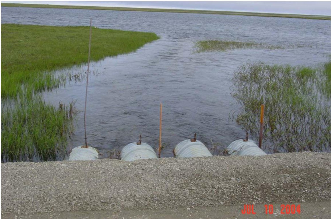
Photograph 119. Fawn Creek culvert outlets downstream of the F-Pad to E-Pad Road.
