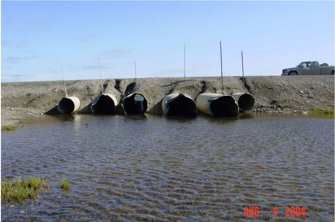
Photograph 292. West Fork Ugnuravik River culvert inlet damage, road prism erosion, and a high water mark about 1 foot above the inlets.
