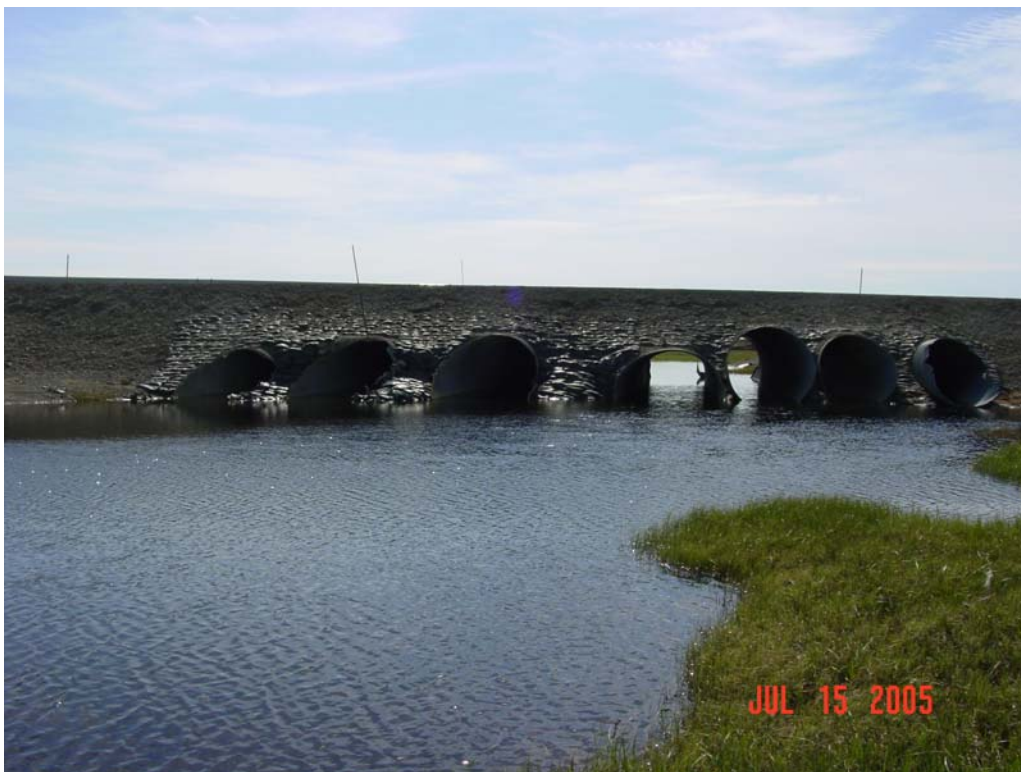
Photograph 219. East Creek culvert outlets with sand bag armor.
