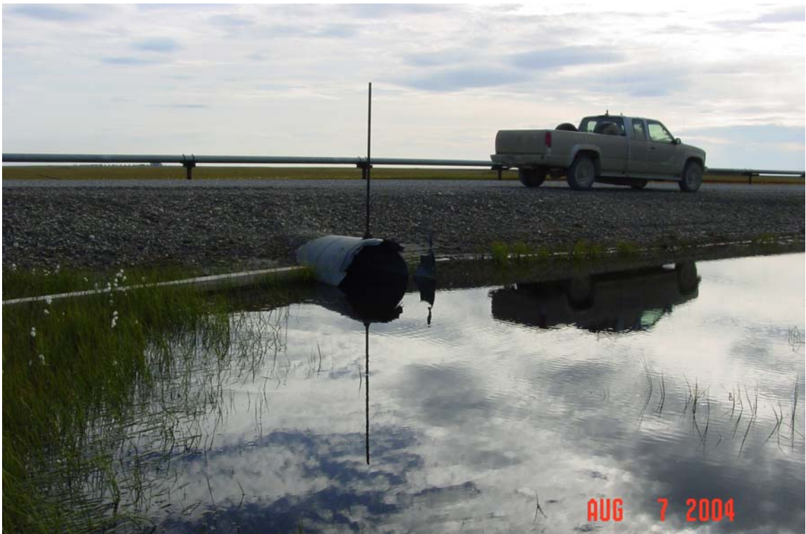
Photograph 11. Duck Island Creek culvert outlet.
