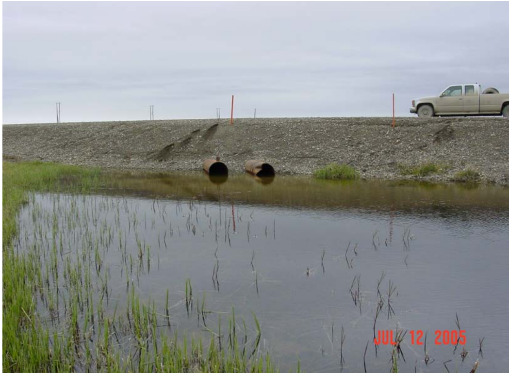
Photograph 27. Washout Creek Tributary culvert inlets. Damage to one of the inlet pipes can be seen as well as high water mark above pipes.
