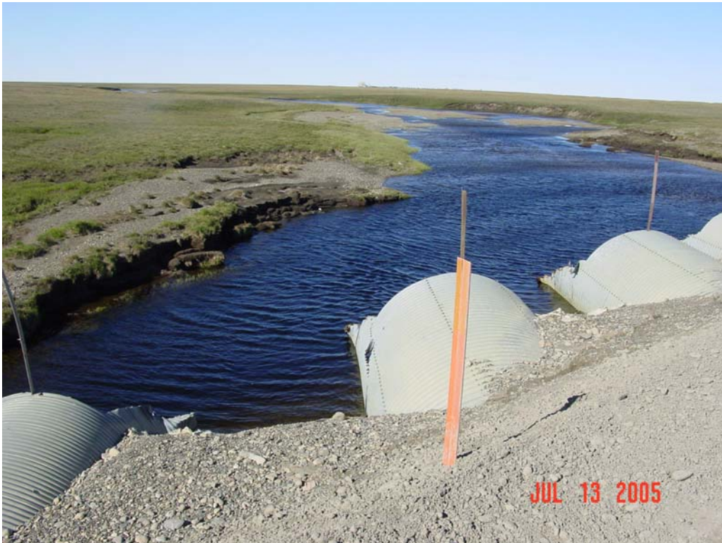
Photograph 145. Smith Creek downstream of the Spine Road. Damage to outlets, outlet scour, bank erosion and significant gravel outwash can be seen.
