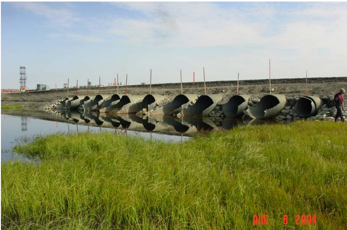
Photograph 260. Ugnuravik River culvert outlets at the Spine Road crossing.
