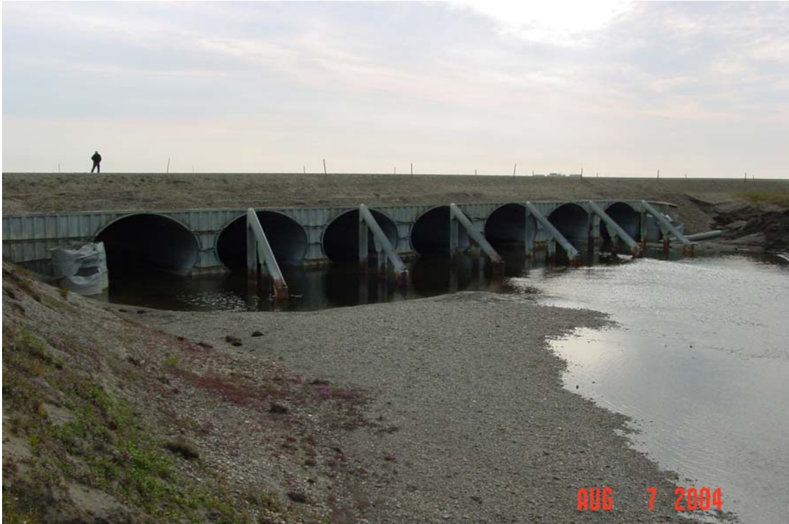
Photograph 63. Putuligayuk River culvert inlets at the Drill Site 15 road. Damage to armor, bank erosion, and gravel deposition from scour can be seen. A washed out culvert can also be observed in the stream channel.
