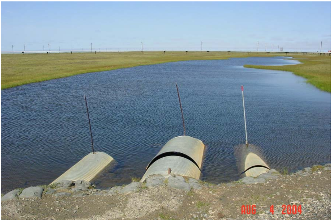
Photograph 297. Caribou Creek downstream of the access road at Drill Site 3B. Broken outlets.
