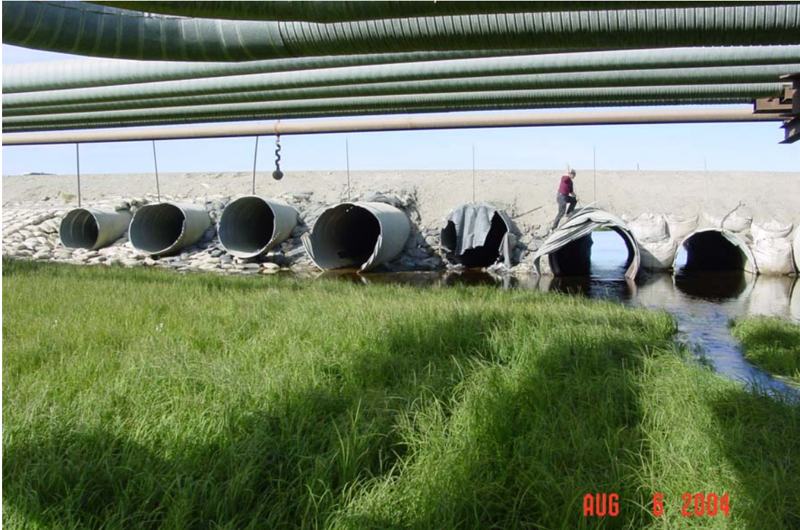
Photograph 257. The western half of the Ugnuravik River culvert battery inlets.
