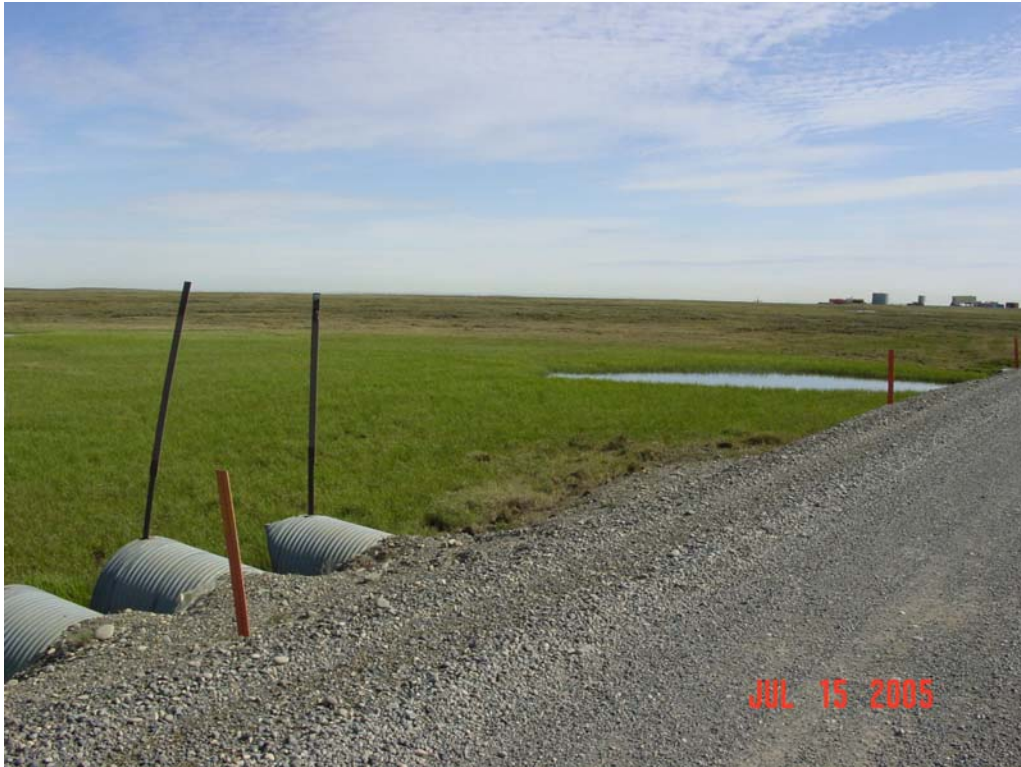
Photograph 241. Main battery outlets and scour pool of the single culvert carrying all of the creek flow.
