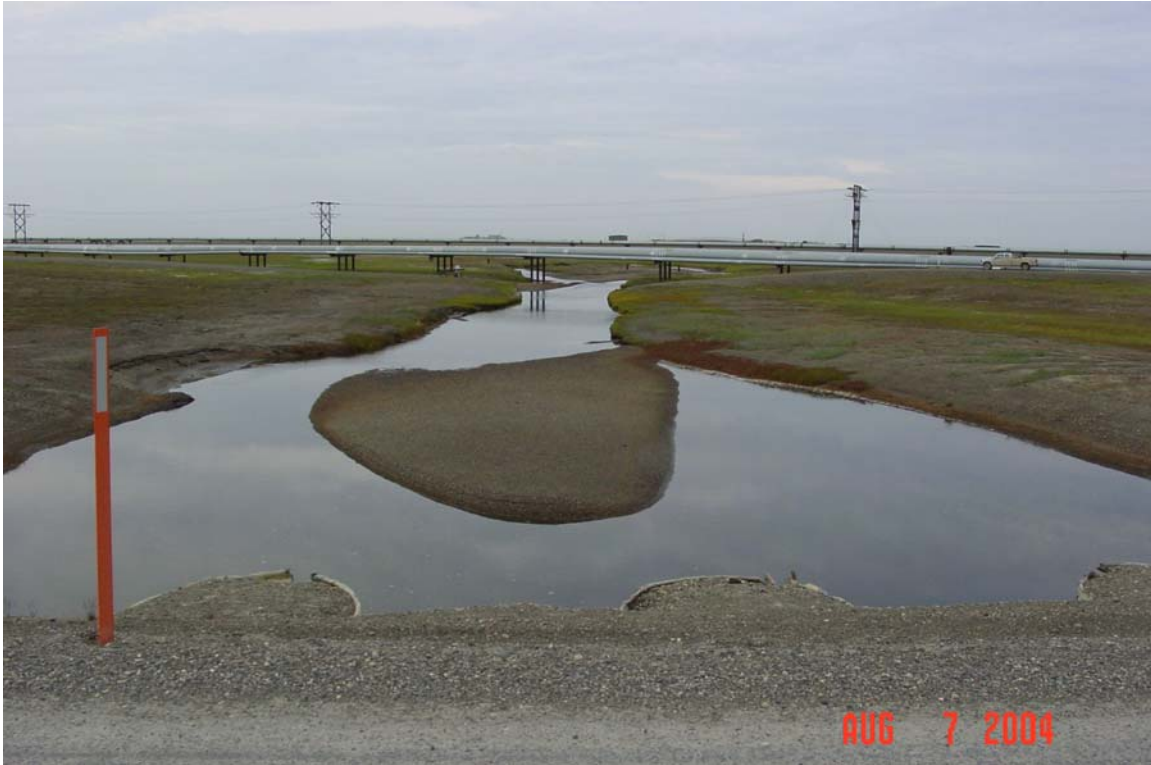
Photograph 82. The Little Putuligayuk River upstream of the West Dock Road. A large gravel bar has formed upstream of the culverts. Bank erosion is evident.
