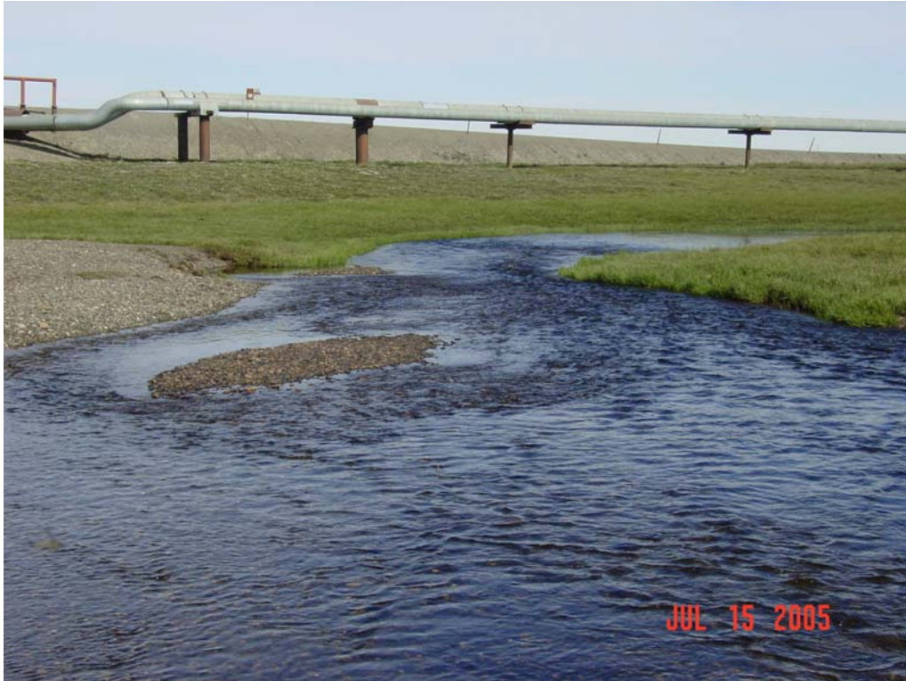
Photograph 222. Gravel deposition downstream of the MP-1 crossing.
