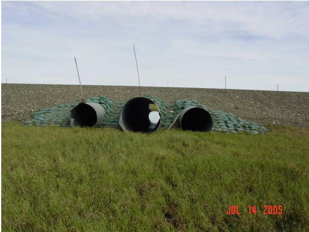
Photograph 327. Ugnuravik River tributary culvert inlets.
