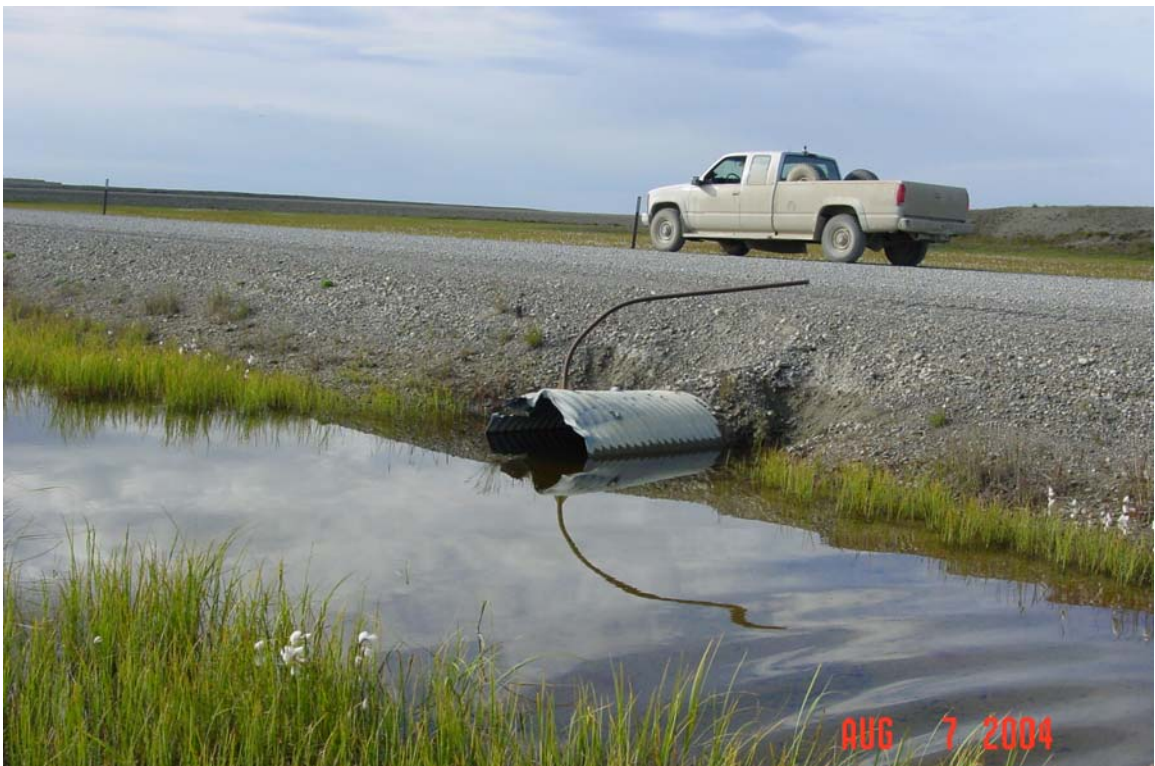
Photograph 9. Duck Island Creek culvert inlet. Note minor road prism erosion and high-water mark above culvert.
