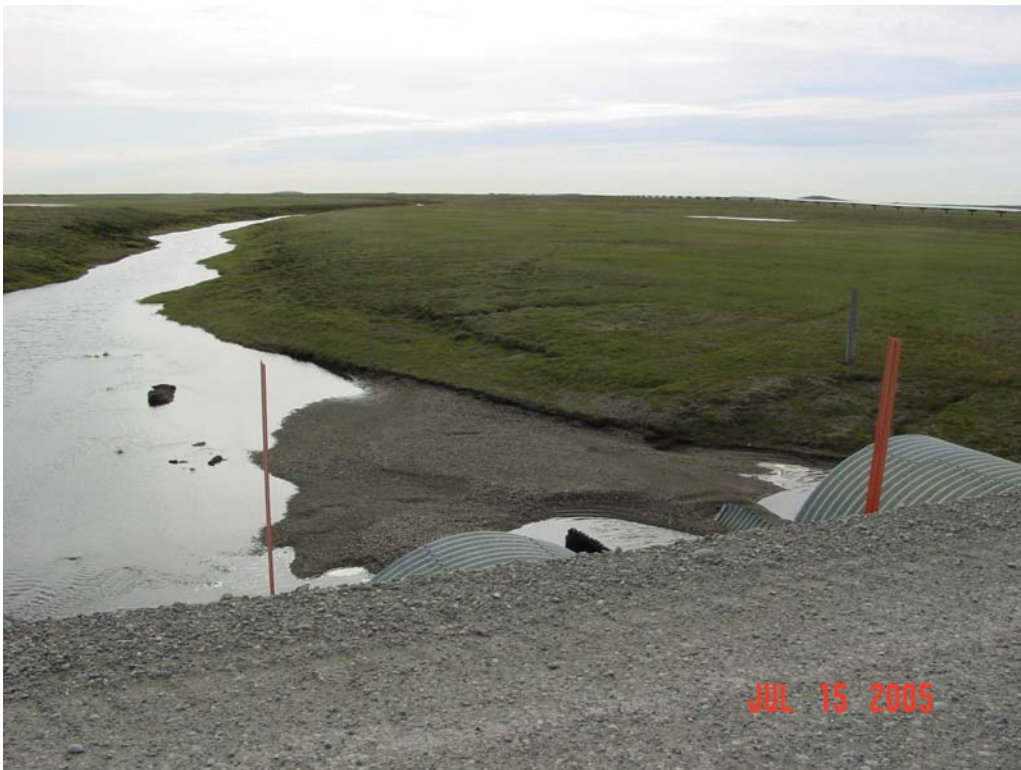
Photograph 158. Smith Creek upstream of the W Pad access road. Gravel deposition at culvert inlets.
