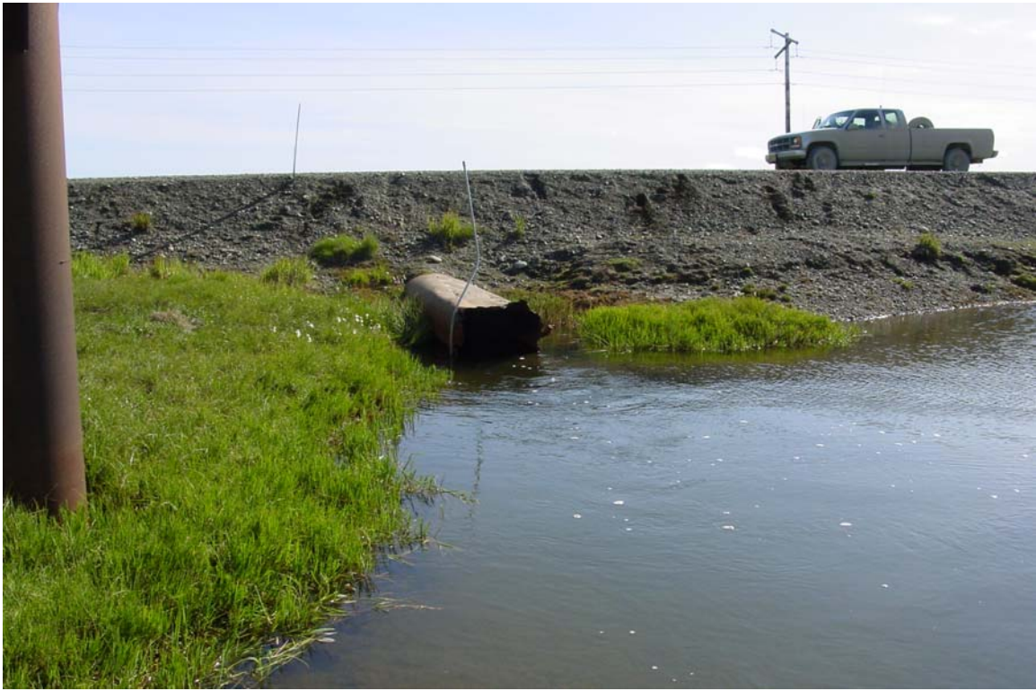
Photograph 215. Milne B Pad Creek flattened culvert outlet.
