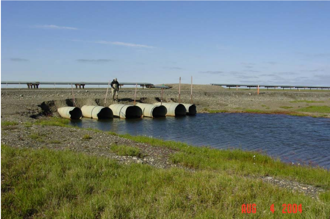
Photograph 294. West Fork Ugnuravik River culvert outlets with substantial road prism erosion and outwash gravels.
