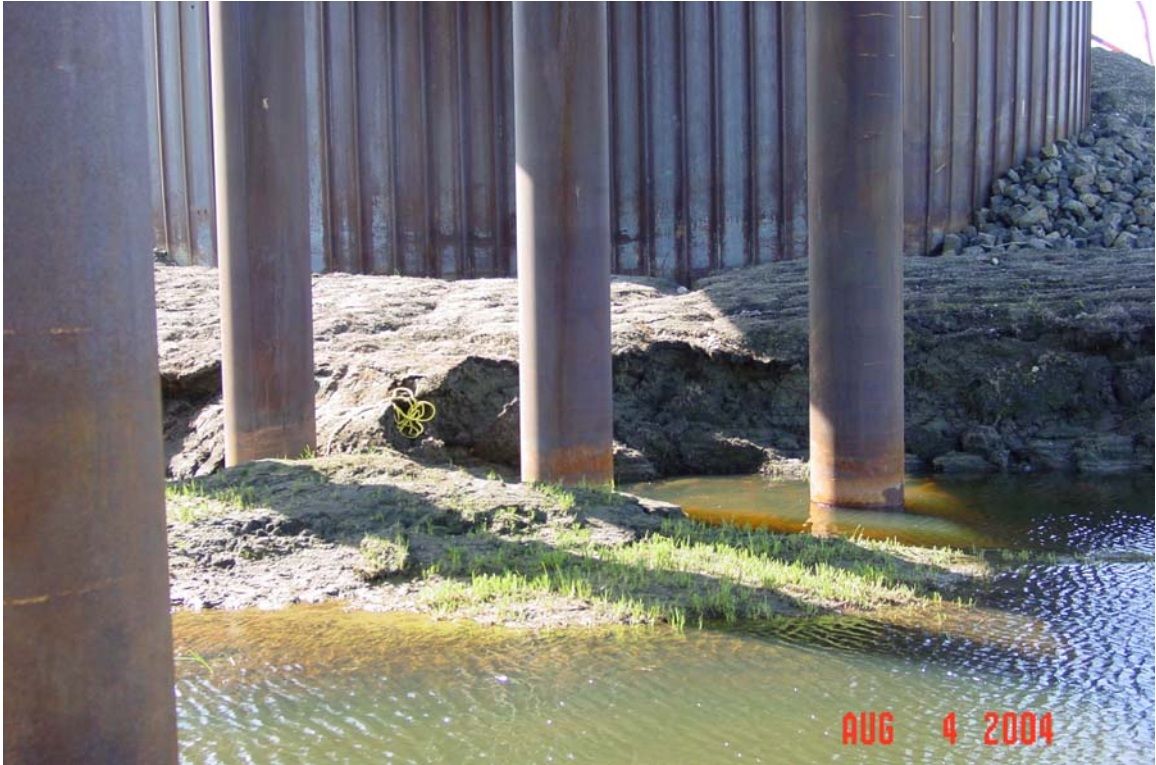
Photograph 319. Scour around the western bridge piers.
