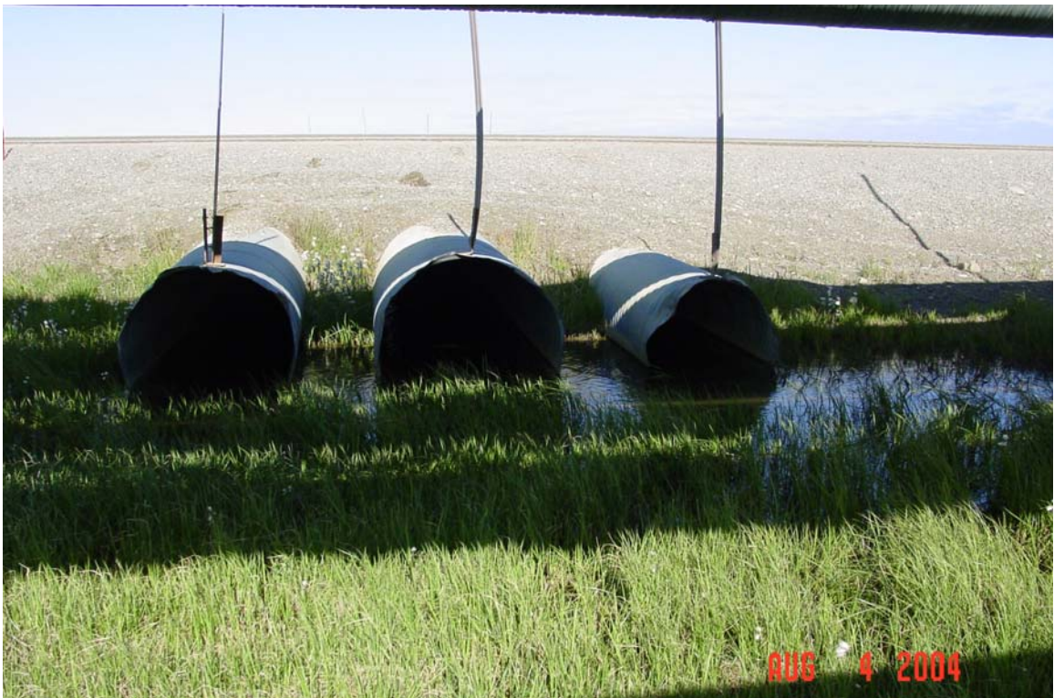
Photograph 355. Charlie Creek culvert inlets.
