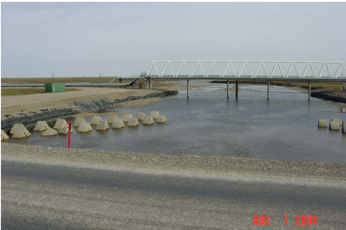
Photograph 69. Putuligayuk River downstream of the Spine Road crossing. Wide Gobi mat apron, Dragon's Teeth, gabion baskets, failing erosion protection and gravel outwash can be seen.
