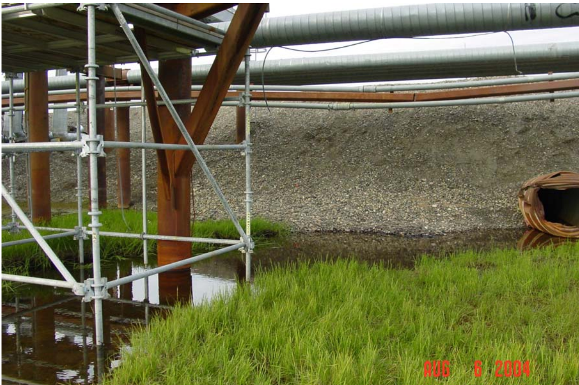
Photograph 136. Leach Creek culvert inlets. Highwater mark is above the culverts. Scaffolding is erected in stream channel, no active work appeared to be occurring.
