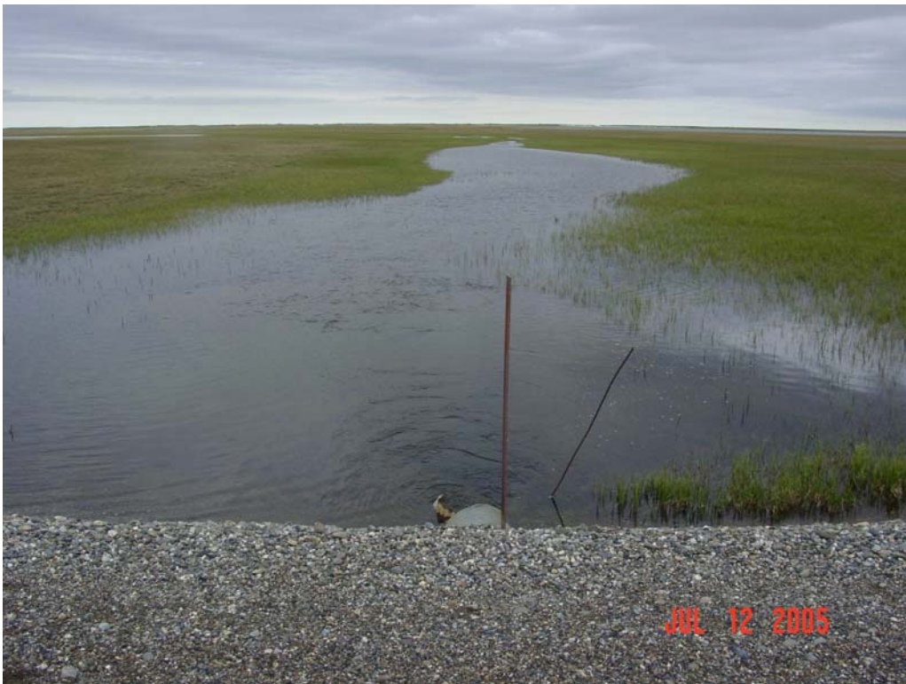
Photograph 42. Unnamed Drill Site 16 Creek downstream of the road. Damage to culvert outlet can be observed. Significant flow was present in this creek at the time of inspection
