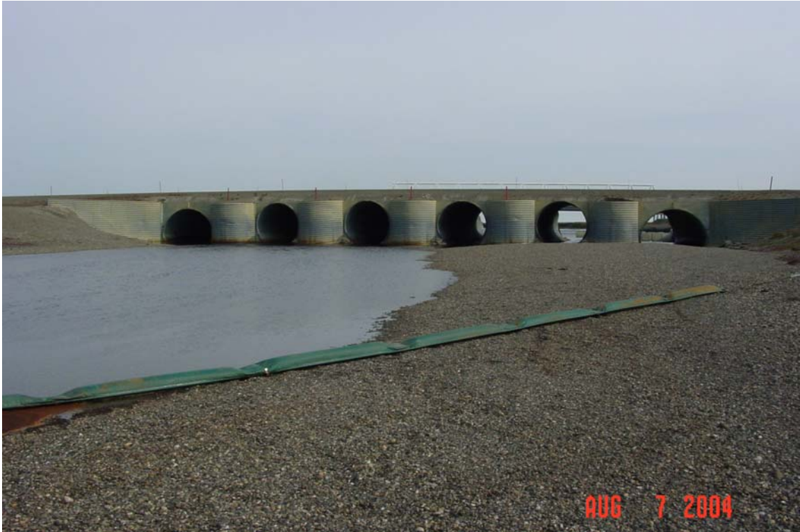
Photograph 70. Putuligayuk River culvert inlets at the Spine Road. Gravel deposition can be observed.
