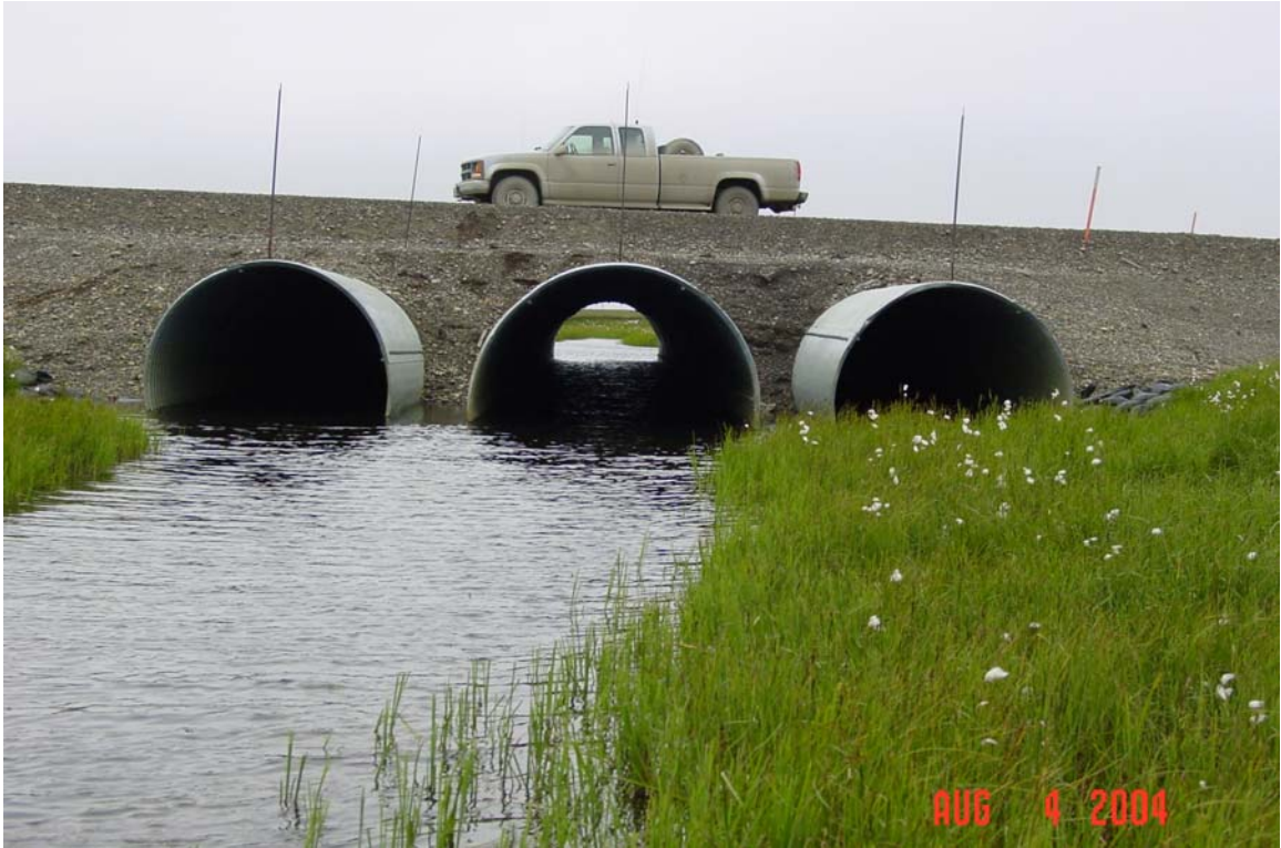
Photograph 391. West Fork Kalubik Creek culvert outlets.
