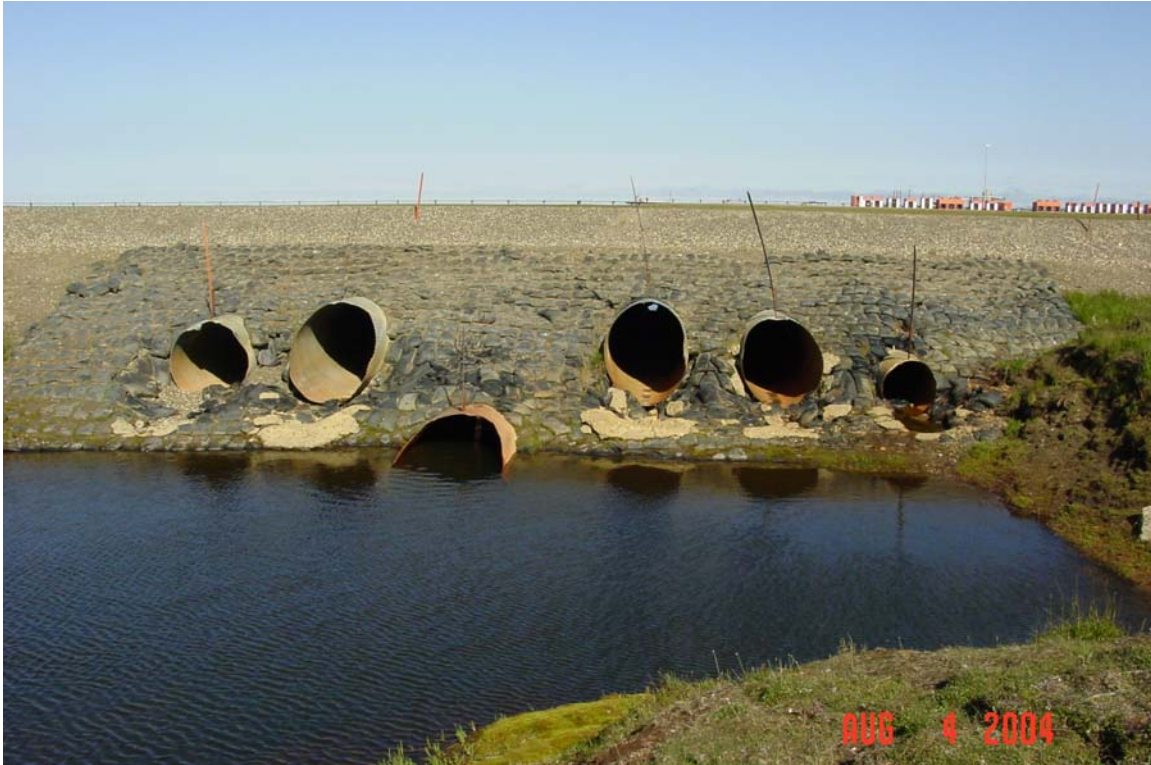
Photograph 307. Kalubik Creek tributary (Nowhere Creek) culvert inlets with partial concrete aprons, missing sand bag armor, and a high water mark about 2 feet above the inlets.
