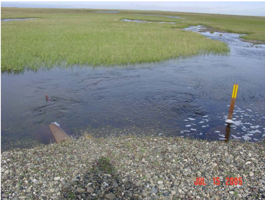
Photograph 175. Submerged Pebble Creek culvert outlets.
