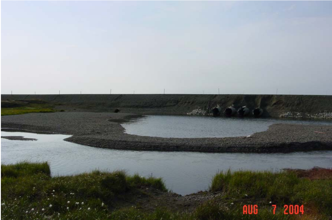
Photograph 98. Little Putuligayuk River culvert outlets, with a massive gravel outwash berm and road erosion.
