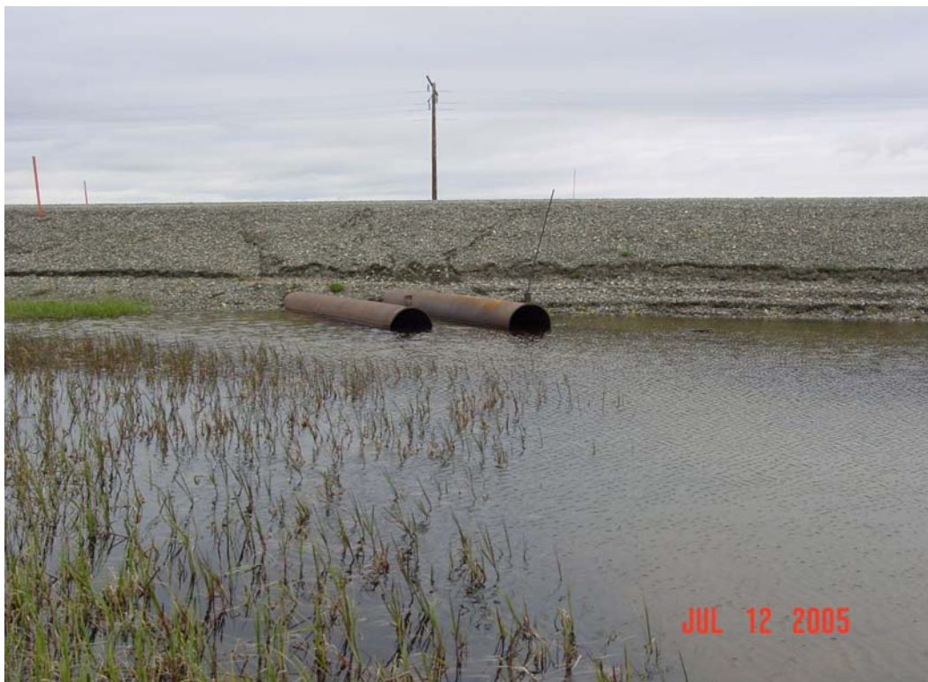
Photograph 28. Washout Creek Tributary culvert outlets. Note highwater marks above or at top of pipe elevation.
