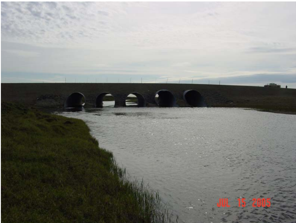
Photograph 162. Smith Creek culvert outlets.
