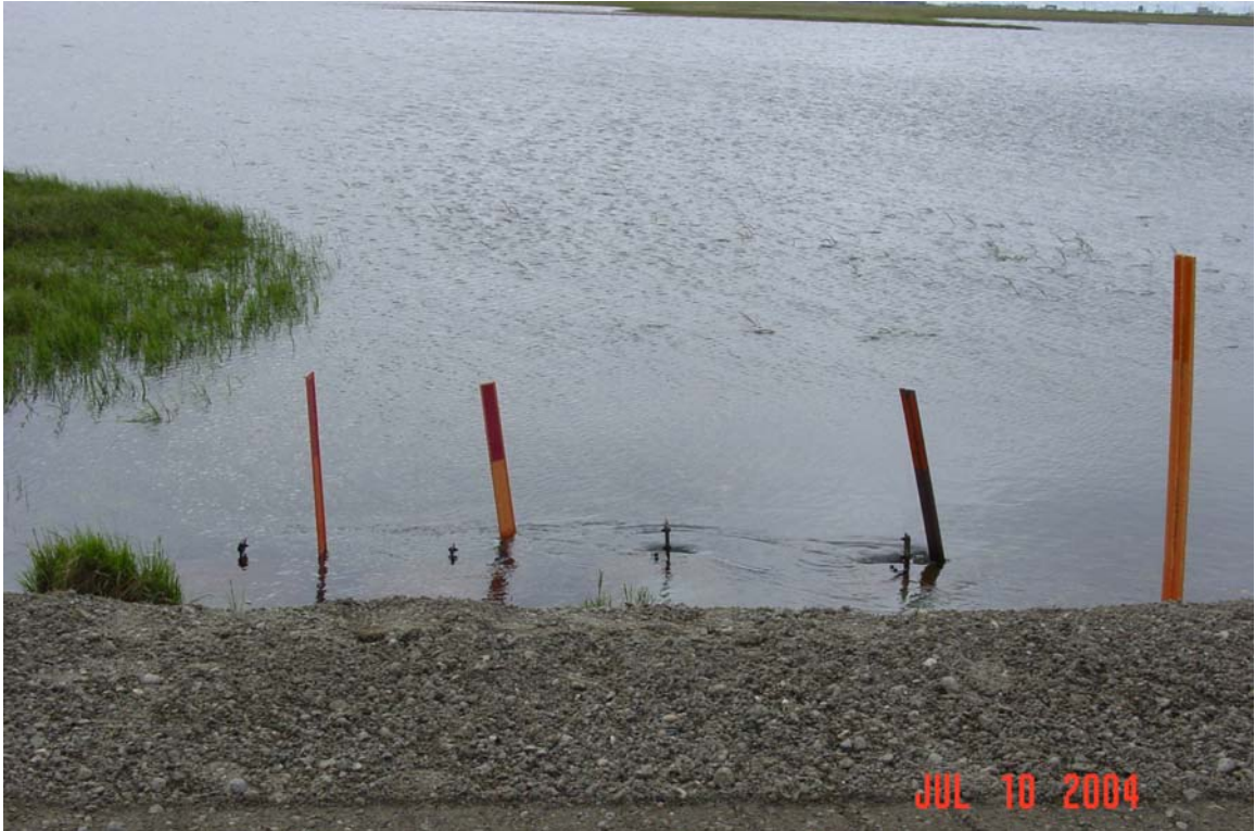
Photograph 118. Fawn Creek upstream of the F-Pad to E-Pad Road. Water is ponded upstream and culverts are submerged; whirlpools at inlets indicate excessive velocity is likely.
