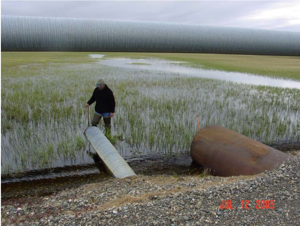
Photograph 46. Significant ponding of the Unnamed Drill Site 16 Creek upstream of the work pad crossing.
