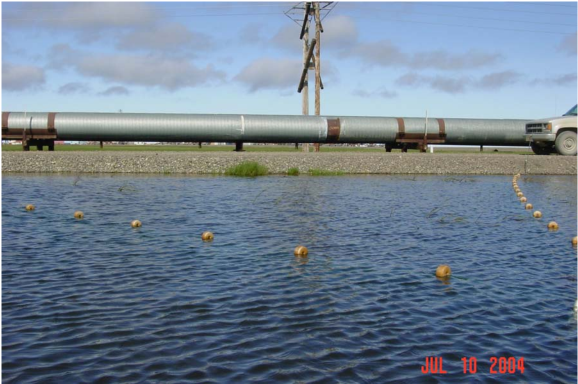
Photograph 108. Fawn Creek looking at upstream side of crossing; culvert is submerged.
