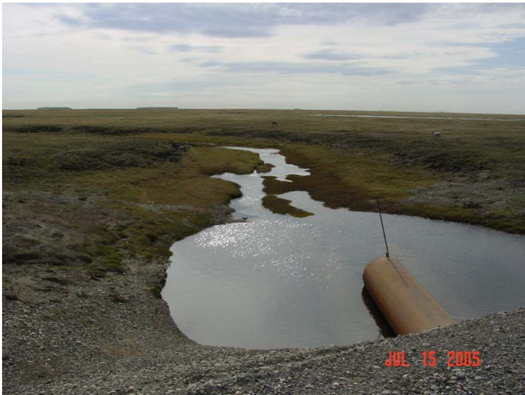
Photograph 210. No Point Creek upstream of the Milne Point F Pad road. Note the two submerged excessively long pipes.
