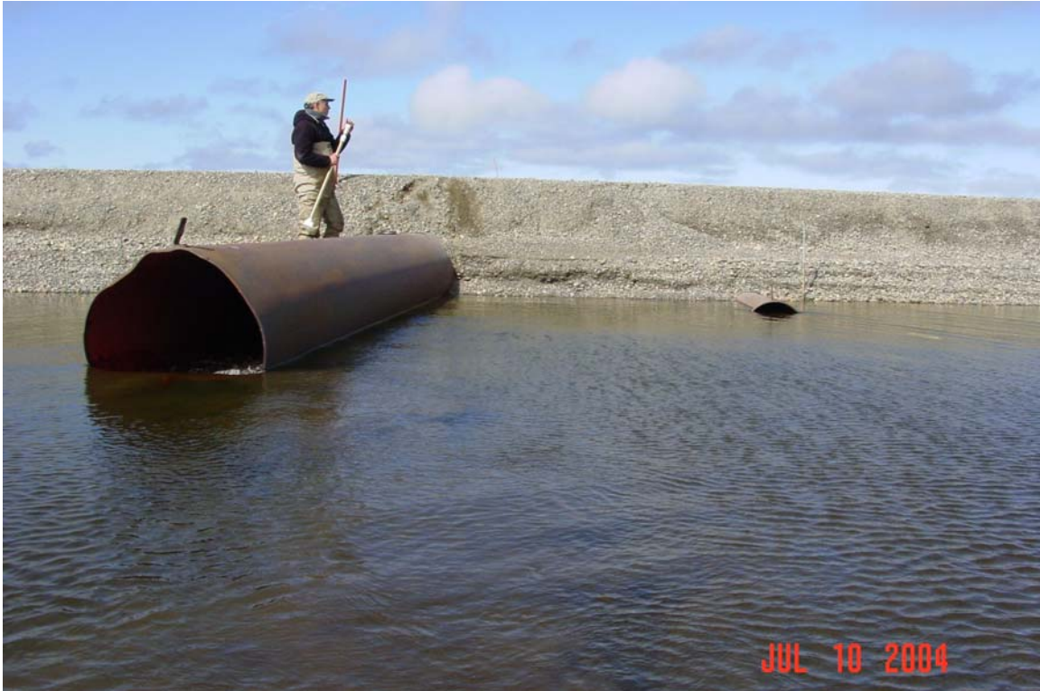
Photograph 112. Fawn Creek culvert inlets. The highwater mark can be seen above the pipes as well as road bed erosion. Water velocity is increased as it passes into the undersized culverts. Note the hydraulic drop into the large pipe.
