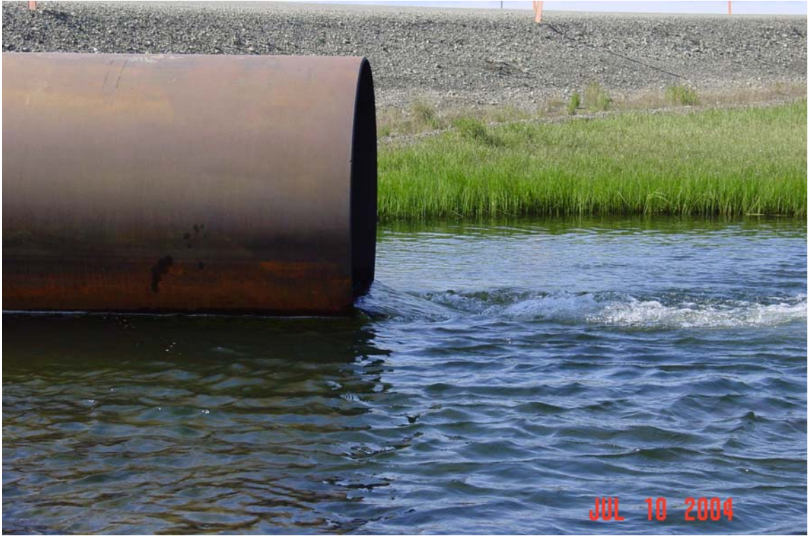
Photograph 126. Fawn Creek culvert outlet. Culvert outlet is slightly perched creating a barrier to passage at most flows for most fish species identified using the system.
