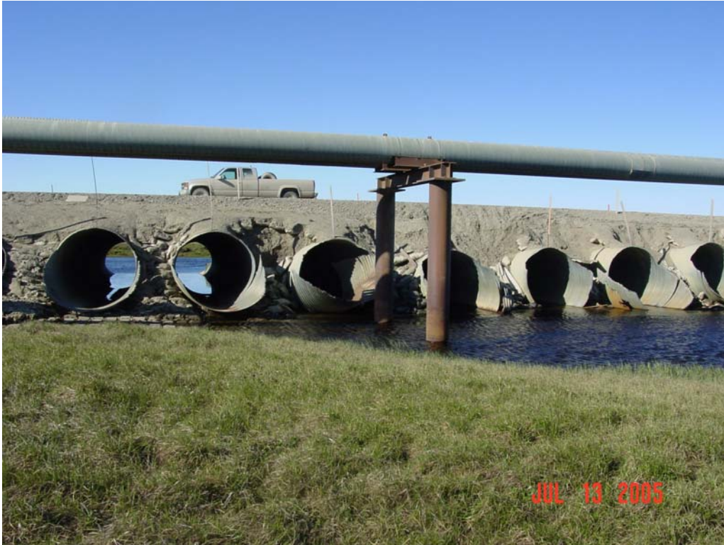
Photograph 142. Road erosion and damaged culvert inlets at the Spine Road crossing of the Sakonowak River.
