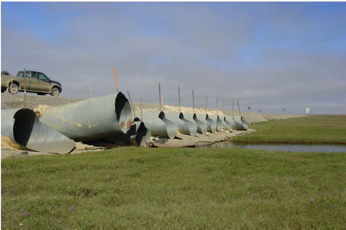
Photograph 385. Culvert inlets at the Kalubik Creek Spine Road crossing, July 8, 2007.
