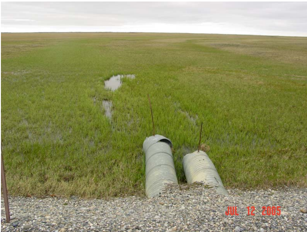
Photograph 38. Unnamed Drill Site 16 Creek downstream of road. Damaged culvert outlets.
