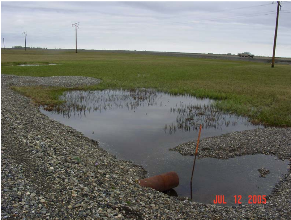
Photograph 49. Unnamed Drill Site 16 Creek downstream of the work pad crossing. The 36 inch culvert is located just in the foreground of the ponded water in the top left of the picture.
