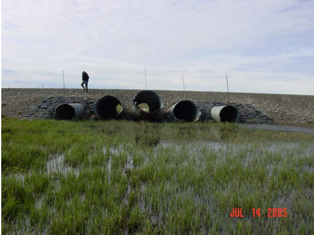
Photograph 371. Kalubik Creek tributary bowed and perched culvert inlets, coupled with perched outlets, block fish passage.
