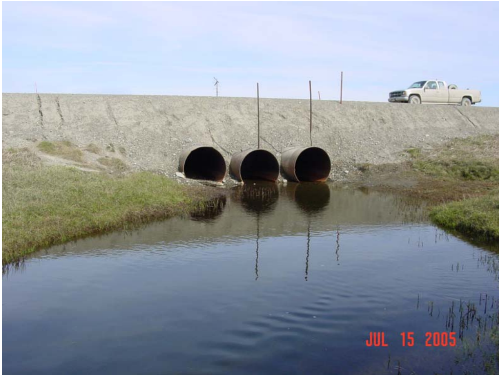
Photograph 207. Lower West Central Creek culvert inlets.
