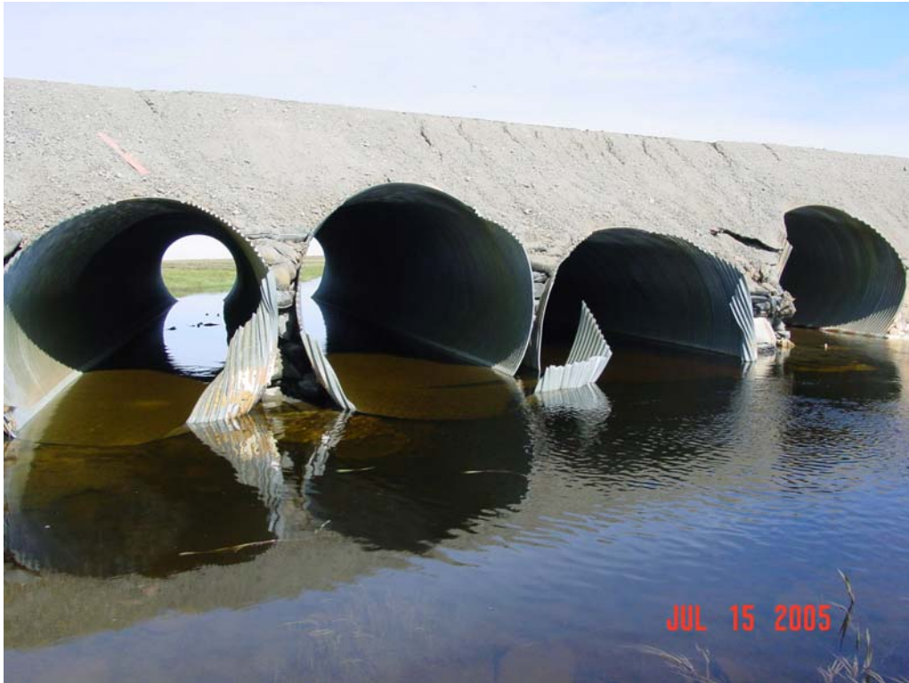
Photograph 218. East Creek culvert inlets with substantial damage.
