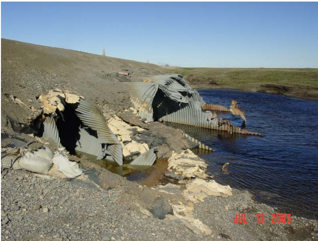
Photograph 147. Smith Creek at the Spine Road crossing. Severe damage to culvert inlets, significant road and armor erosion, and upstream scour.
