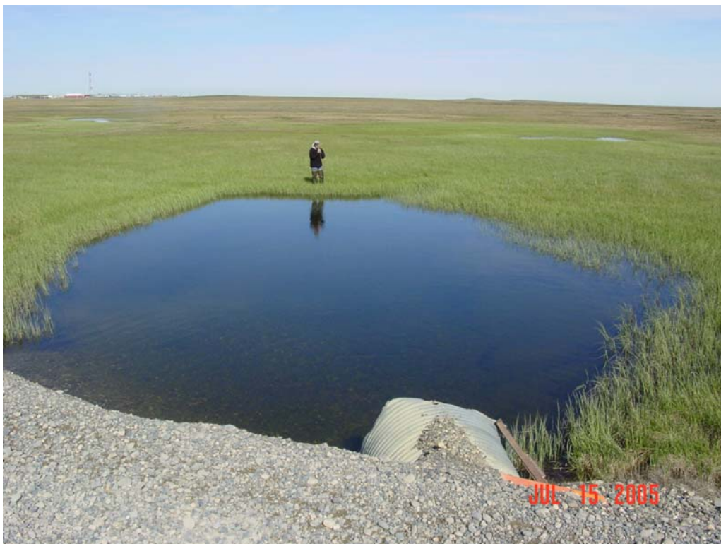
Photograph 242. Five to six foot deep scour pool at the outlet of the culvert carrying all of the creek flow.
