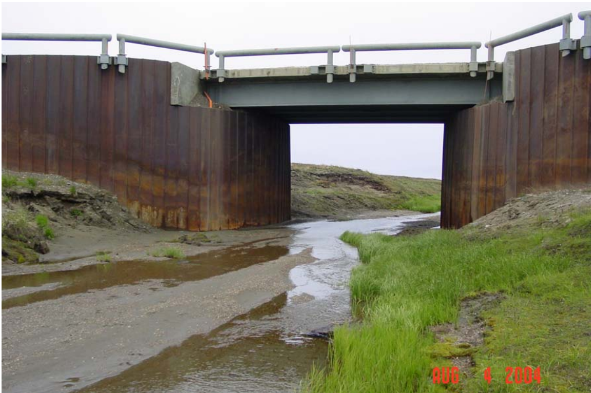
Photograph 396. The Trouble Creek bridge viewed from upstream. Note the bank erosion upstream of the west abutment.
