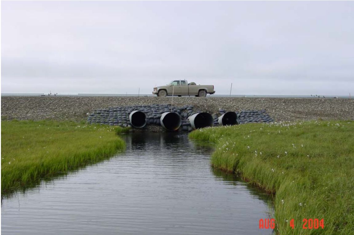
Photograph 360. West Fork Ugnuravik River culvert outlets.
