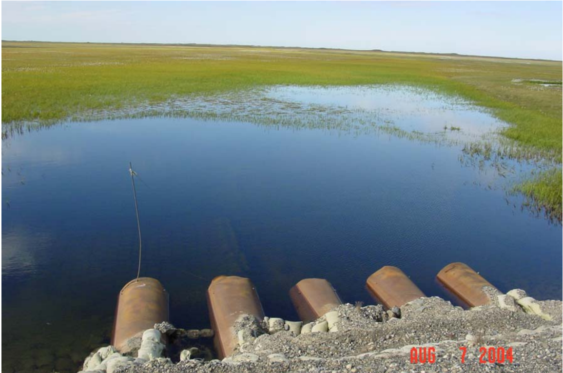
Photograph 16. North Fork Endicott Creek downstream of road, with sand bag armor and road prism erosion.
