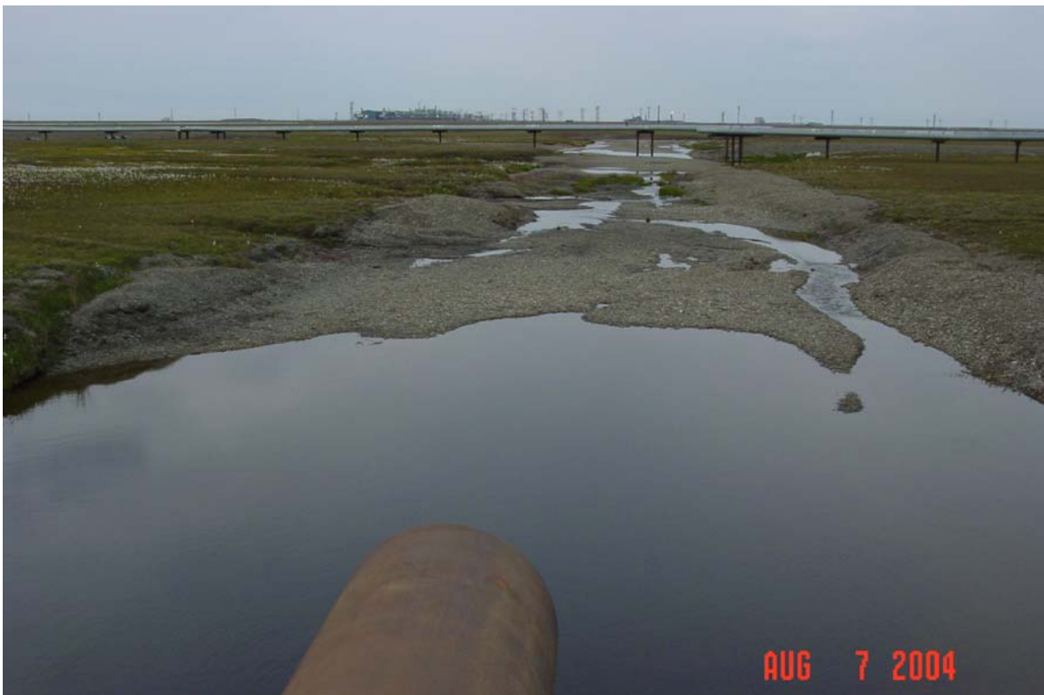
Photograph 81. Pump 1 Drain to the Putuligayuk River downstream of the X Pad Road. Significant gravel outwash is present.
