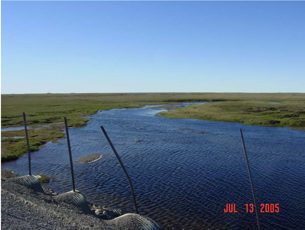
Photograph 140. Gravel outwash and deep scour downstream of the western portion of the Spine Road crossing of the Sakonowiyak River.
