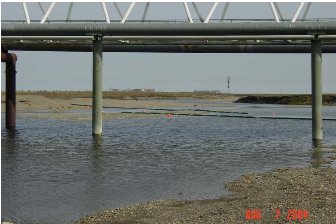
Photograph 75. Extensive gravel outwash and actively eroding tundra banks in the Putuligayuk River downstream of the Spine Road crossing and pipeline bridge.
