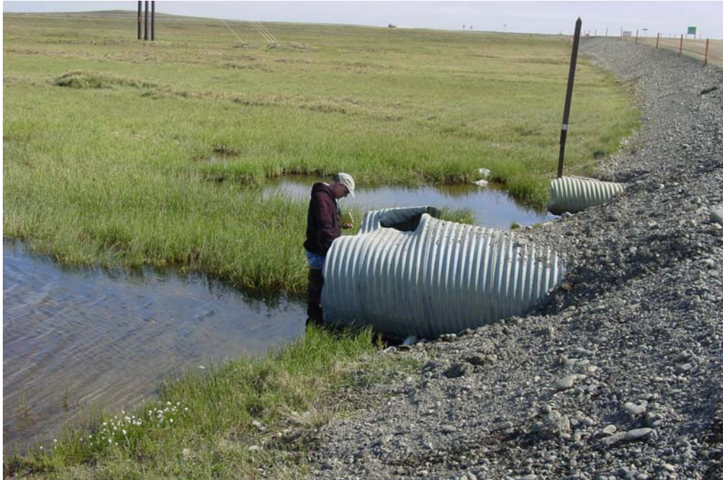
Photograph 238. Damaged outlet of the East Fork Central Creek 48 inch culvert, July 8, 2007.
