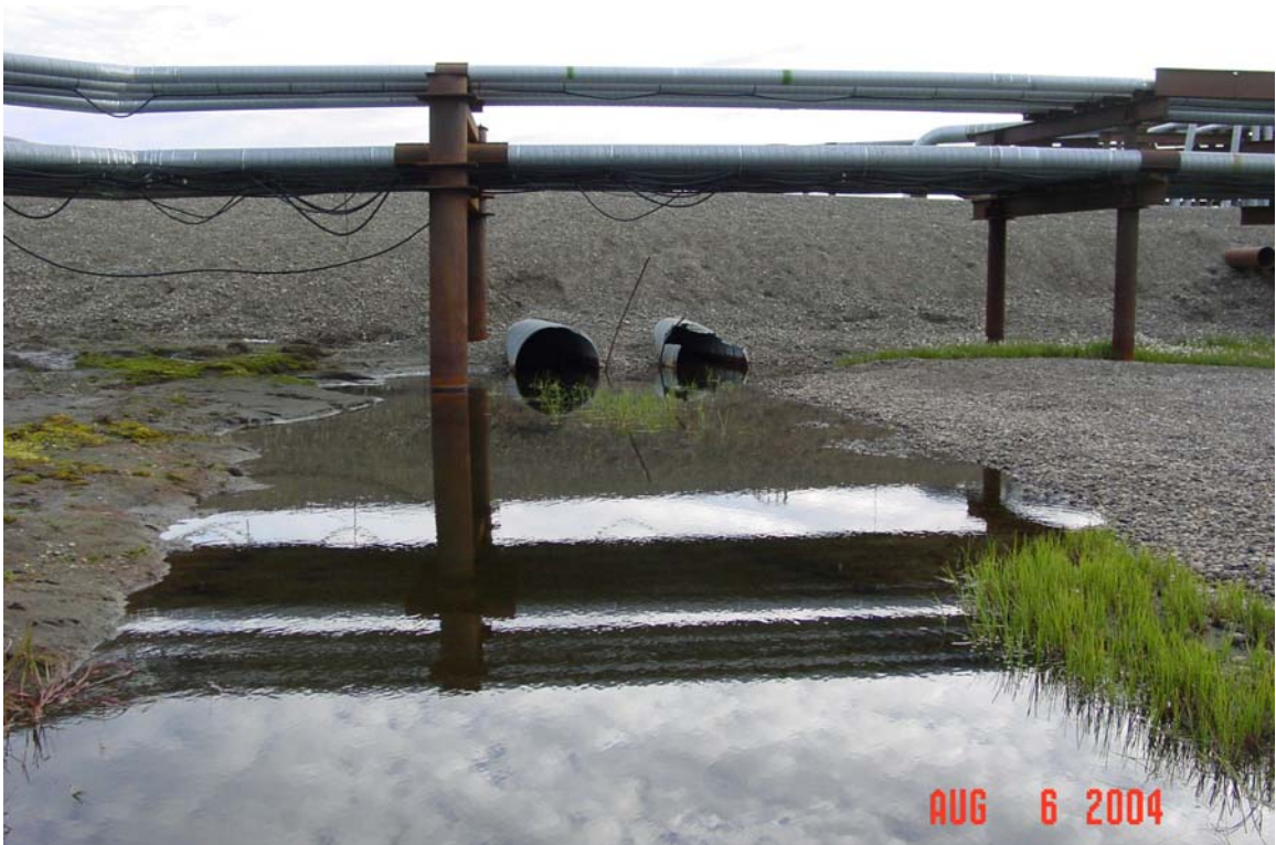
Photograph 134. Leach Creek damaged culvert outlets and outwash gravel.
