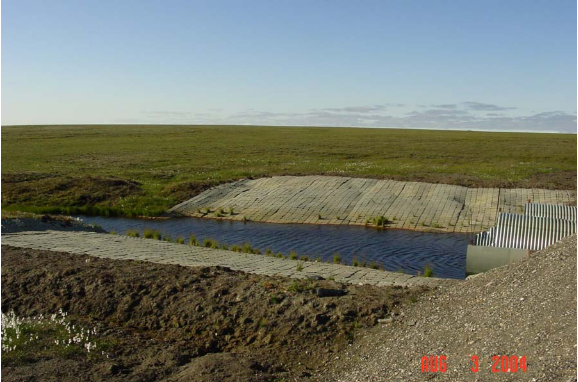
Photograph 408. Kachemach River tributary culvert outlets with extensive gobi mat erosion protection.
