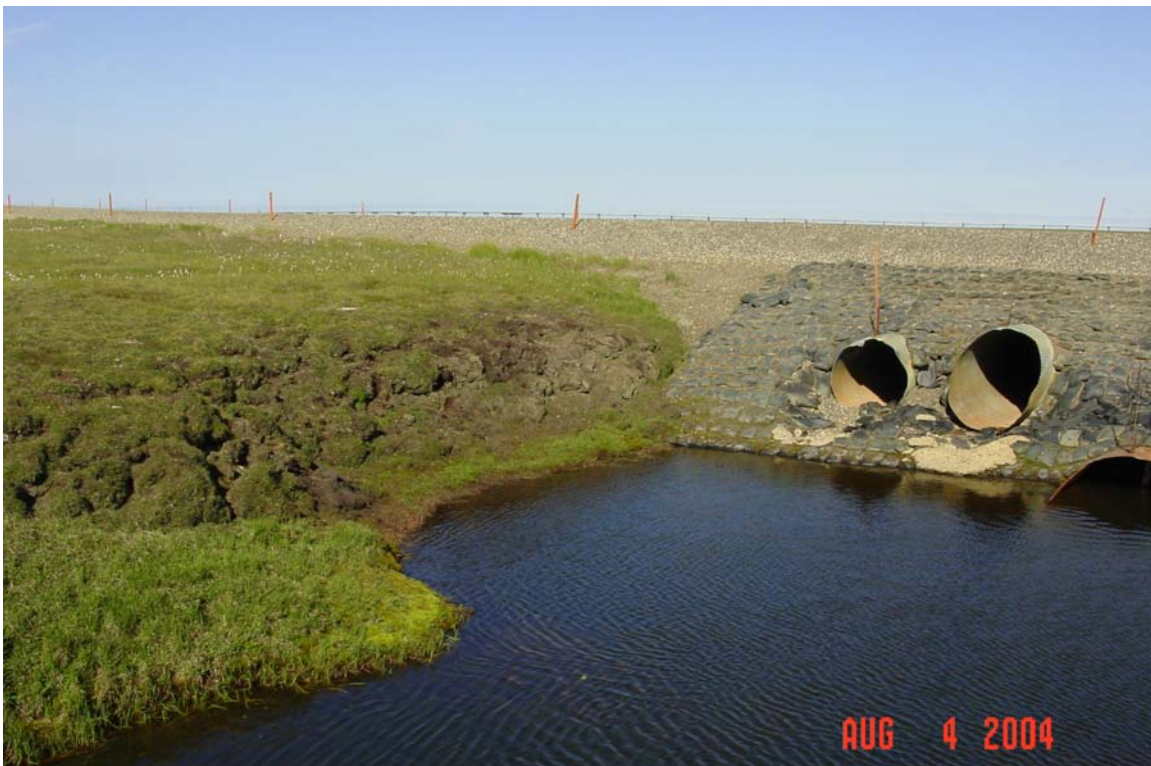
Photograph 308. Tundra erosion along the western margin of the Kalubik Creek tributary (Nowhere Creek) culvert battery inlet.
