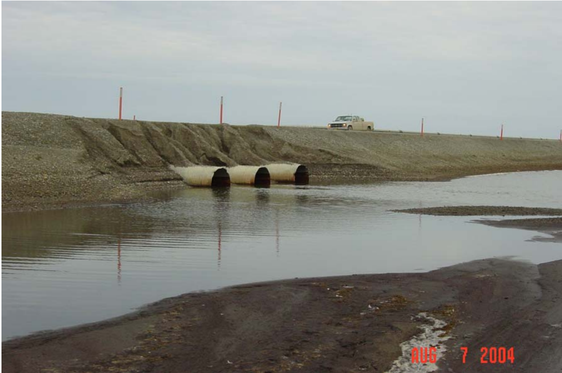
Photograph 57. LGI Estuary Creek culvert outlets, with significant gravel outwash and road prism erosion.
