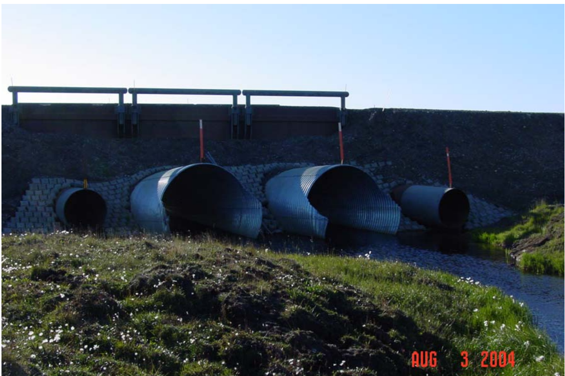
Photograph 407. Kachemach River tributary culvert battery inlets.
