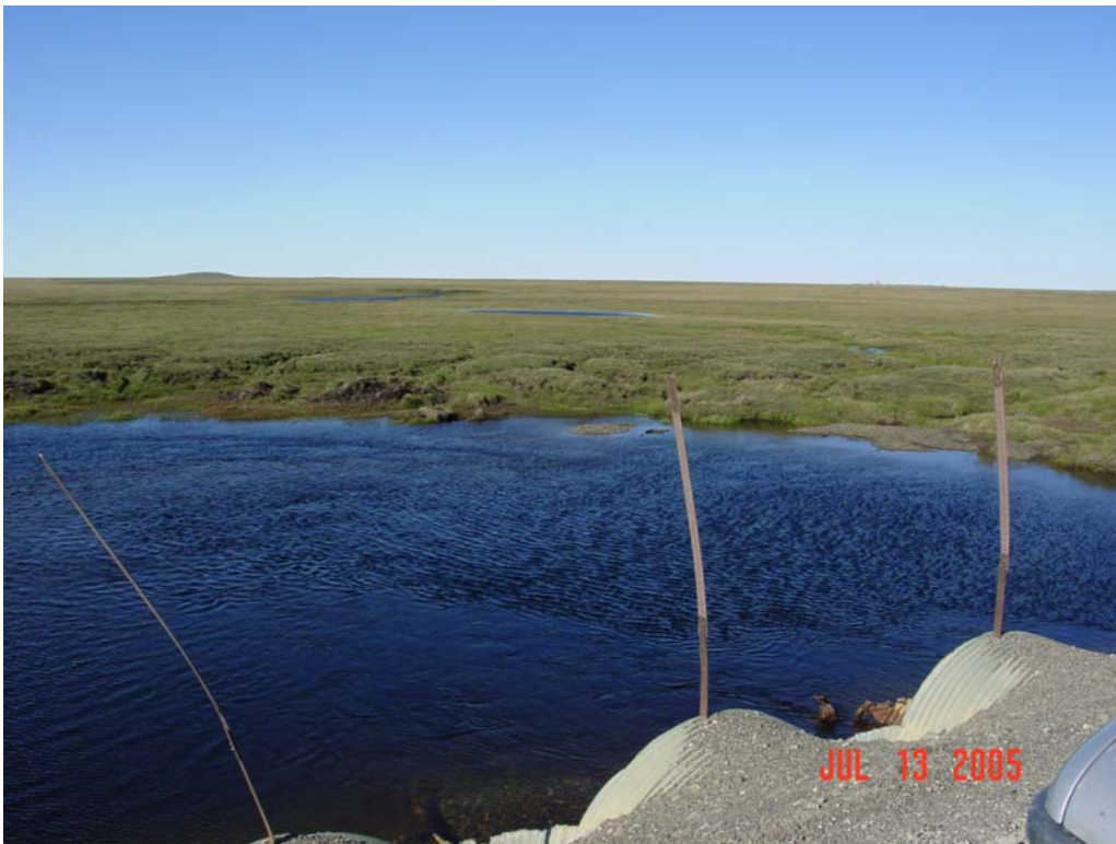
Photograph 139. Deep scour pool and gravel outwash at the eastern portion of the Spine Road crossing of the Sakonowyak River.
