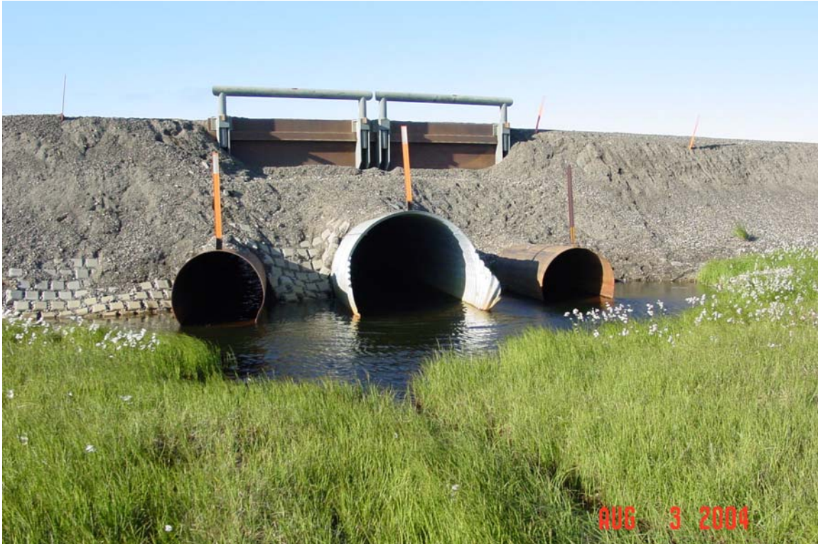
Photograph 403. Culvert inlets at the Miluveach River tributary. Note the bridge decking over the partially collapsed culvert.
