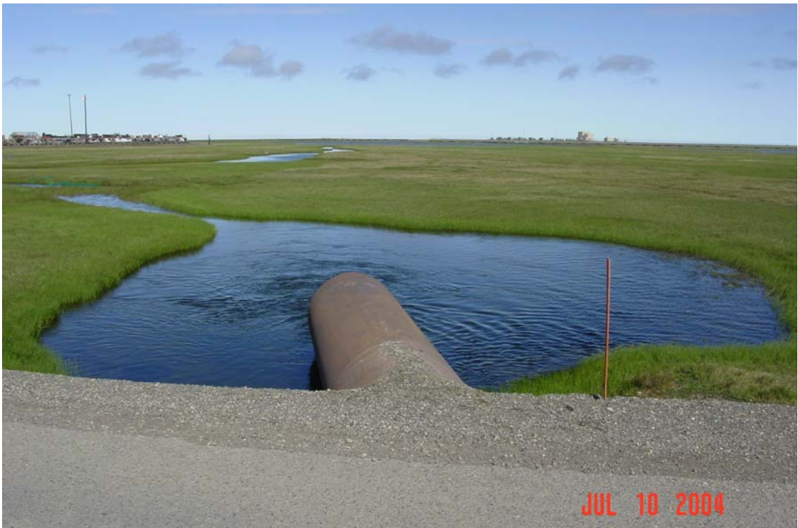
Photograph 123. Fawn Creek downstream of the Spine Road crossing and its large scour pool.
