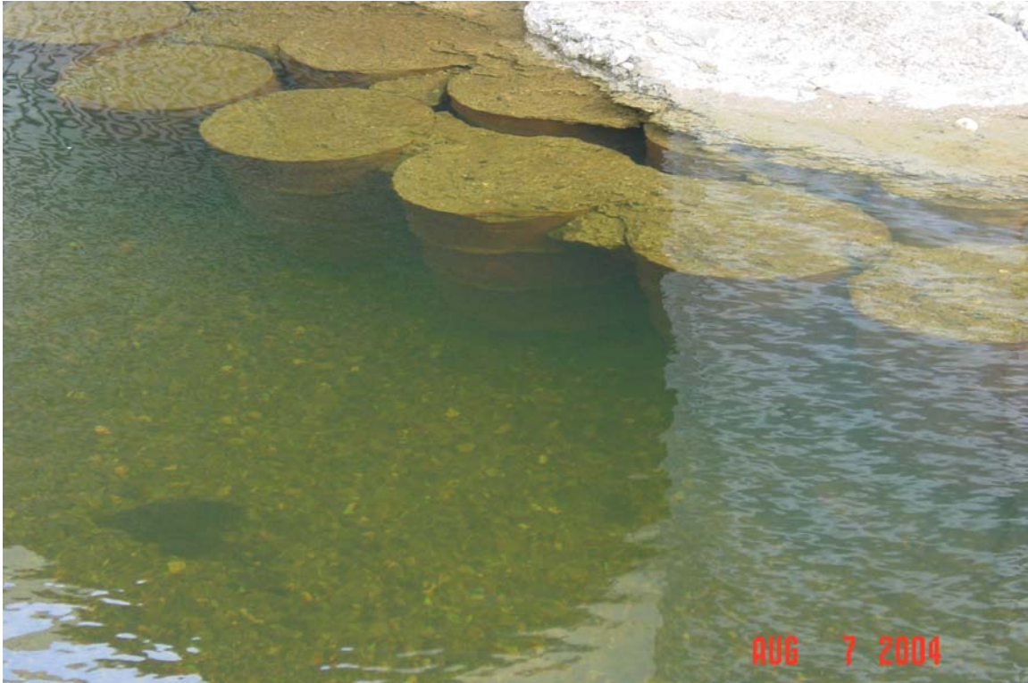
Photograph 72. Concrete-filled barrel armor has been undercut by scour at the inlets to the Putuligayuk River Spine Road culverts.
