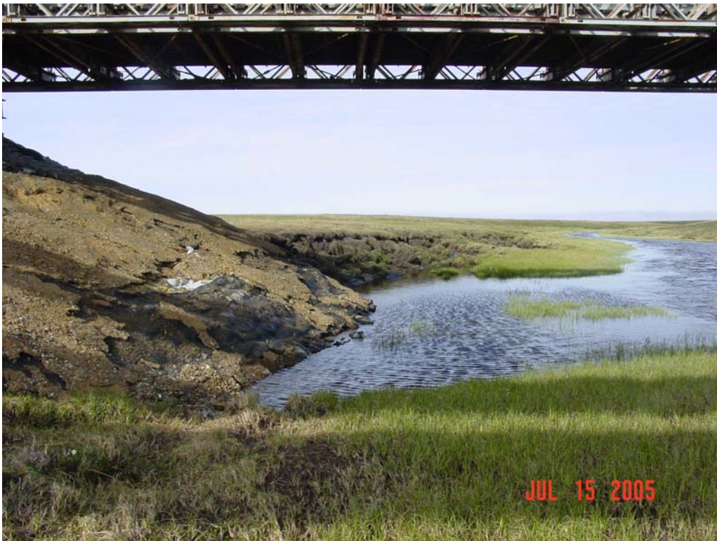
Photograph 156. West abutment erosion, sand bag disturbance and tundra erosion.
