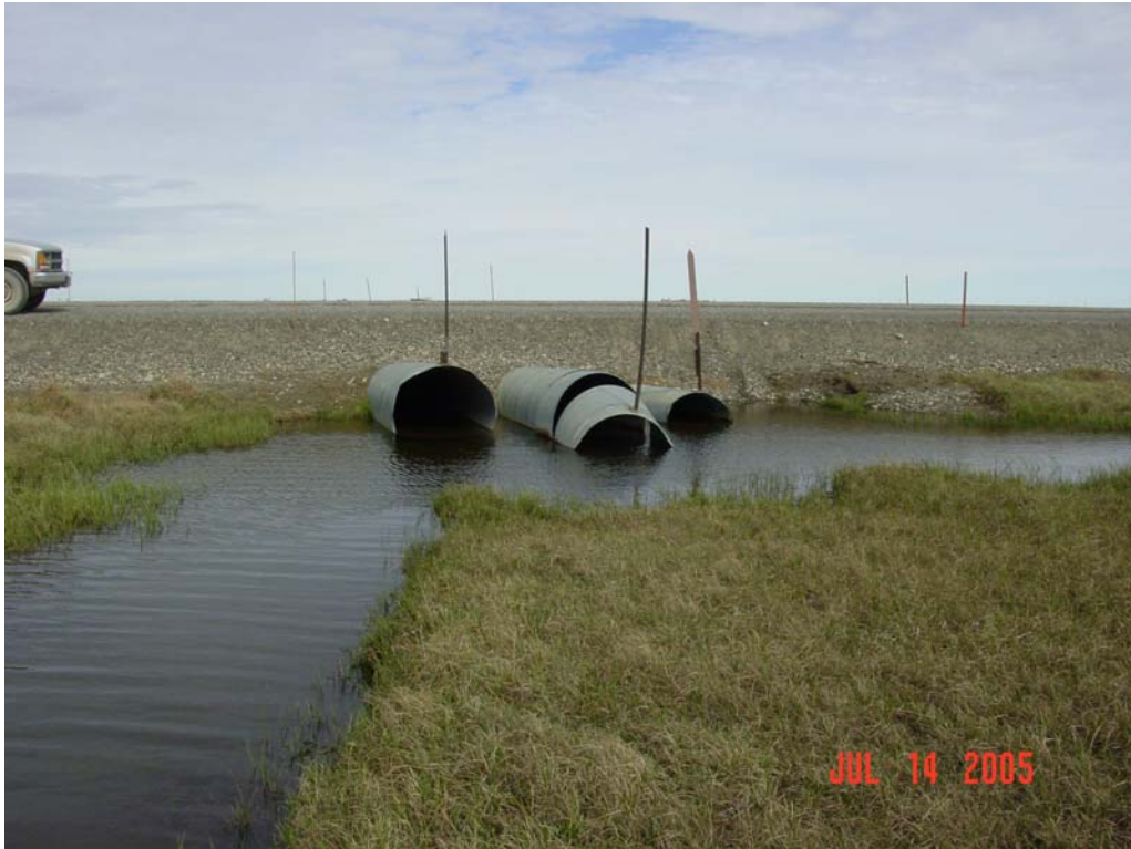
Photograph 335. Ugnuravik River tributary culvert outlets.
