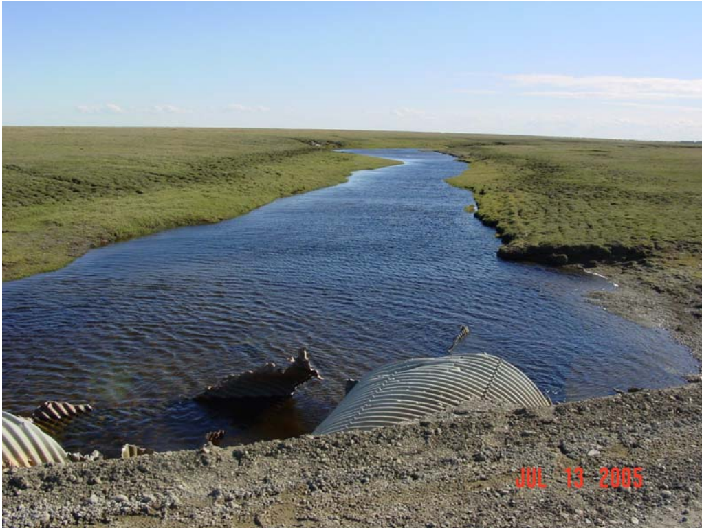
Photograph 144. Damaged culvert inlets at the Smith Creek crossing of the Spine Road.
