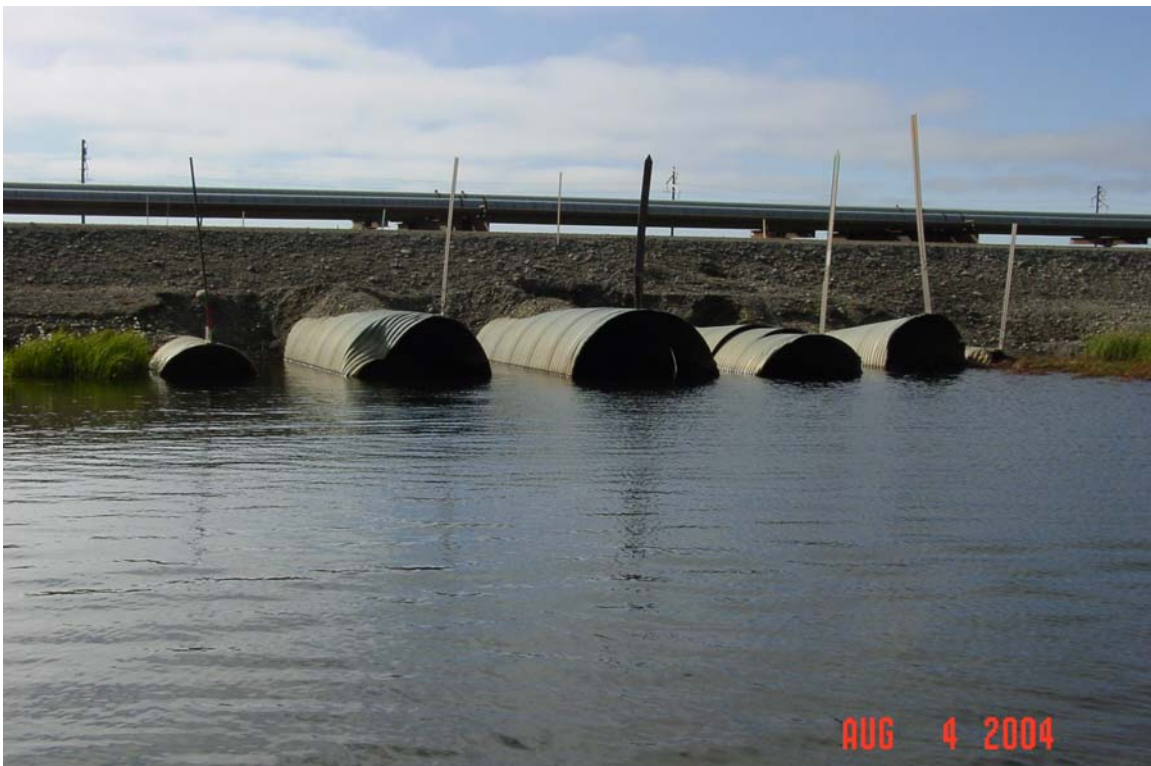
Photograph 359. West Fork Ugnuravik River culvert outlets. Note the damaged outlets, the split culvert and the bowed culvert.
