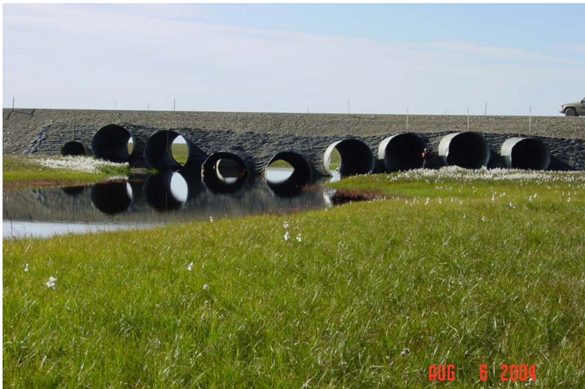
Photograph 265. Ugnuravik River culvert outlets.
