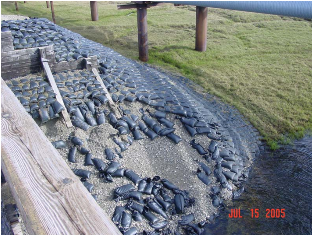
Photograph 166. Eroded sandbag armor on the east abutment.
