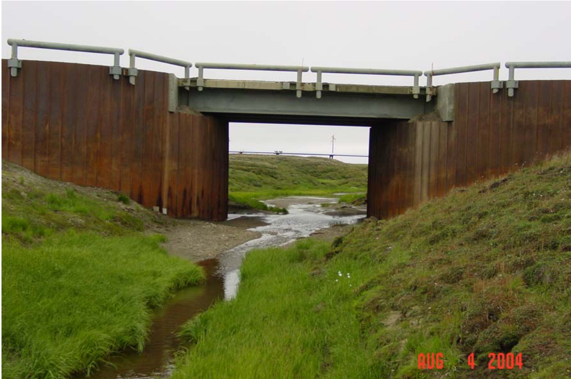
Photograph 395. The Trouble Creek bridge viewed from downstream. Note the bridge does not span bankfull flows.
