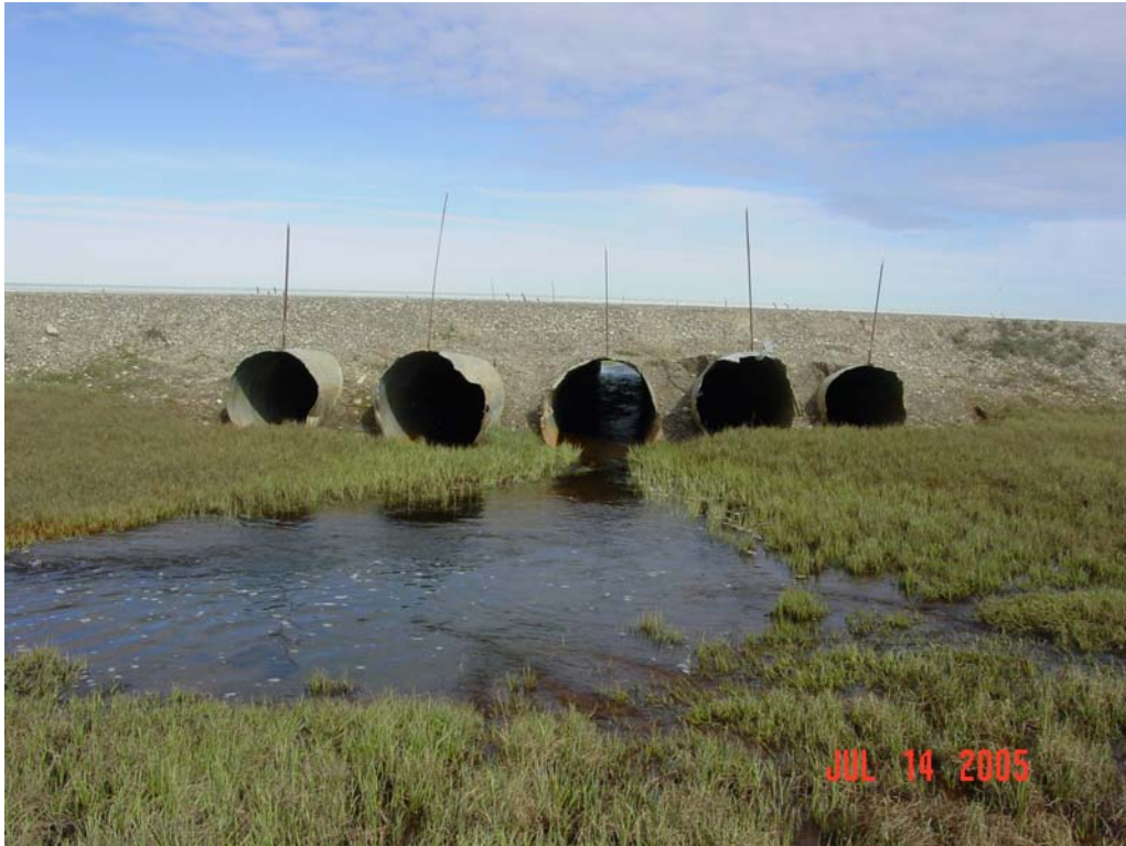
Photograph 367. Kalubik Creek tributary culvert inlets.
