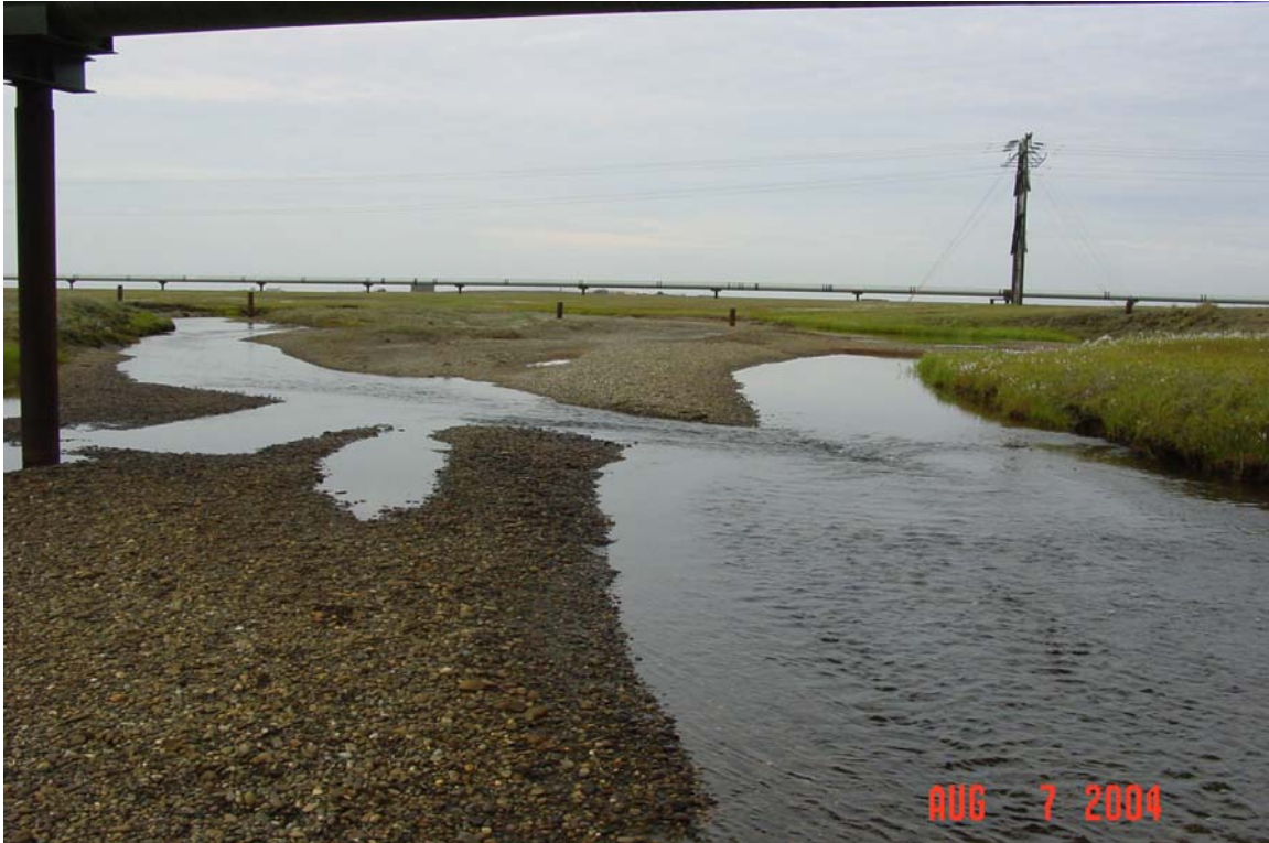
Photograph 86. Little Putuligayuk River old low water crossing area, looking immediately upstream. Gravel accretion and split channel can be seen.
