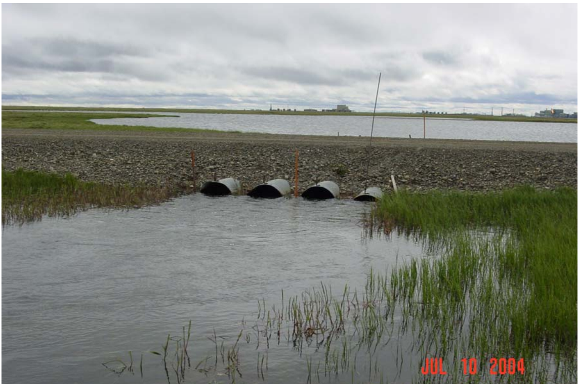
Photograph 121. Fawn Creek culvert outlets. Note the difference in water surface elevation between the upstream and downstream sides of the road.
