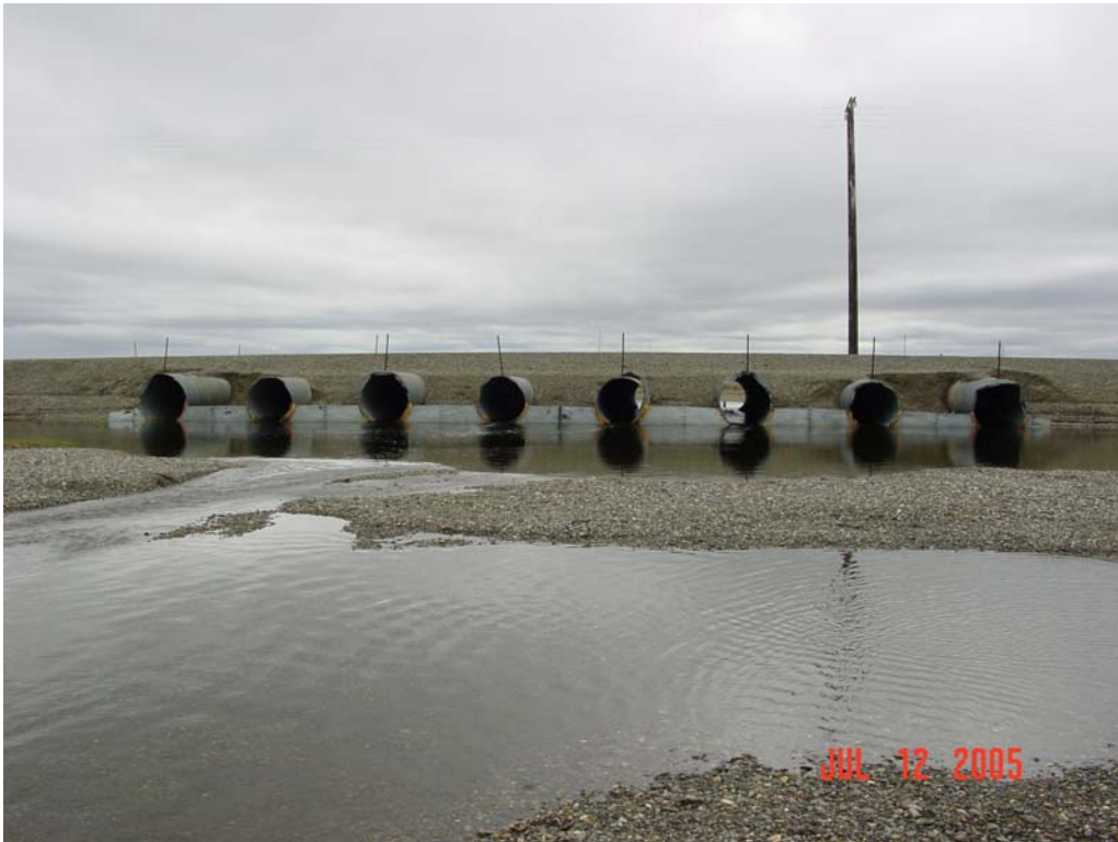
Photograph 32. Washout Creek culvert outlets. Damage to all outlets can be observed along with significant gravel outwash and road prism erosion.
