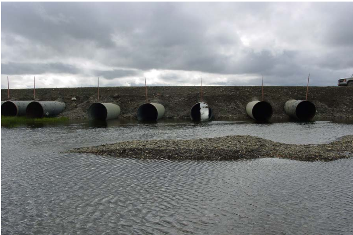
Photograph 232. East Fork West Fork Central Creek culvert outlets and outwash gravels, August 8, 2006.
