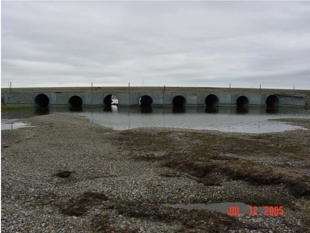
Photograph 31. Washout Creek culvert inlets.
