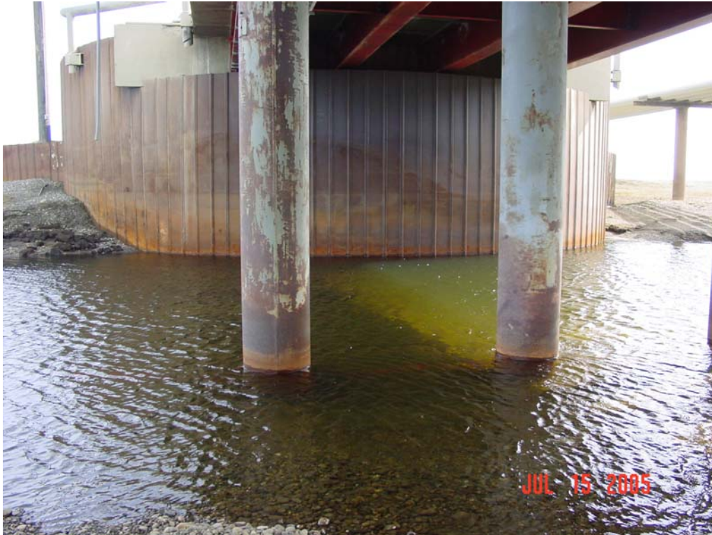
Photograph 203. Abutment encroaching in the stream channel.
