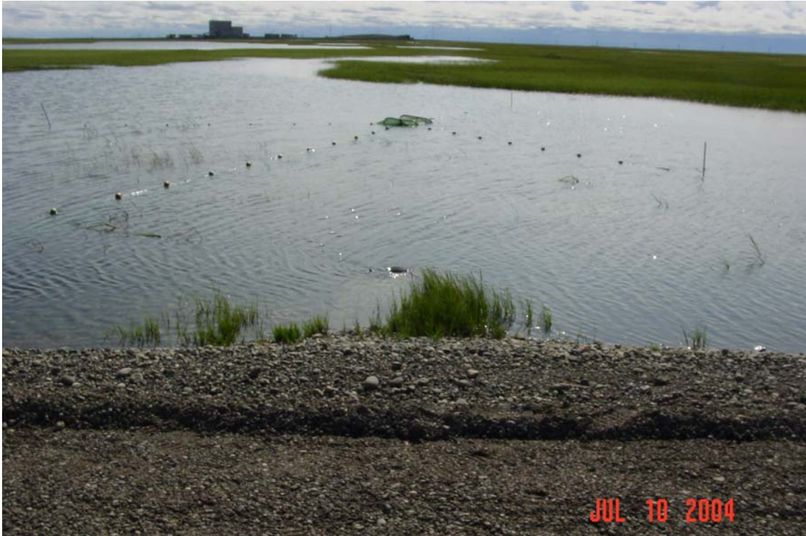
Photograph 106. Fawn Creek upstream of the GC1 to GC2 Road. Water is ponded above the crossing; culvert is submerged in the foreground.
