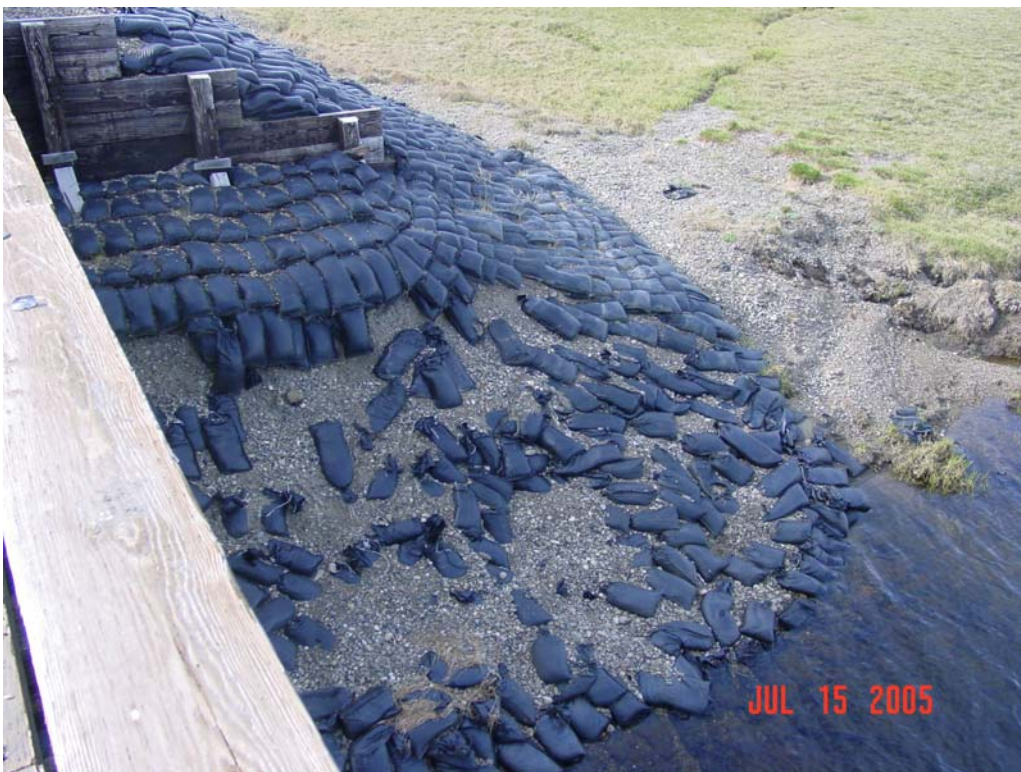
Photograph 168. Sand bag armor erosion on the west abutment of the Pebble Creek bridge.
