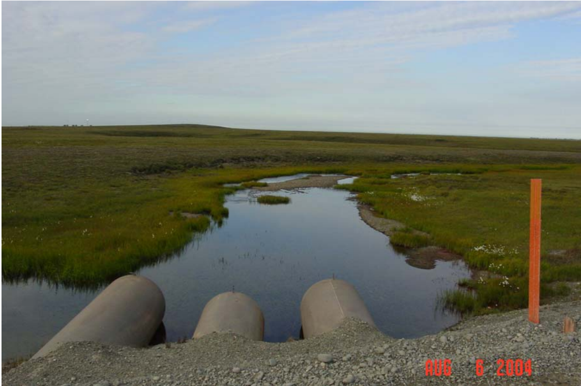
Photograph 127. Leach Creek downstream of the Spine Road crossing. Significant gravel outwash is present in the stream channel.
