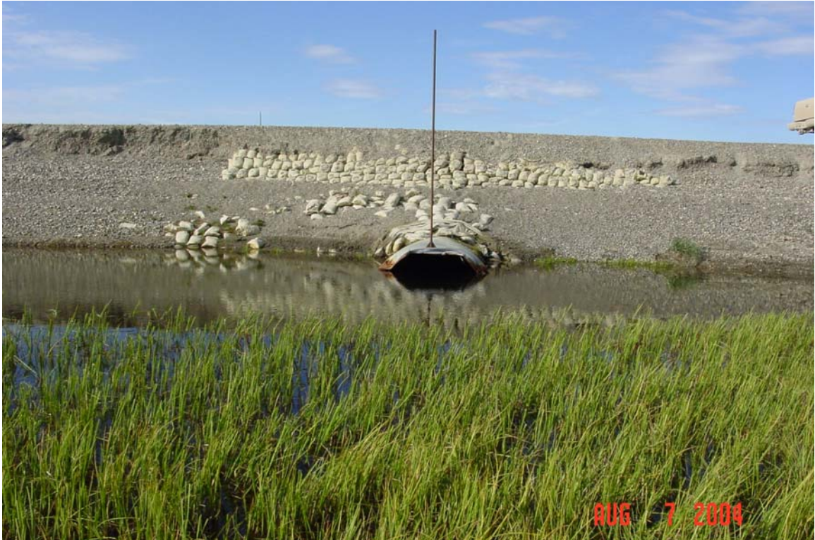
Photograph 14. South Fork Endicott Creek culvert inlet. Note the road prism erosion and high-water mark above culvert.
