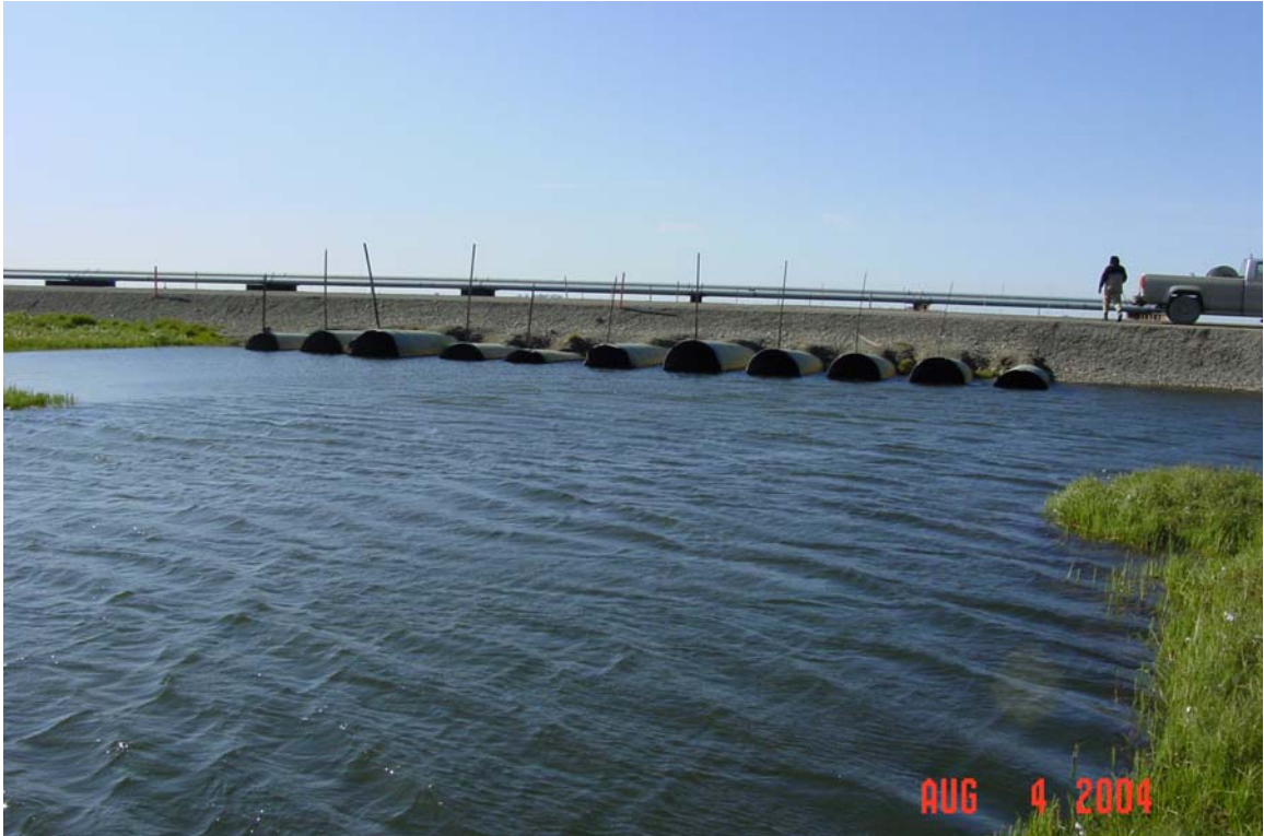
Photograph 288. West Fork Ugnuravik River tributary culvert outlets.
