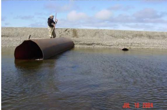
**FC3 Crossing**- View of upstream side of culvert battery, crossing creating significant head resulting in whirlpool effect as water drops into culverts inlets.
