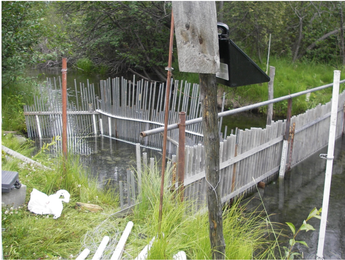
Figure 4. Long Lake weir and sampling box under construction, 2008.
