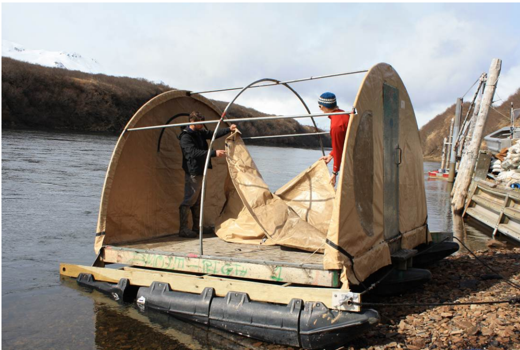
Figure 13. The photo illustrates the platform, pontoon frame, harness/anchor line attachment, and weatherport construction.
