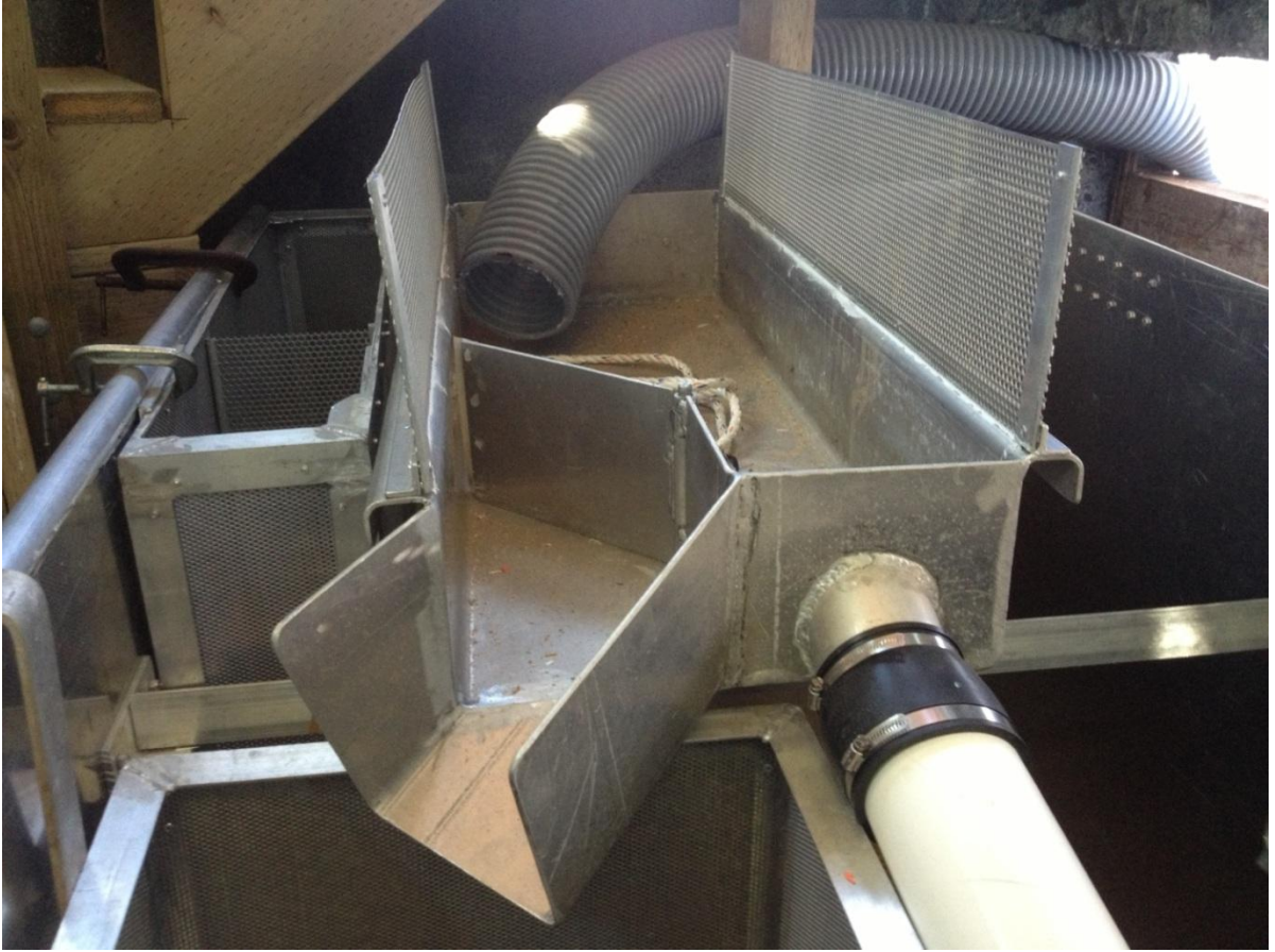
Figure 8.–Flex pipe position entering the smolt shack.
