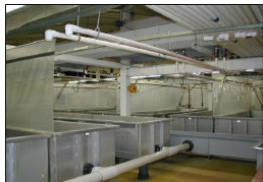
Main Bay Hatchery interior
