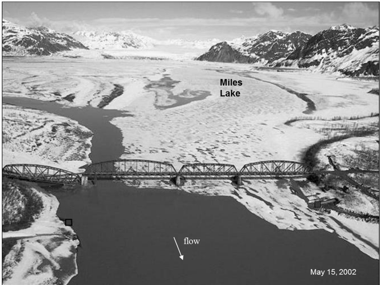
Figure 2.—The Copper River at mile 48 of the Copper River Highway showing the Million Dollar Bridge.
