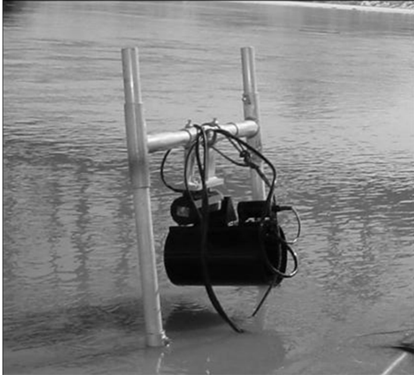
Figure 4.—A DIDSON positioned horizontally for estimating salmon passage, encased in an aluminum cylinder, attached to a single-axis, automated rotator mounted to an aluminum H-mount, with an attached tilt and roll sensor along the Copper River’s south bank, Miles Lake sonar.
