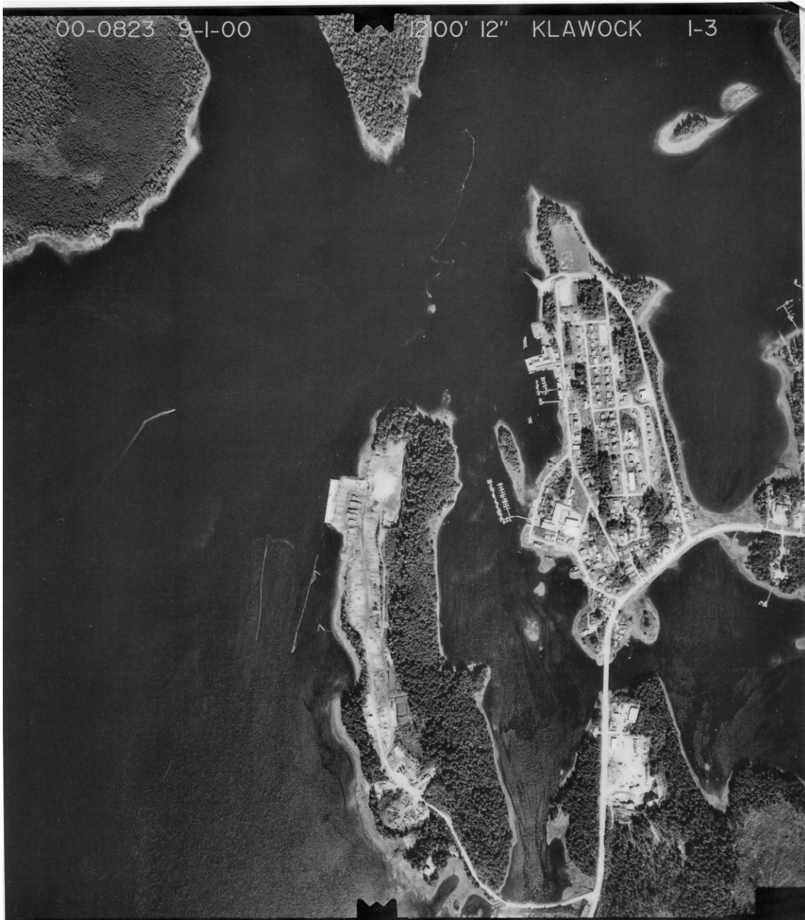
Figure D- 2. Aerial Photograph of Klawock Inlet
