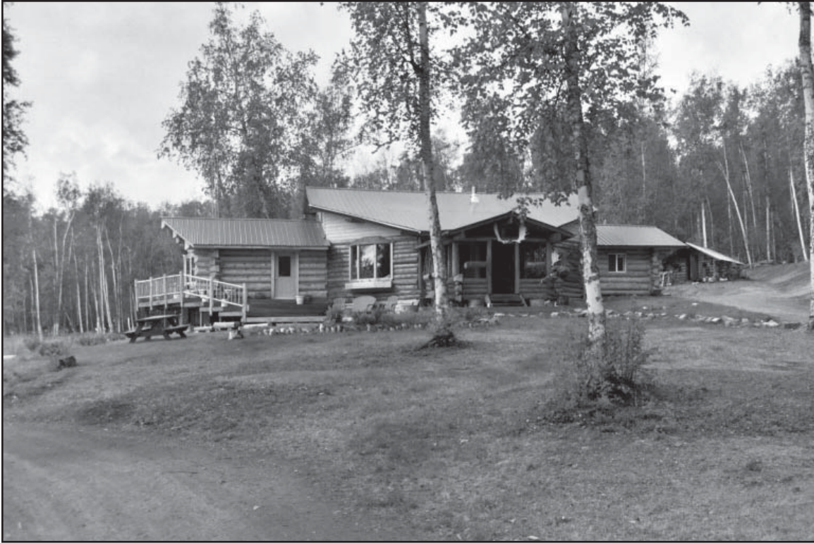
Plate 3-1 Denali West Lodge, Lake Minchumina Alaska
