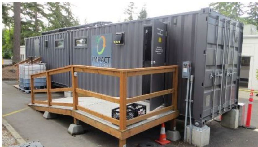
Figure 3.2. Impact Bioenergy modular anaerobic digestion system.
