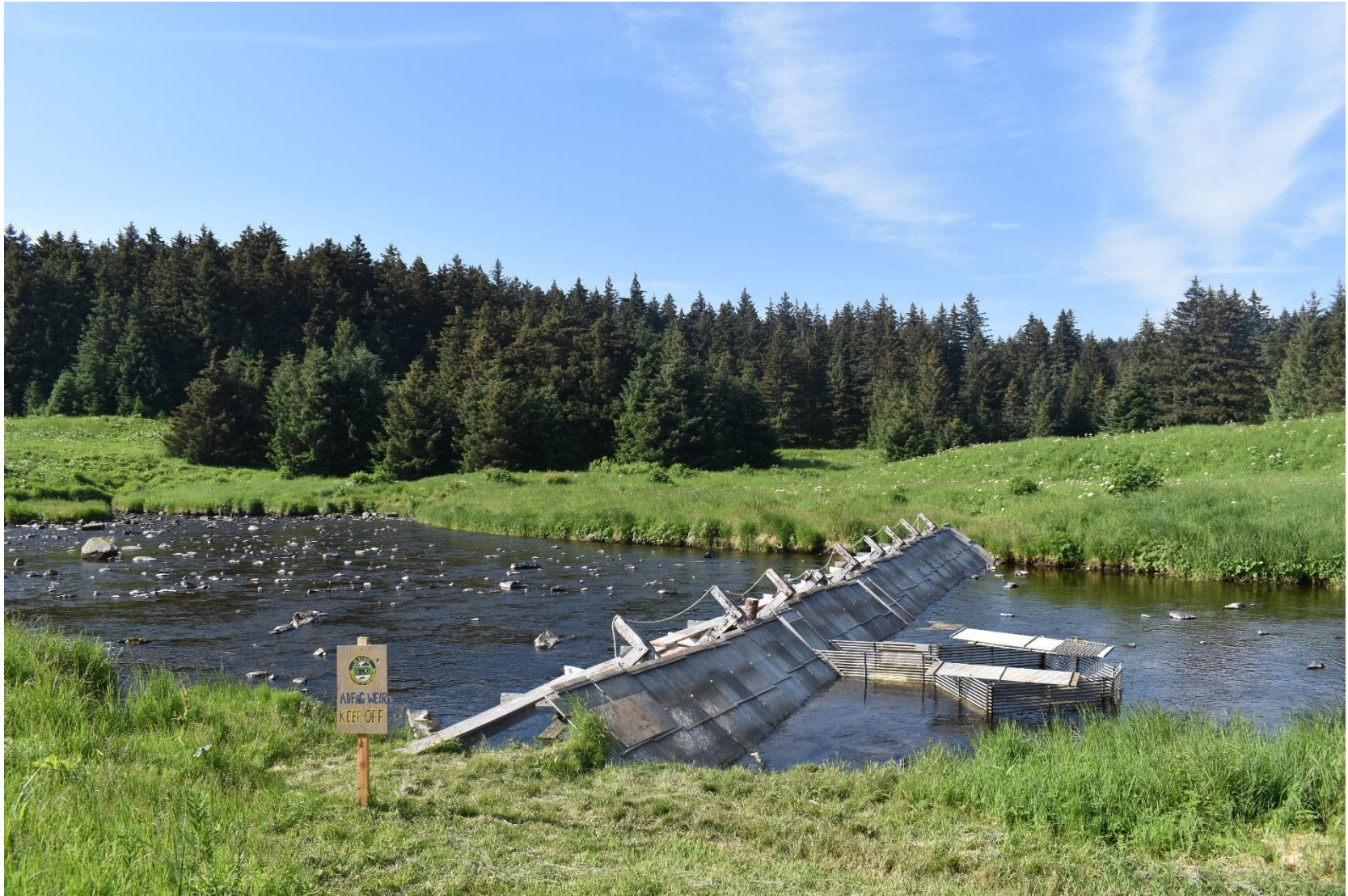
Figure 3.–View of the adult salmon enumeration weir and “Scott” trap in Afognak River, 2019.
