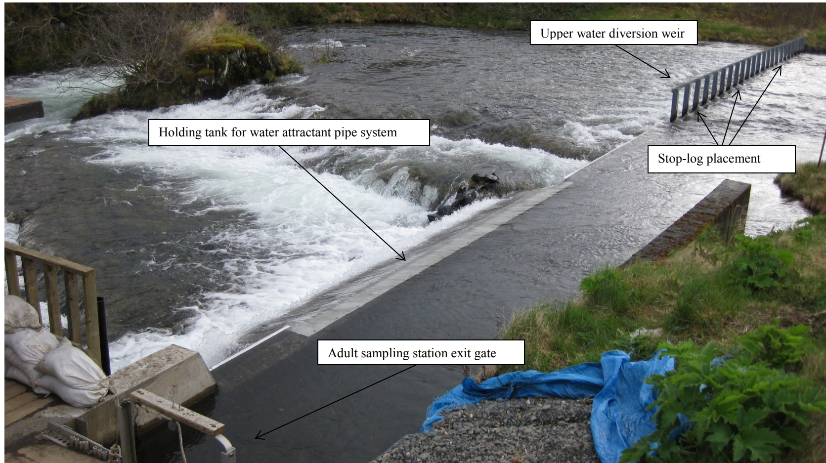
Figure 6.—Frazer fish pass upper water diversion weir and holding tank for water attractant pipe system.
