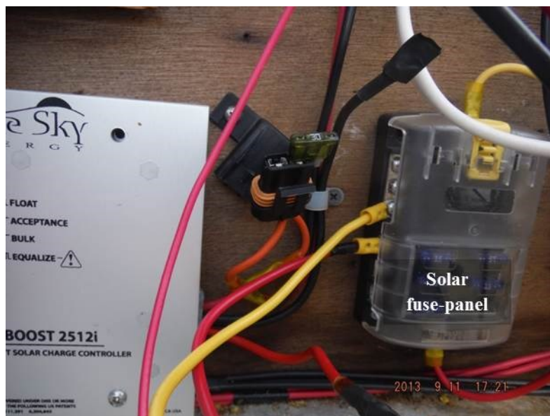
Figure 7. Photo of the solar fuse panel where positive and negative leads from the solar panels terminate.
