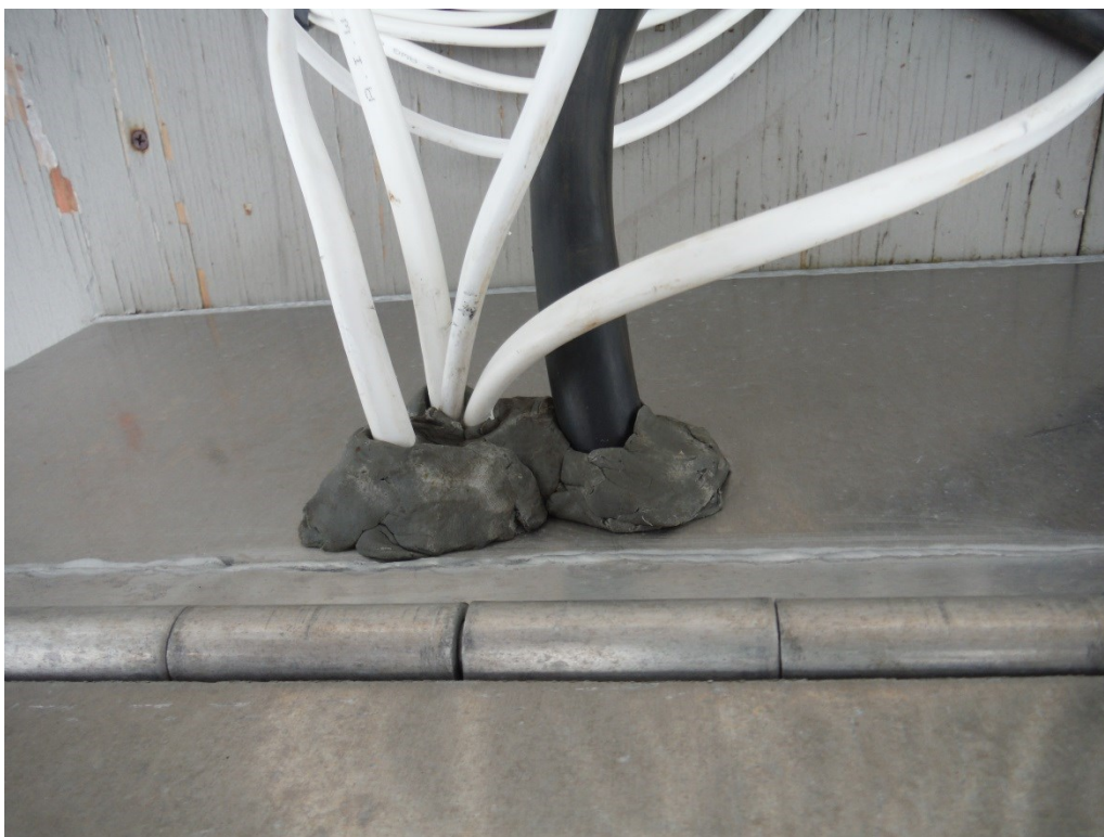
Figure 20. Use plumbers putty to waterproof the holes in the strongbox through which coax and electrical wires are routed.
