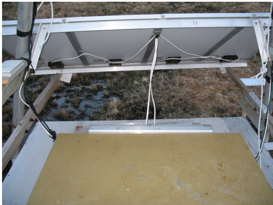
Figure 23. Illustrates the aluminum brackets used to attach the solar panel array to the Quad at Chenik Lake.
