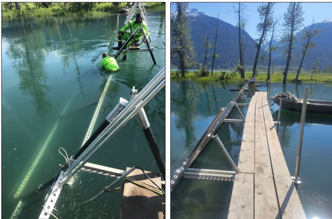
Figure 5.—The installation of the gate frame by weir crew (left), and the view of the weir board walk with pickets installed (right). (© 2022 ADF&G. Photos by Shelby M. Flemming.)
