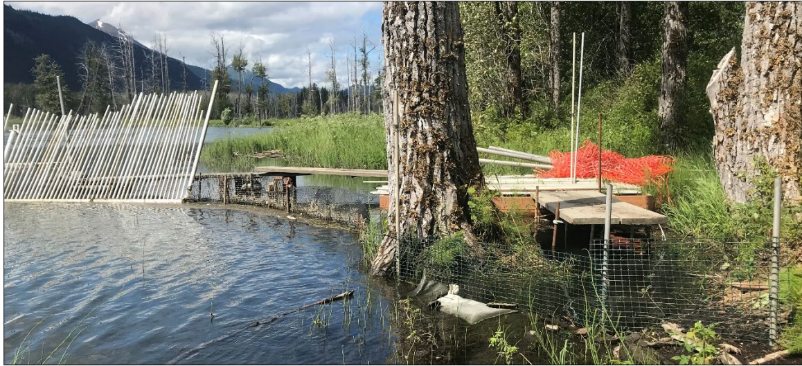
Figure 6.—Fencing and sandbags installed river right of weir to ensure no fish passage during high water events. (© 2022 ADF&G. Photo by Shelby M. Flemming.)
