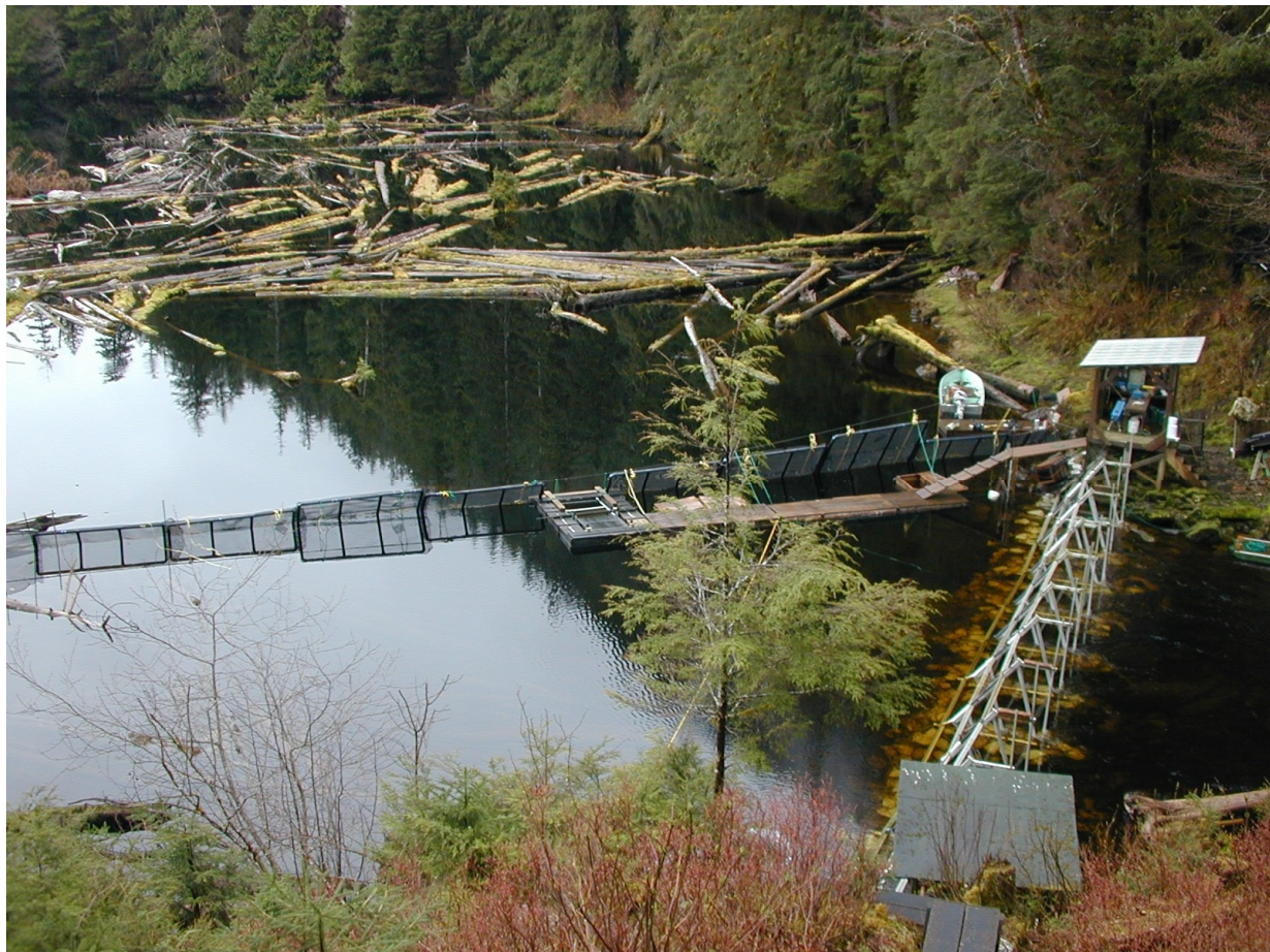
Figure 3.—The outlet of Hugh Smith Lake showing the smolt weir and the adult weir support structure.
