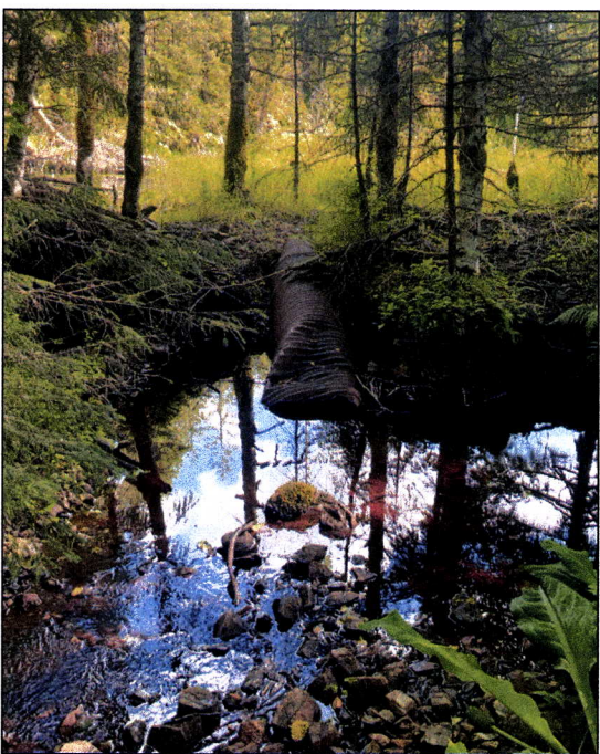
Figure 3. Damaged pipe at waypoint 492.
