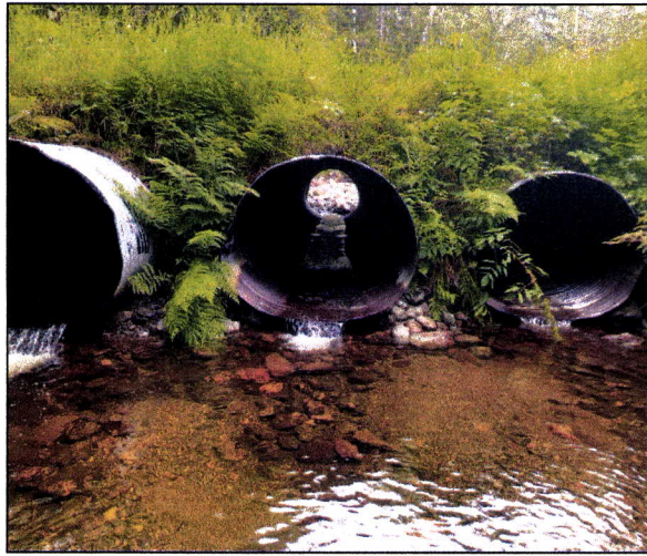
Figure 2.—Outlets of the triple culvert bank waypoint 436.
