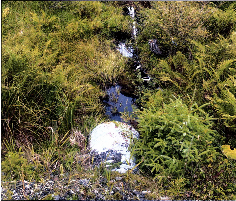
Figure 2.—Stream channel and culvert at waypoint 715.
