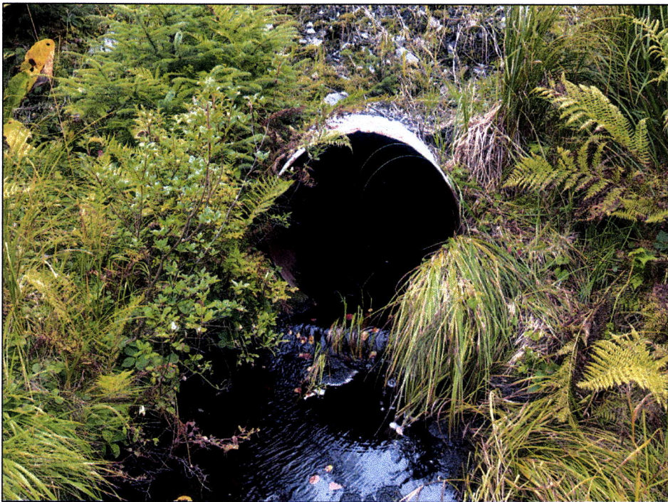
Figure 3.—Culvert at waypoint 715.
