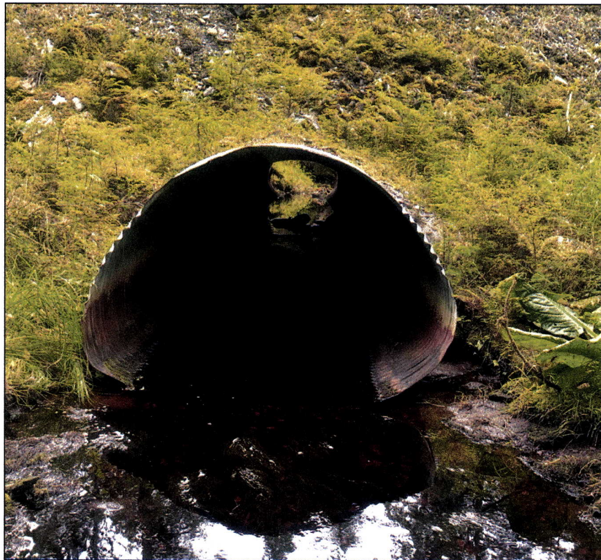
Figure 3.—Culvert at waypoint 714.
