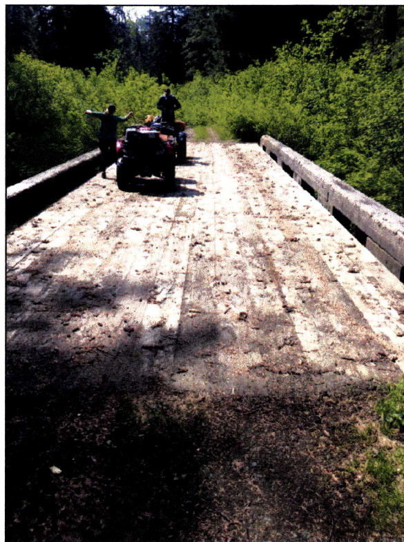
Figure 3.—Bridge surface at waypoint 444.
