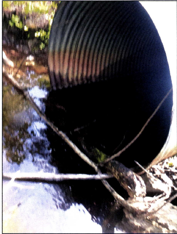
Figure 3.—Culvert outlet at waypoint 442.
