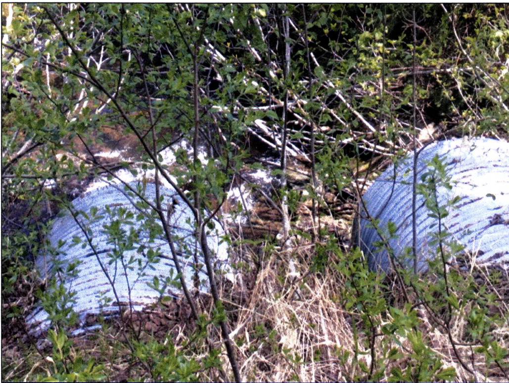
Figure 2.—Side-by-side culvert outlets at waypoint 448.
