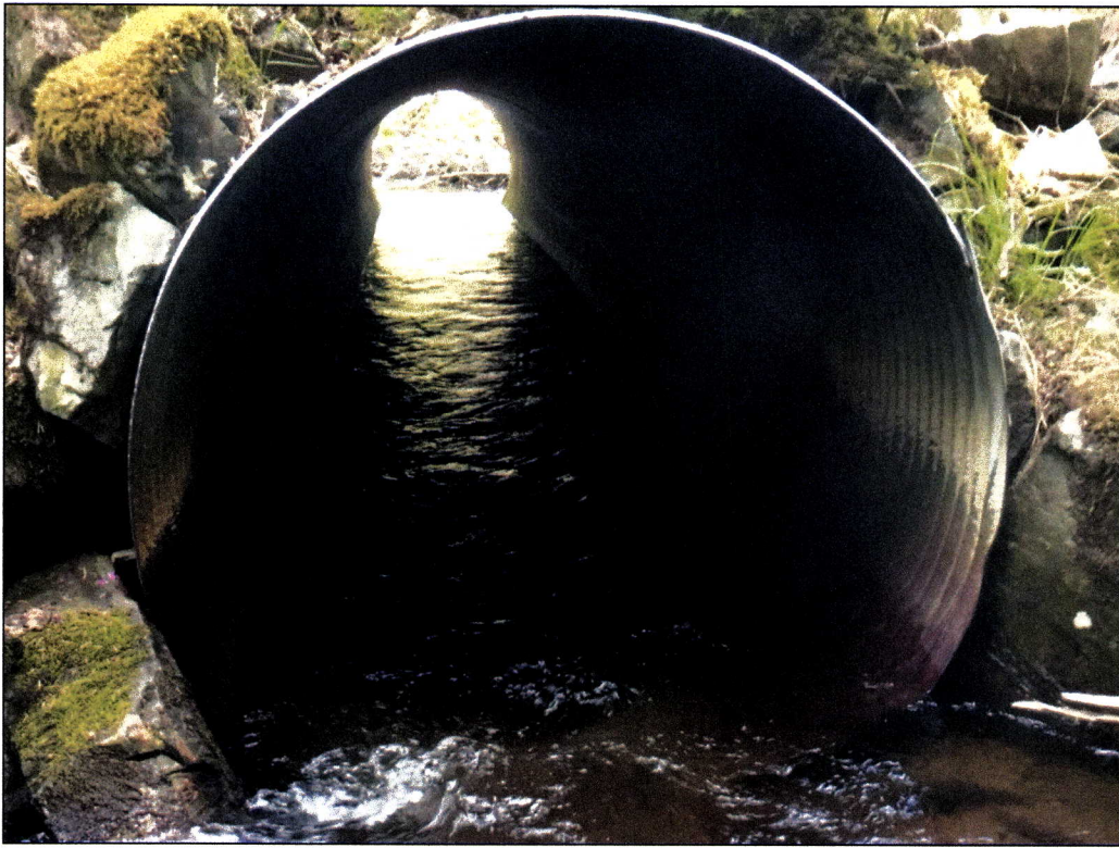
Figure 3.—Culvert outlet at waypoint 448.
