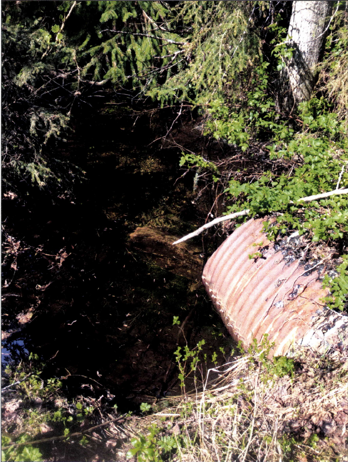
Figure 2.—Culvert inlet at waypoint 440.
