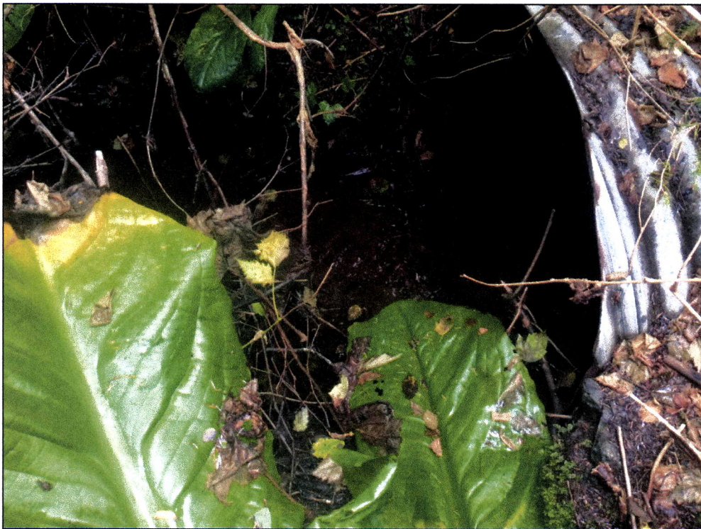
Figure 1.—Culvert outlet at waypoint 1802.
