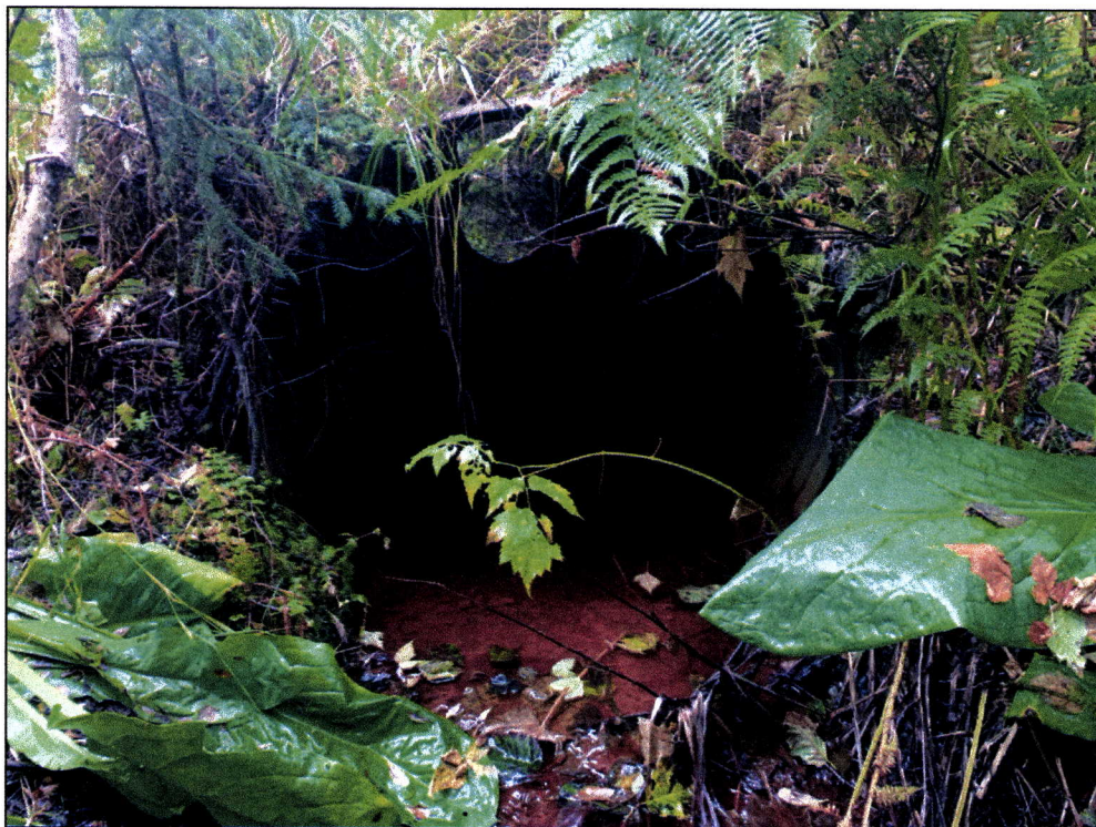
Figure 1.—Culvert outlet at waypoint 1768.
