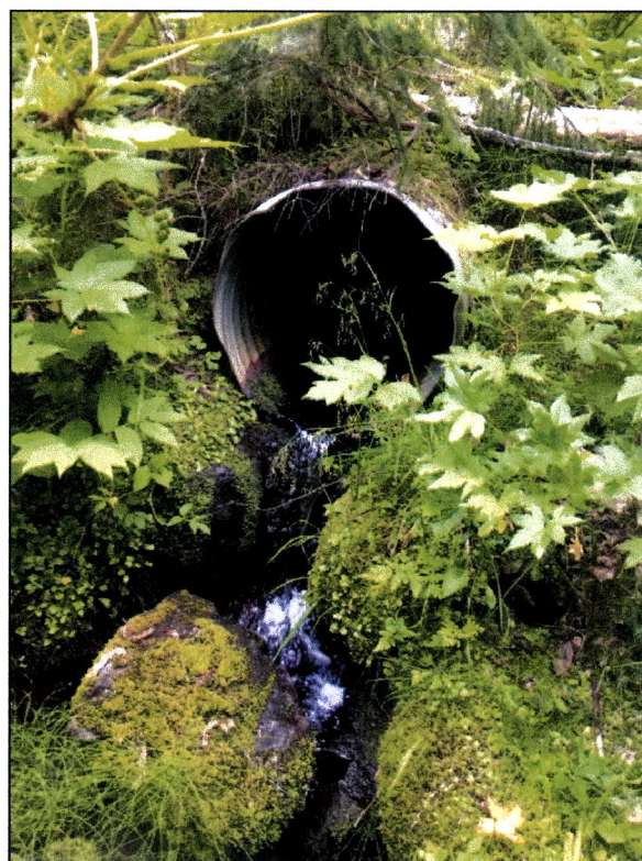
Figure 3.—Perched culvert outlet at waypoint 959.
