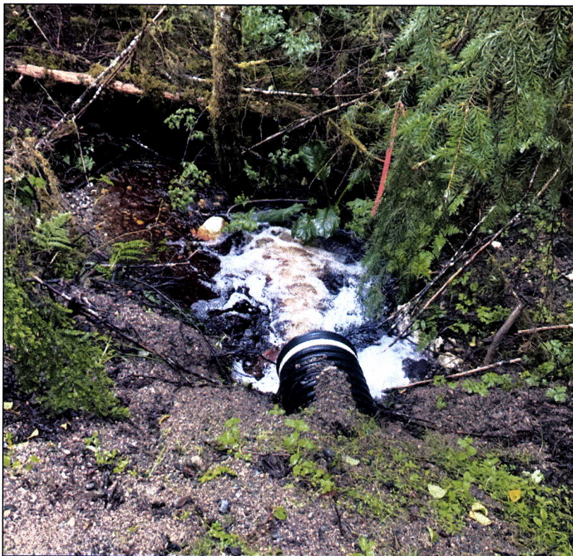
Figure 2.—Culvert and channel at waypoint 1526.
